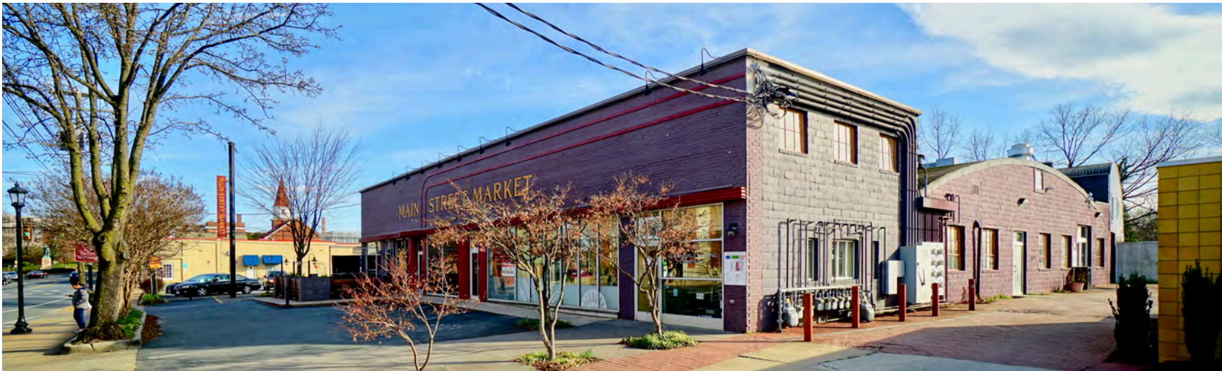
VIEW SOUTHEAST FROM WEST ENTRANCE
