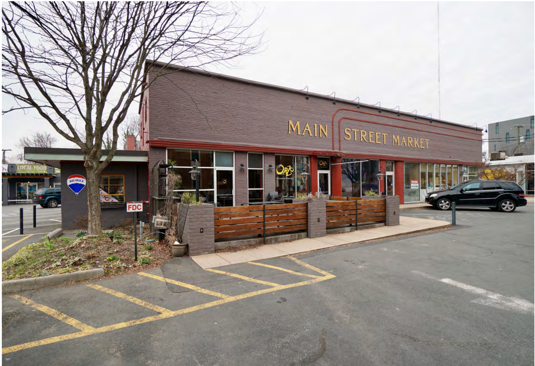
VIEW OF NORTH ELEVATION FROM EAST
