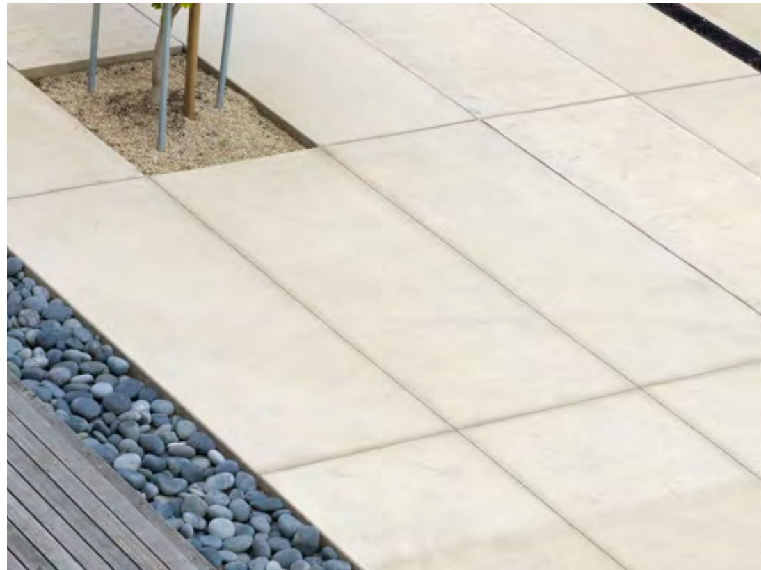
② Scored Concrete Paving
