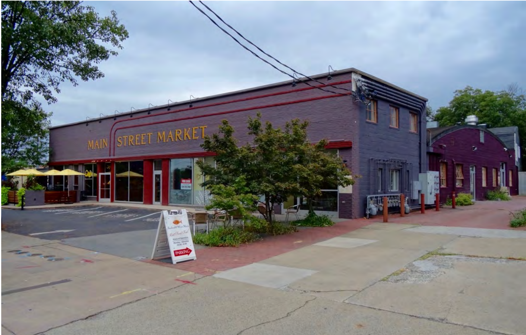
VIEW OF NORTHWEST CORNER
