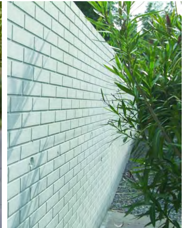
③ White Stamped Concrete Retaining Wall with Brick Coping
