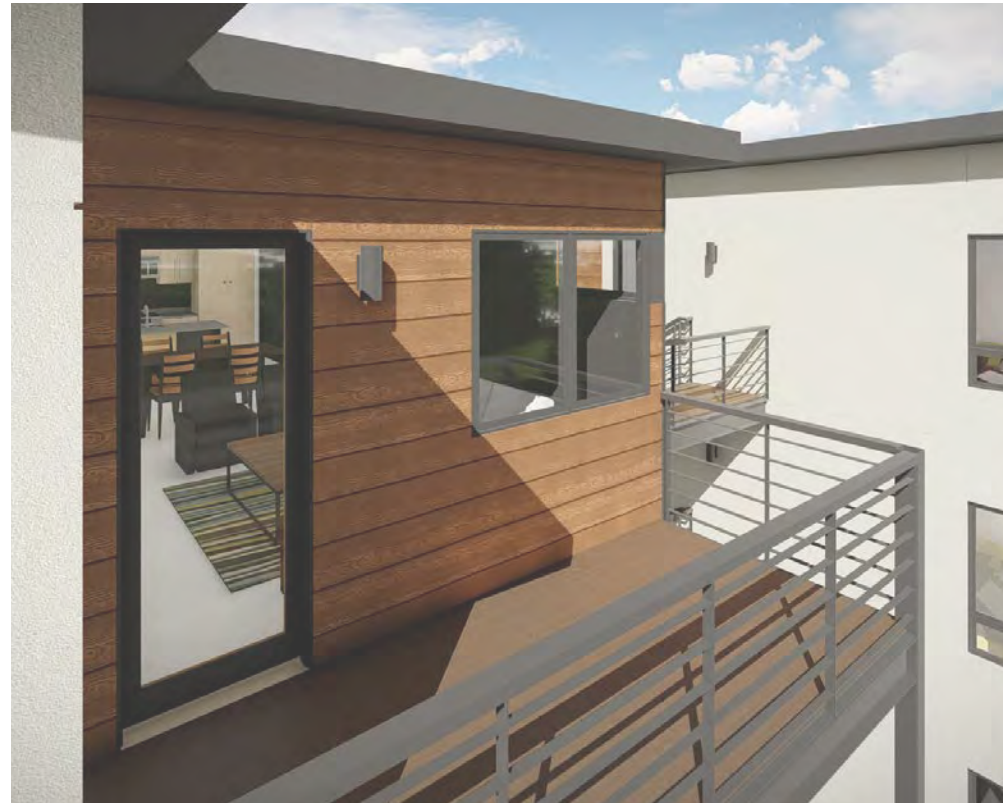
LAP SIDING AT DECK
