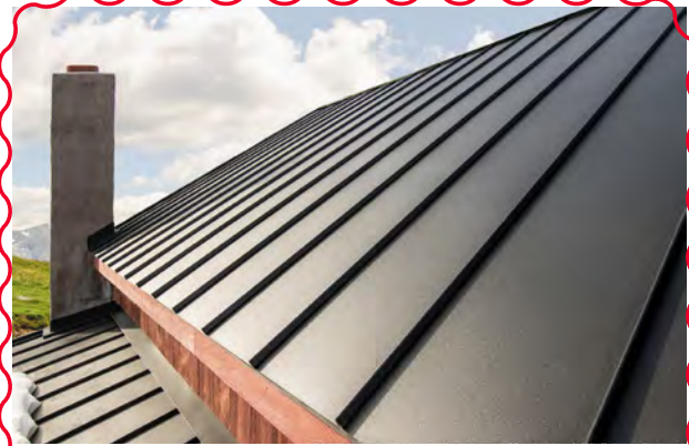
STANDING SEAM METAL ROOF
