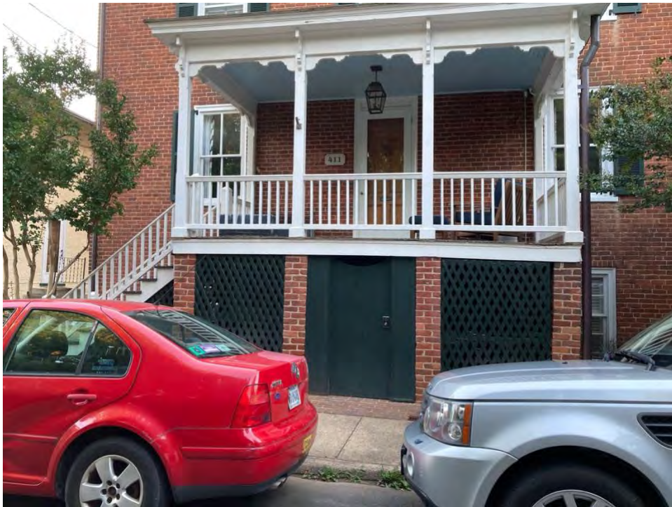
Figure 6: Focus view of entry porch and existing door below porch.
