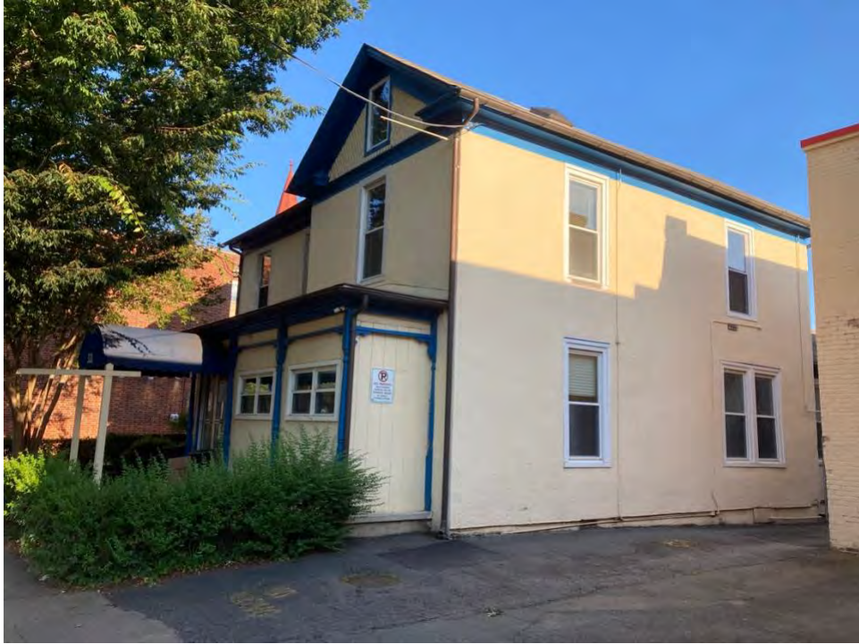
Figure 3: Oblique view of 320 West Main Street, facing southeast.
