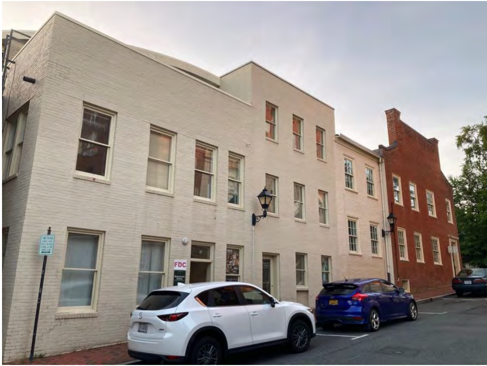
Figure 6: Oblique view of Renaissance School annex buildings along 5 th Street NE, facing northwest.
