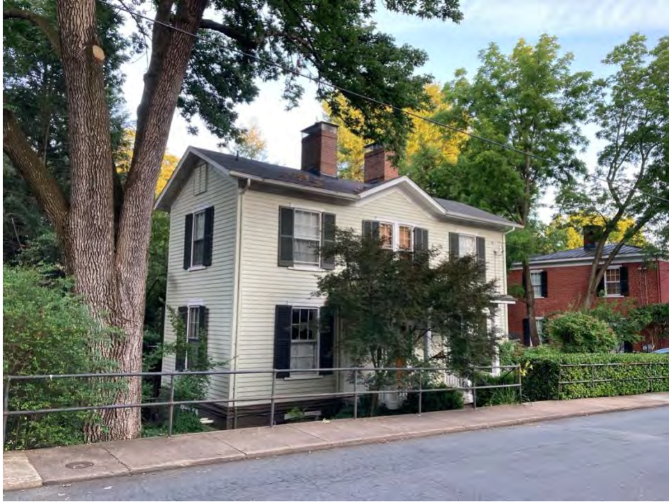
Figure 3: Oblique view of 422 North 1 st Street, facing southeast.
