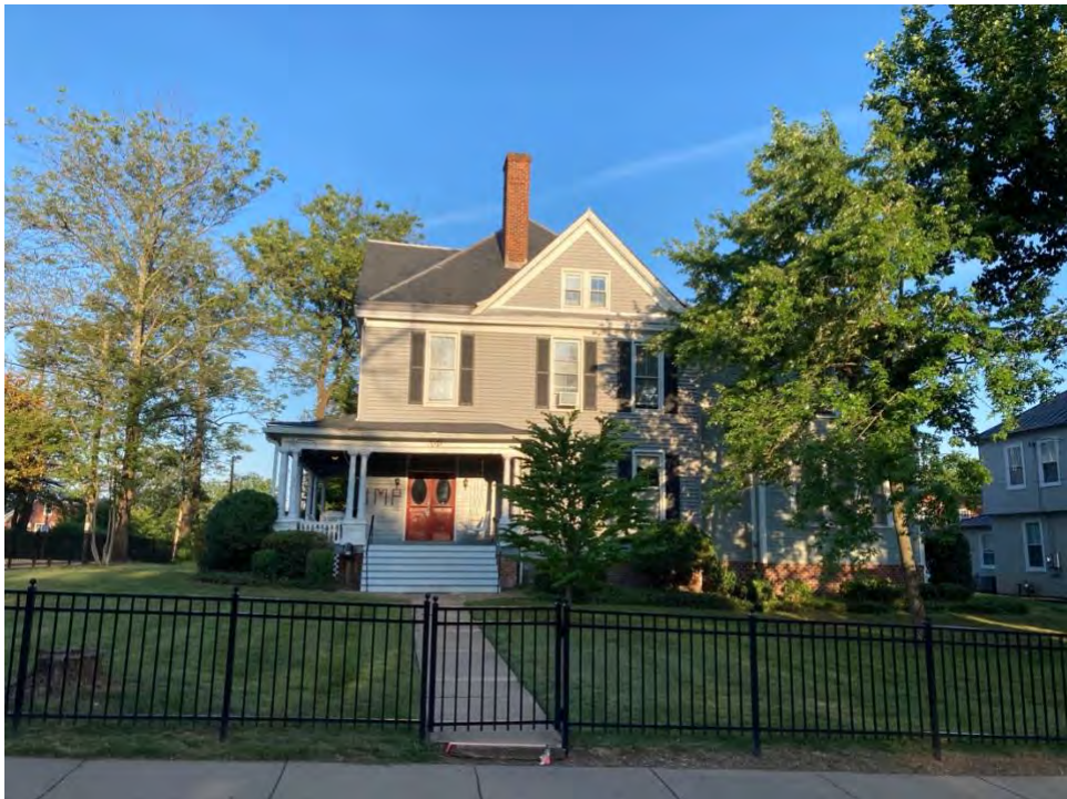
Figure 4: West elevation of 518 17 th Street NW.
