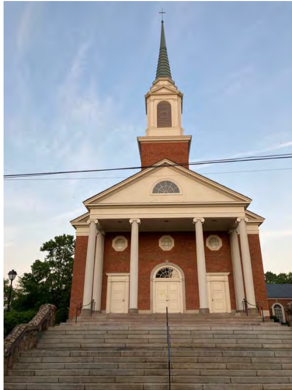
Figure 1: West elevation of 506 Park Street.
