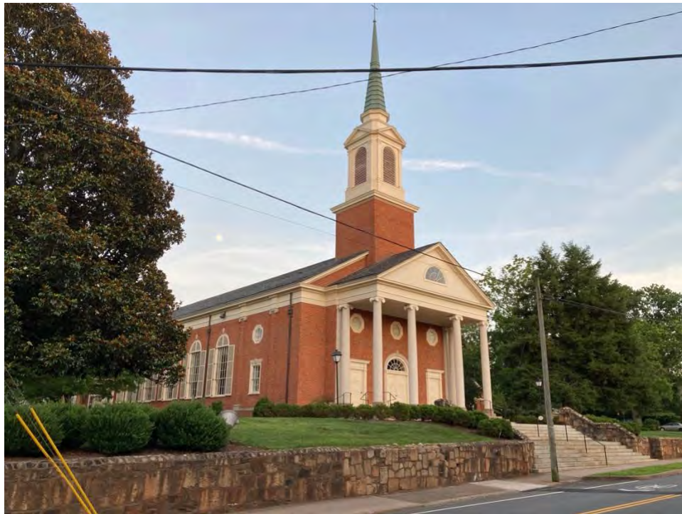
Figure 2: Oblique view of 506 Park Street, facing southeast
