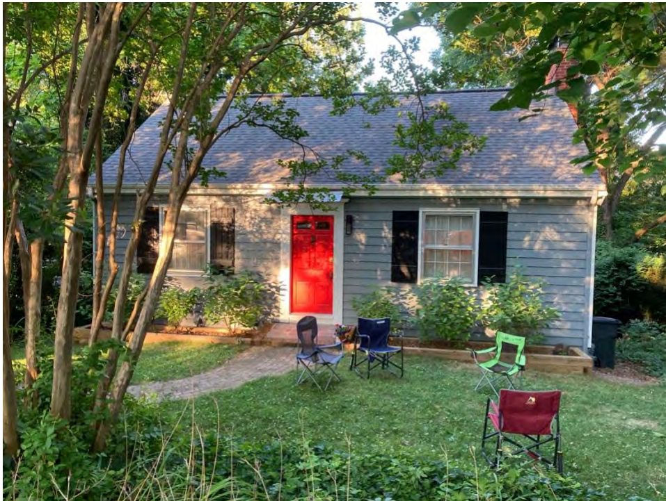
Figure 2: West elevation of 120 Oakhurst Circle.
