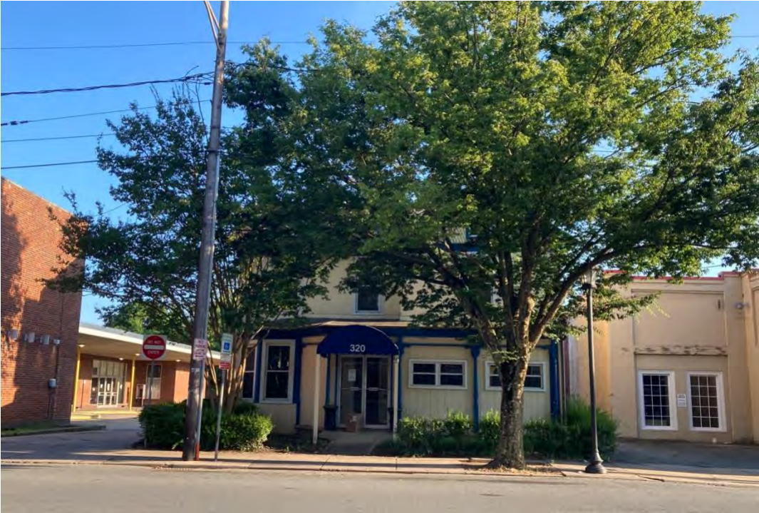
Figure 2: North elevation of 320 West Main Street.
