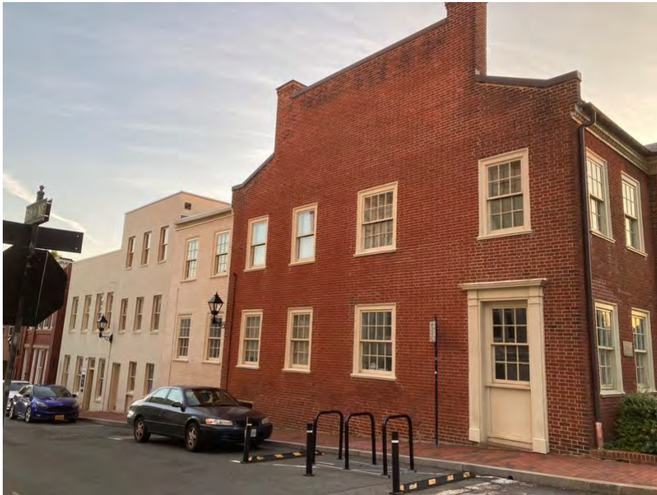
Figure 4: Oblique view of 418 East Jefferson Street, facing southwest.
