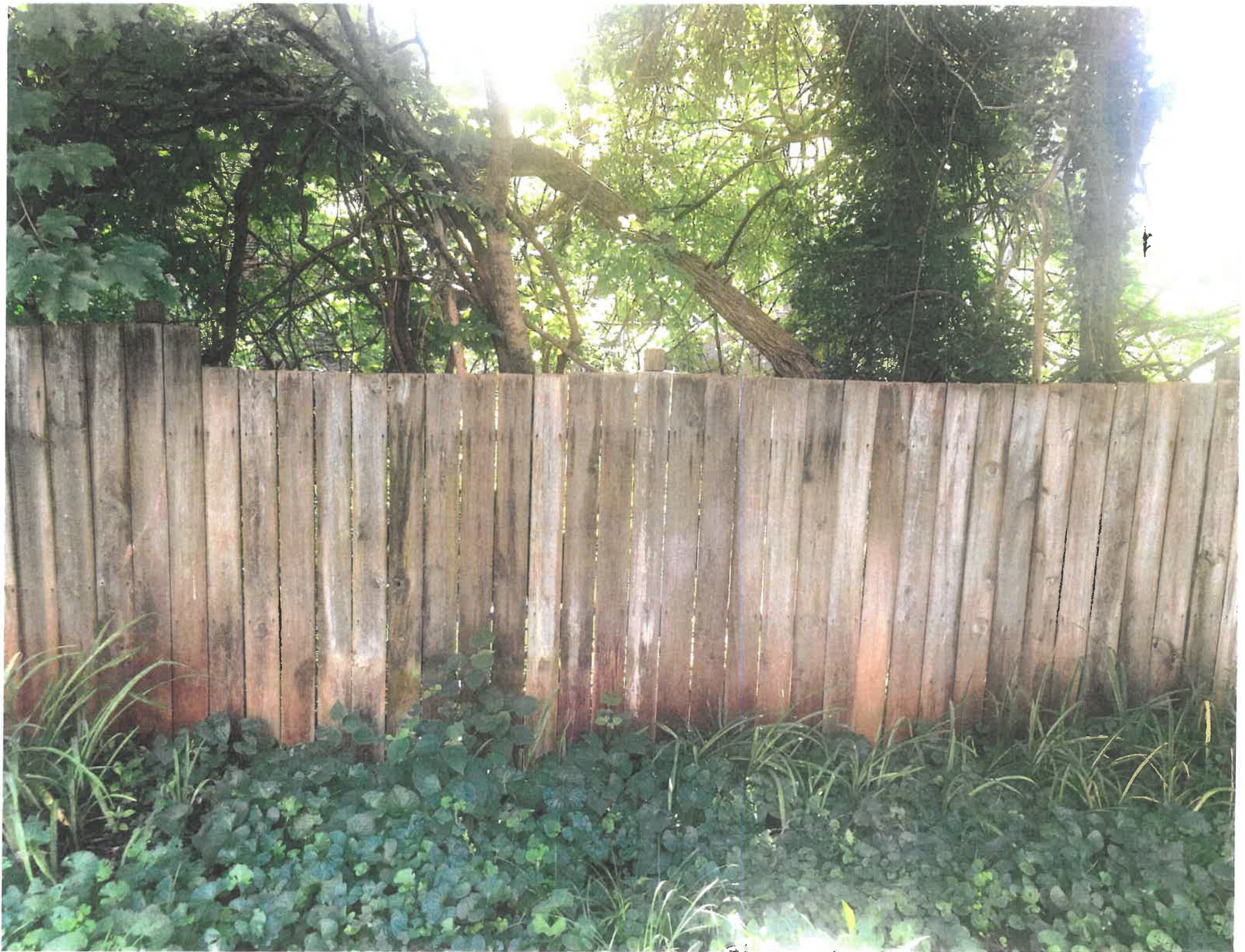
EXISTING DEAD FENCE TO BE REMOVED AND REBUILT
