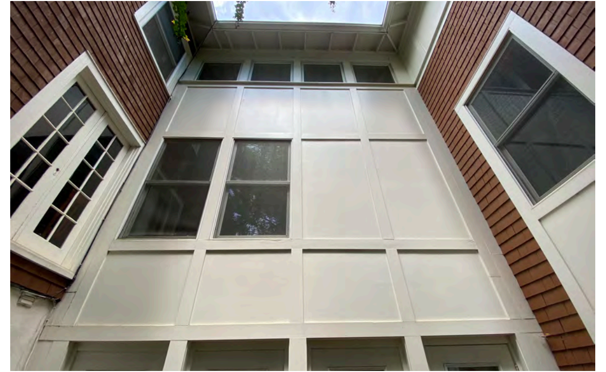
3. 1996 ADDITION - SOUTH ELEVATION - DETAIL OF WOOD PANELING
