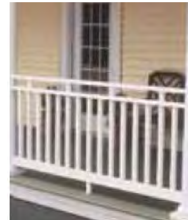
2. SIDE PORCH RAILING
