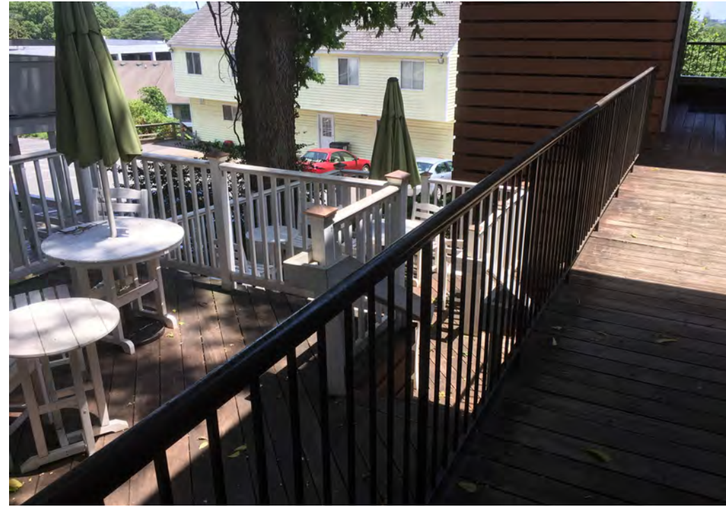
2. NORTH WOOD DECKS
