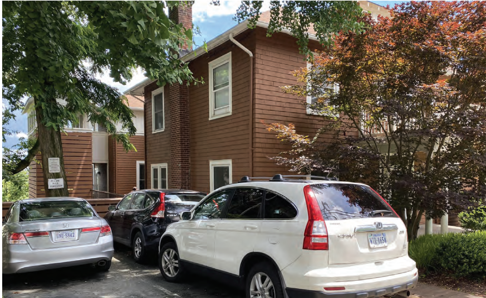
Existing view from Chancellor Street sidewalk
