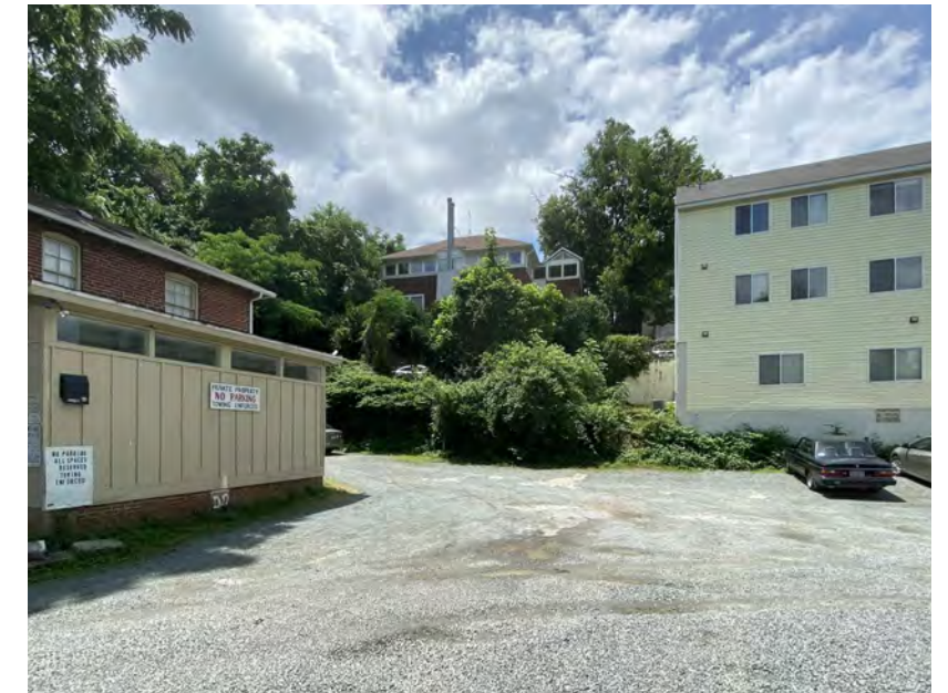
5. 1996 ADDITION EAST (ELLIEWOOD AVE)
