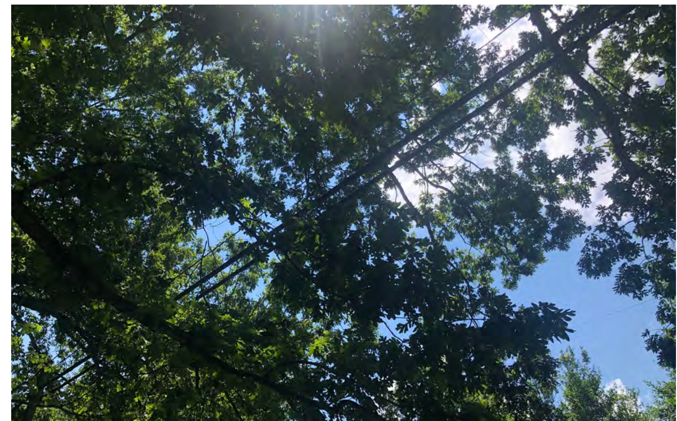
Branches of 24" DBH white oak in tel/data lines (power across street)
