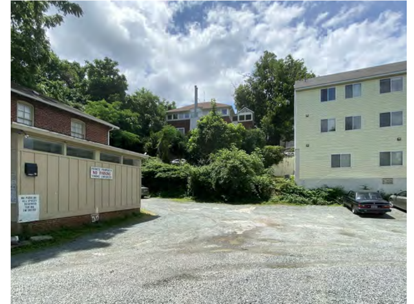
5. 1996 ADDITION EAST (ELLIEWOOD AVE)
