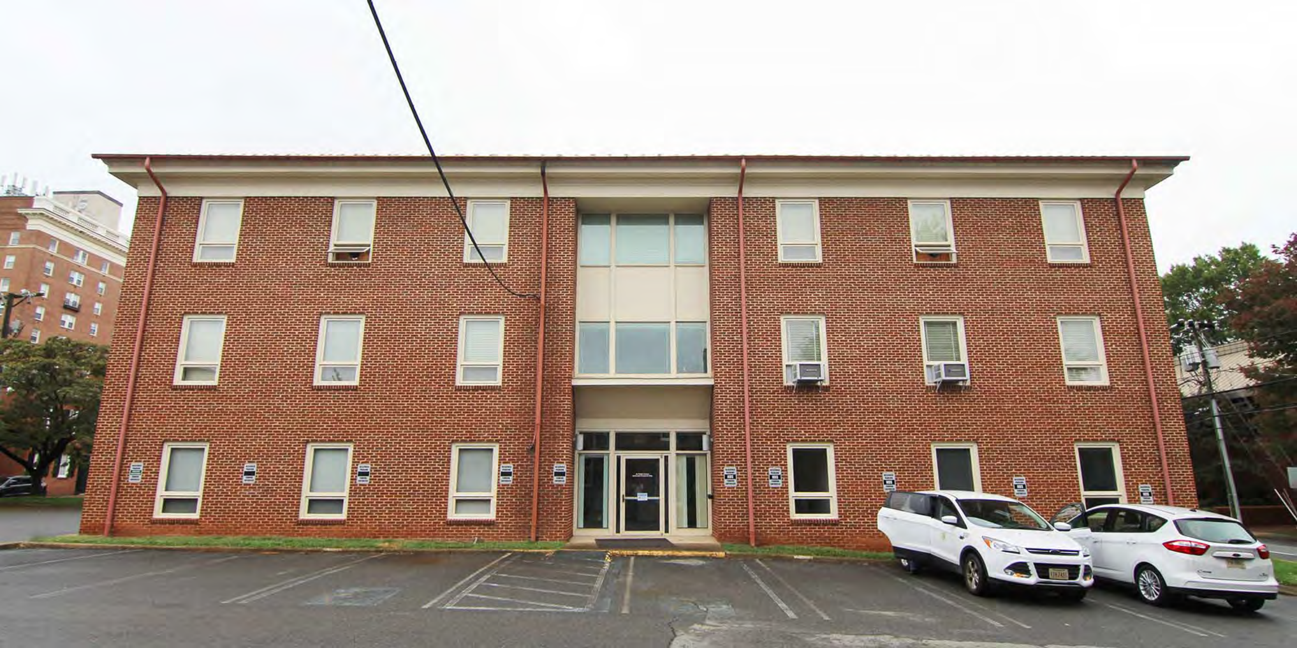
Levy Building Annex: East Facade
