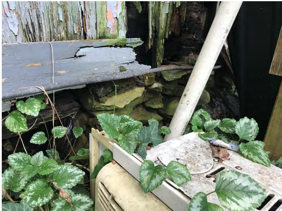
Cottage foundation detail
