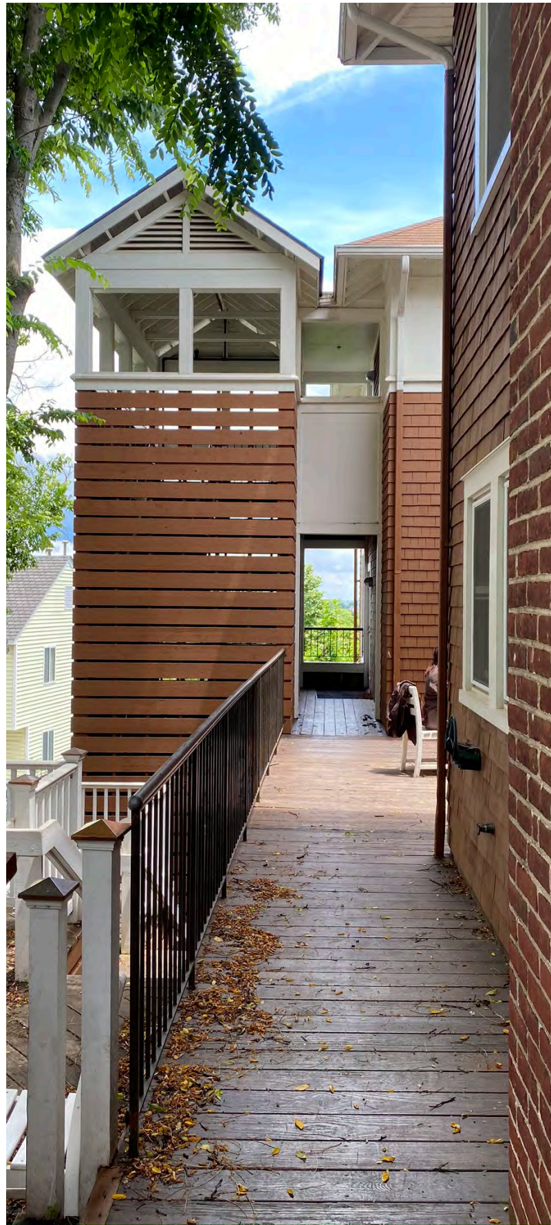
1. NORTH WALK LOOKING EAST
