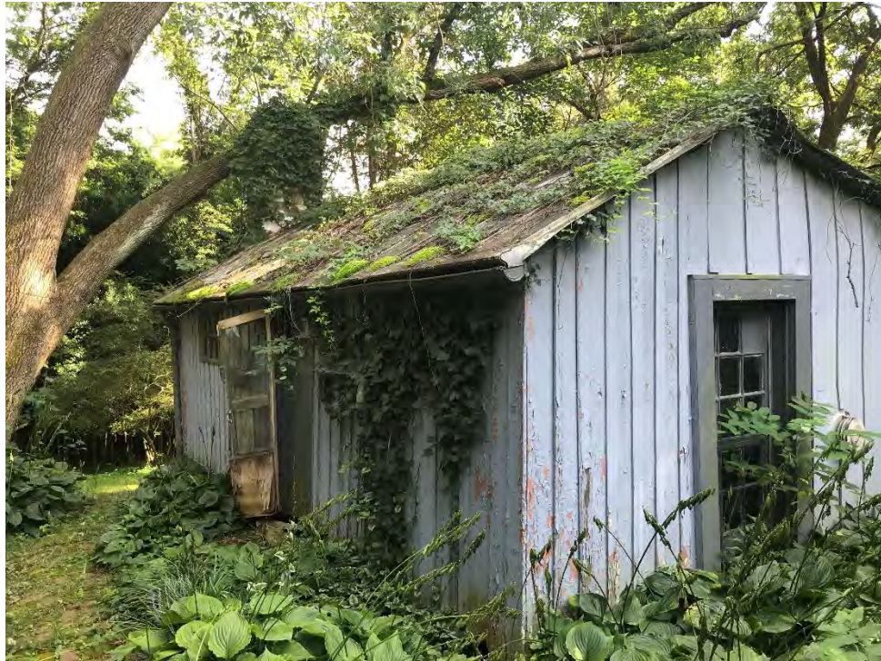
Cottage front view from rear of main structure
