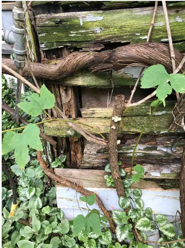
Cottage foundation detail
