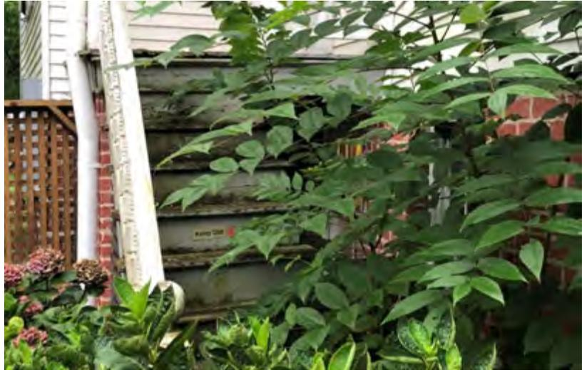
The stair and landing framing and decking appear to be water damaged. The stair stringer connections to the landing are questionable. The main beam supporting the stair stringers has limited bearing over the brick pier.
