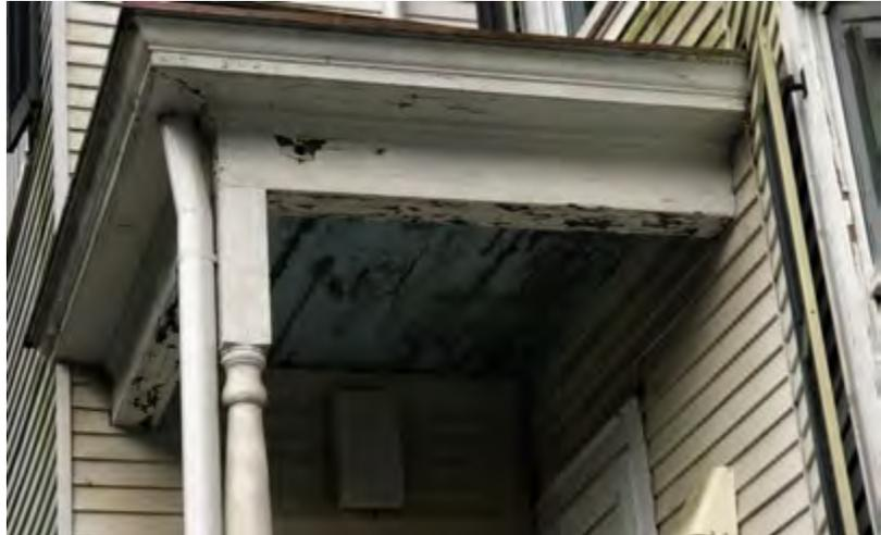
The existing wood framing of the porch landing, stairs and roof are in poor structural condition. The stability of the structure is questionable and it should not be occupied. In our opinion, given the extent of the damage, repair to the existing structure would not be practical. If the structure is intended to be used, we recommend a complete replacement that is designed to be comply with current building code requirements.
