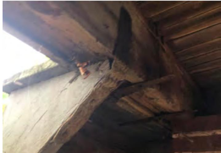
The treads and risers are water damaged.
