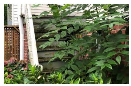
The stair and landing framing and decking appear to be water damaged. The stair stringer connections to the landing are questionable. The main beam supporting the stair stringers has limited bearing over the brick pier.
