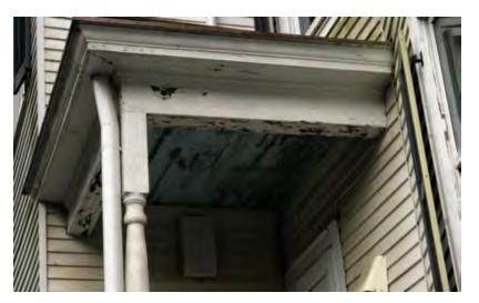
The existing wood framing of the porch landing, stairs and roof are in poor structural condition. The stability of the structure is questionable and it should not be occupied. In our opinion, given the extent of the damage, repair to the existing structure would not be practical. If the structure is intended to be used, we recommend a complete replacement that is designed to be comply with current building code requirements.
