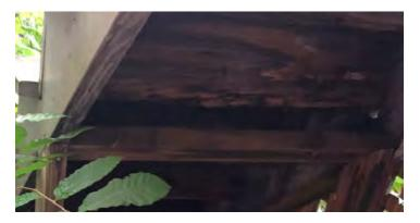
The treads and risers are water damaged.
