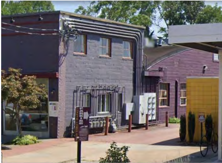
2205-09 Fontaine Avenue. Within an Entrance Corridor. Exterior ductwork and conduits enclosed with prefinished metal panels.
