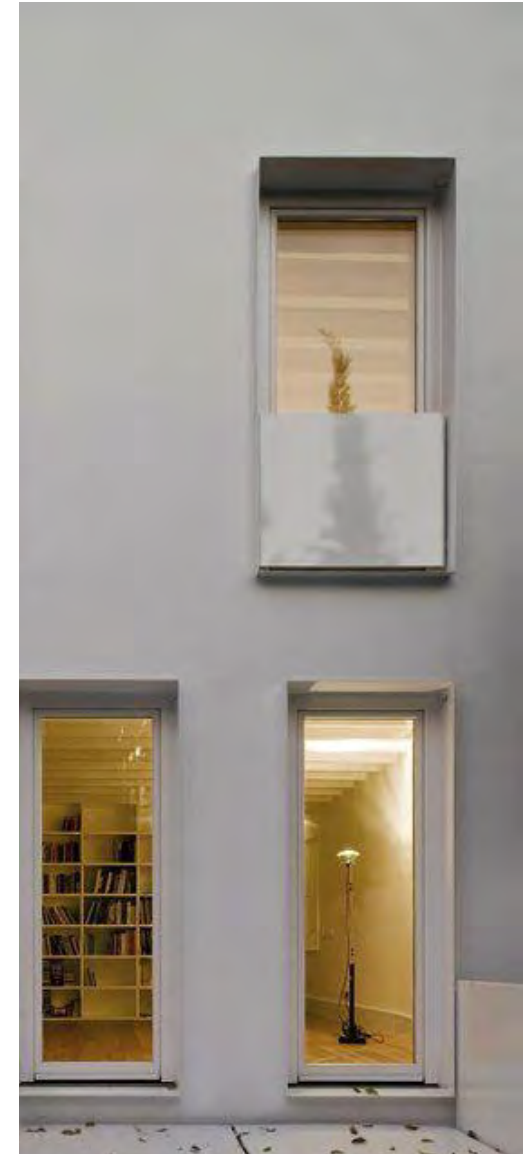
STUCCO EXTERIOR WITH METAL WINDOW SURROUNDS
