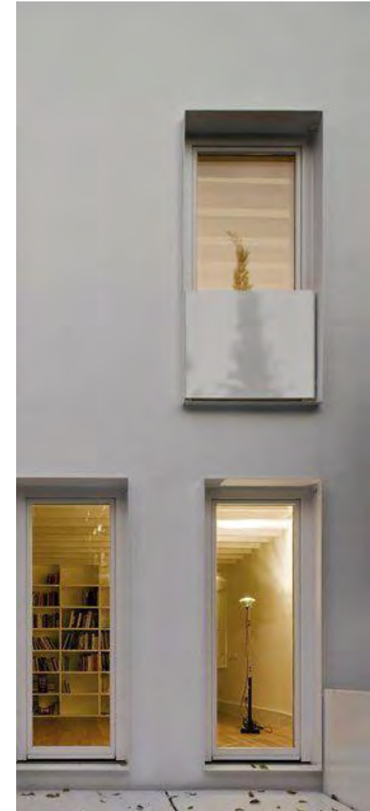
STUCCO EXTERIOR WITH METAL WINDOW SURROUNDS
