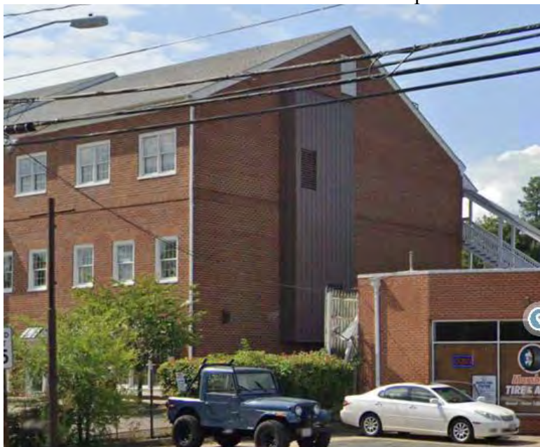
2205-09 Fontaine Avenue. Within an Entrance Corridor. Exterior ductwork and conduits enclosed with prefinished metal panels.
