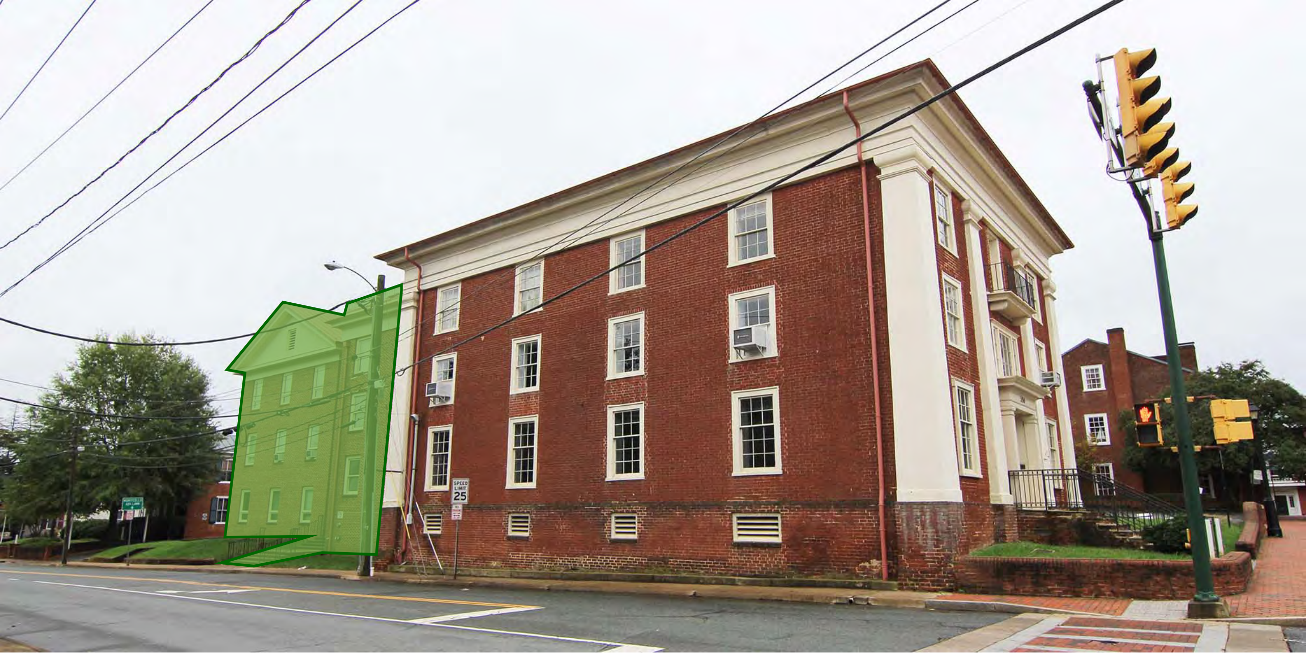
Levy Building: Northwest Corner
