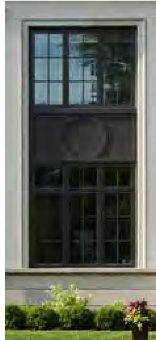
STUCCO EXTERIOR WITH CAST STONE WINDOW SURROUNDS
