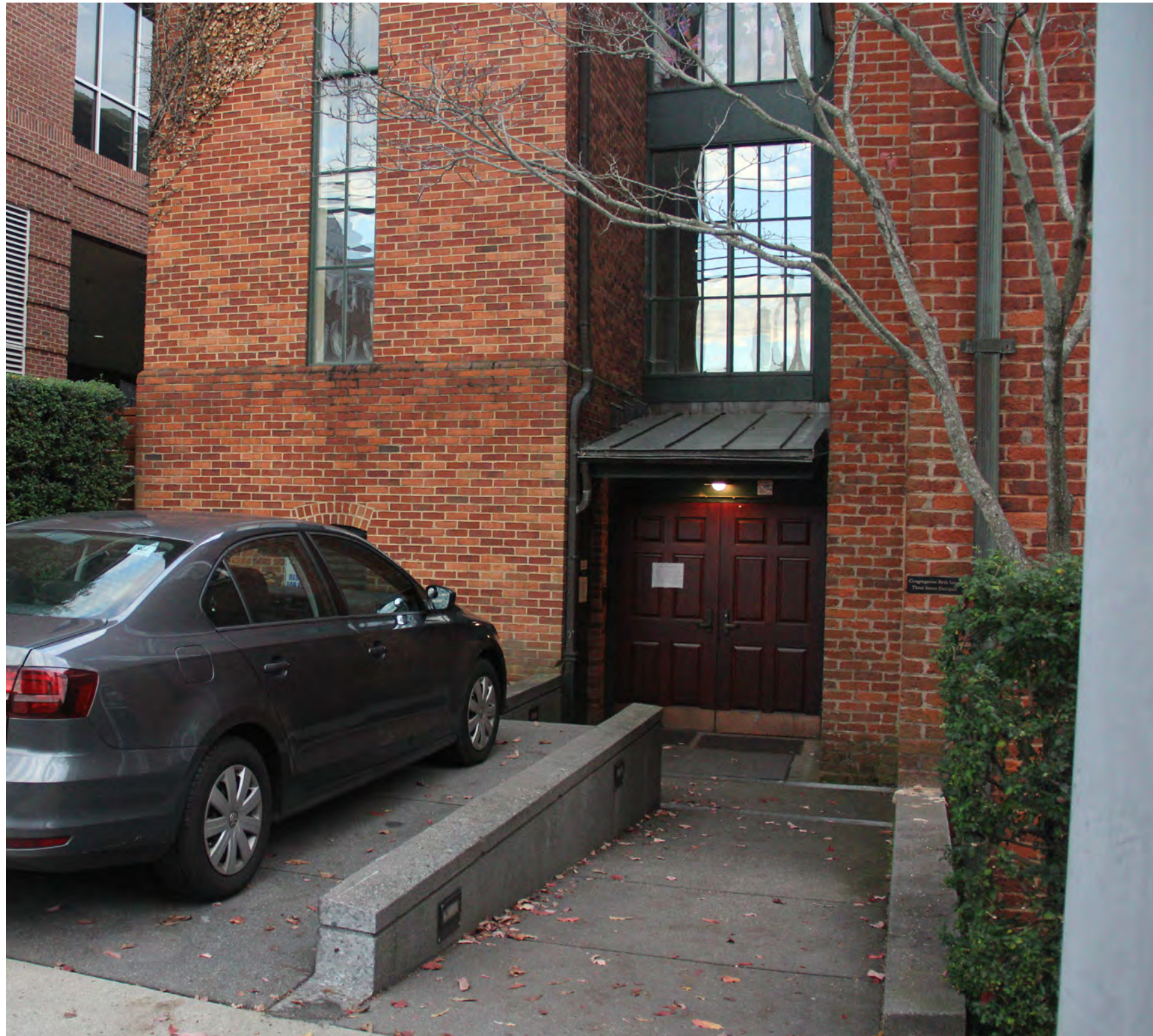
3RD STREET ENTRY
