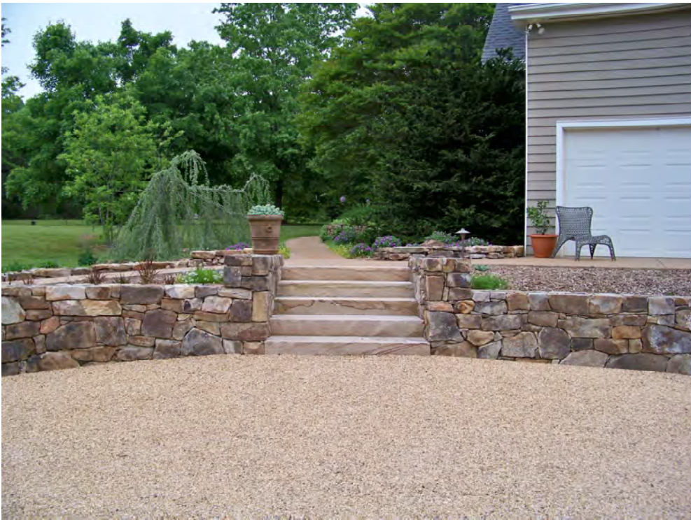
Proposed Fieldstone Retaining Walls and Free-Standing Walls: All proposed walls to be CMU block walls with fieldstone veneer in a dry-laid appearance laying style with raked joints. The proposed walls to have the same appearance as the above precedent images.
