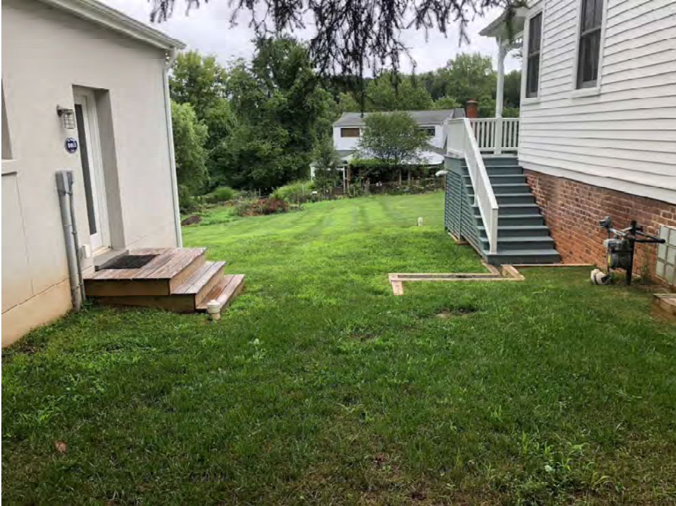
between the garage studio and the main house looking northeast existing timber walls and risers, wooden steps into garage studio
