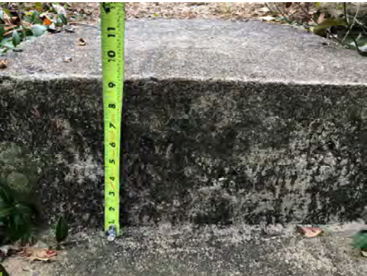
concrete steps - top riser is 9"
