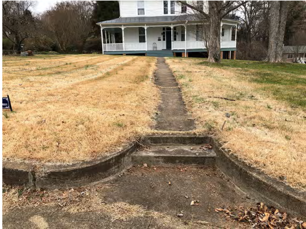
front concrete walkway and steps looking from the park street sidewalk
