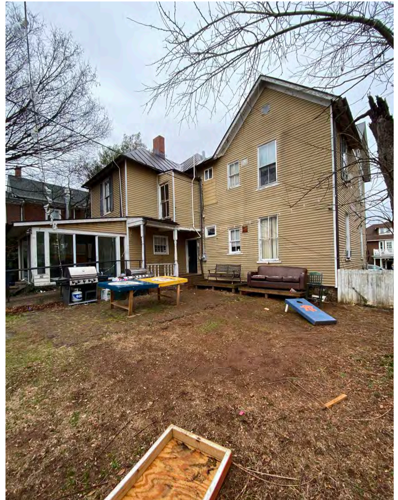
Existing Exterior S/W REAR OF HOUSE
