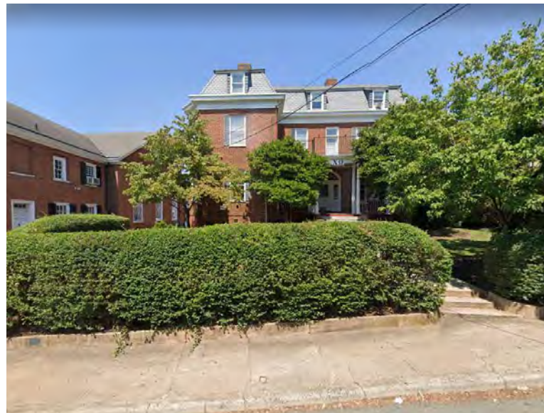
123 Chancellor St - Chi Omega - Built 1902
