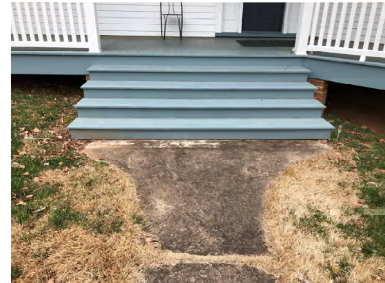
concrete landing at the bottom of the front porch steps
