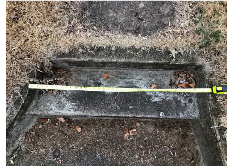
front concrete steps are 38.5" wide, front walkway is 36" wide
