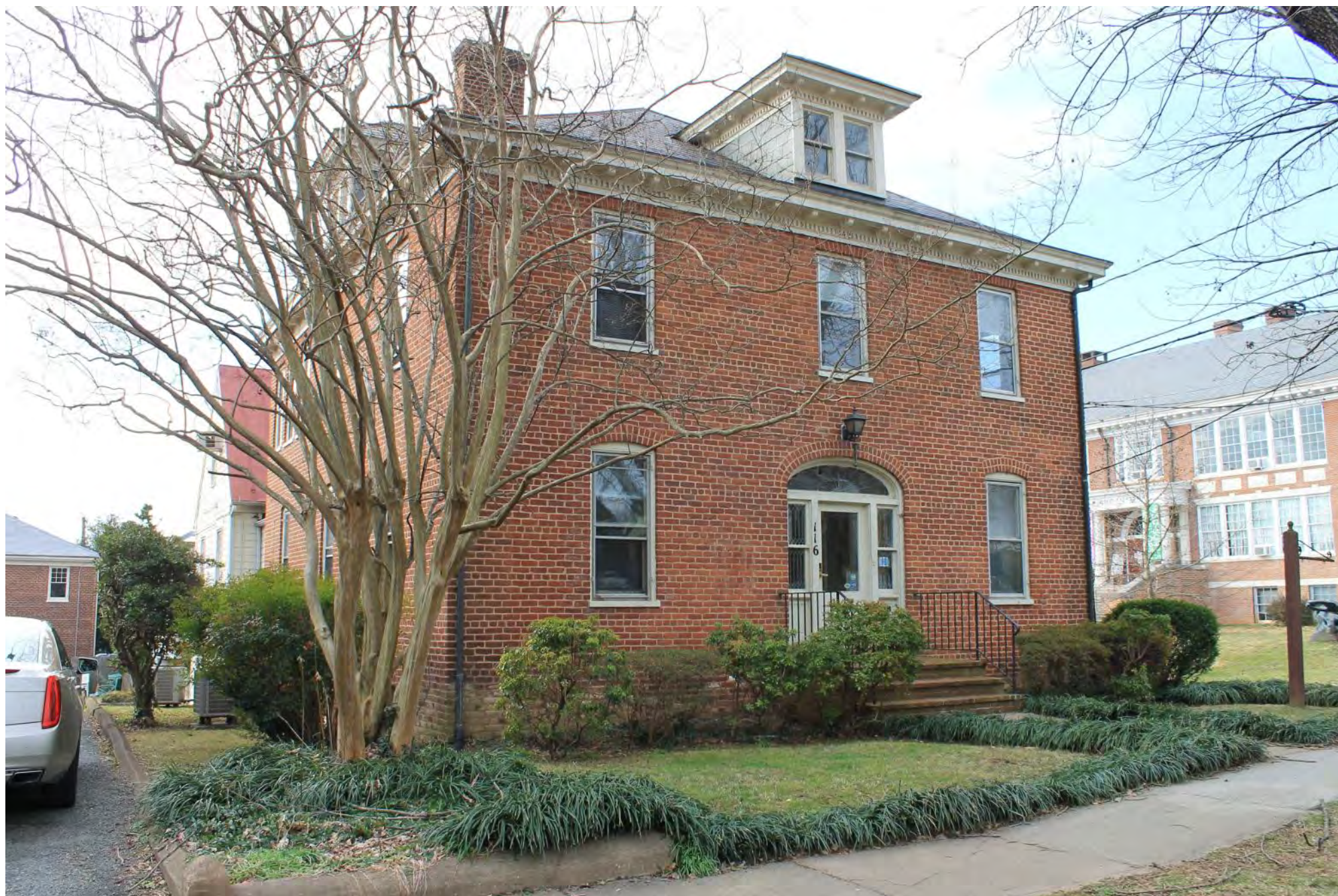
North Elevation—from W. Jefferson
