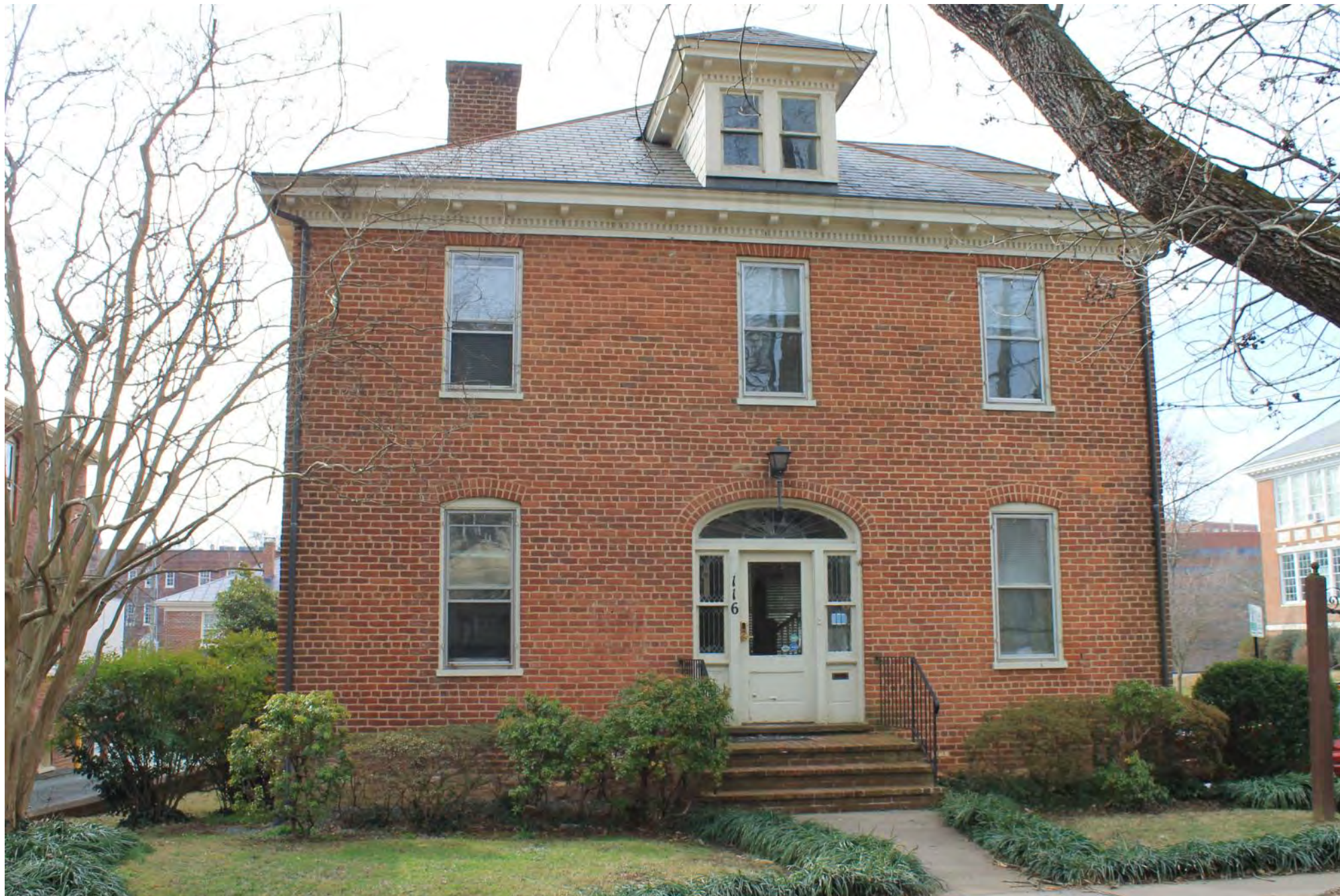
North Elevation—from W. Jefferson
