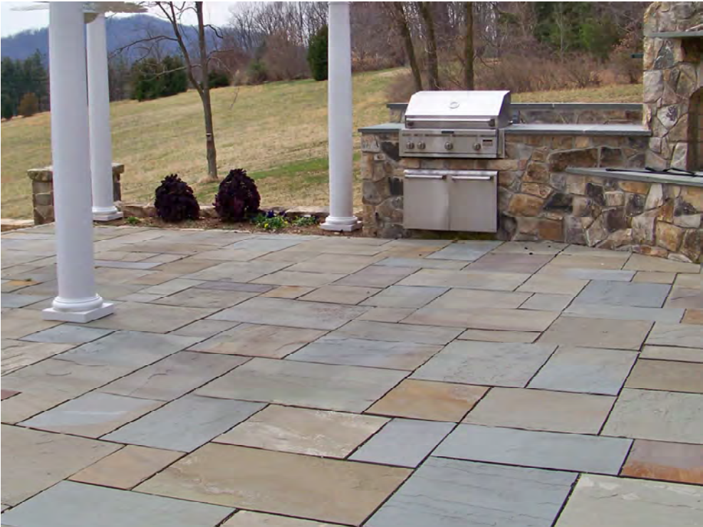
Proposed Fieldstone Retaining Walls and Free-Standing Walls: All proposed walls to be CMU block walls with fieldstone veneer in a dry-laid appearance laying style with raked joints. The proposed walls to have the same appearance as the above precedent images.
