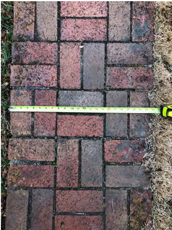
walkway and steps are 23" wide
