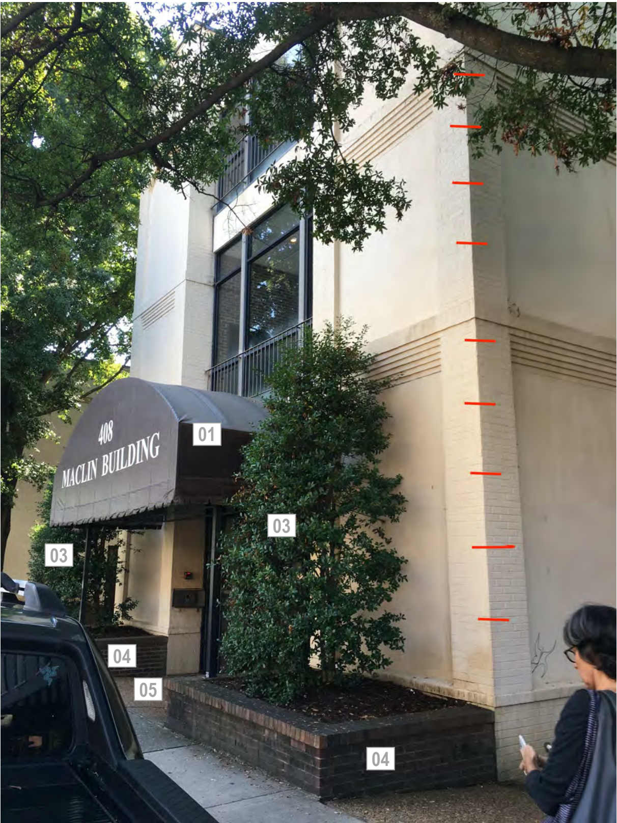
FRONT ENTRY - SIDEWALK APPROACH
