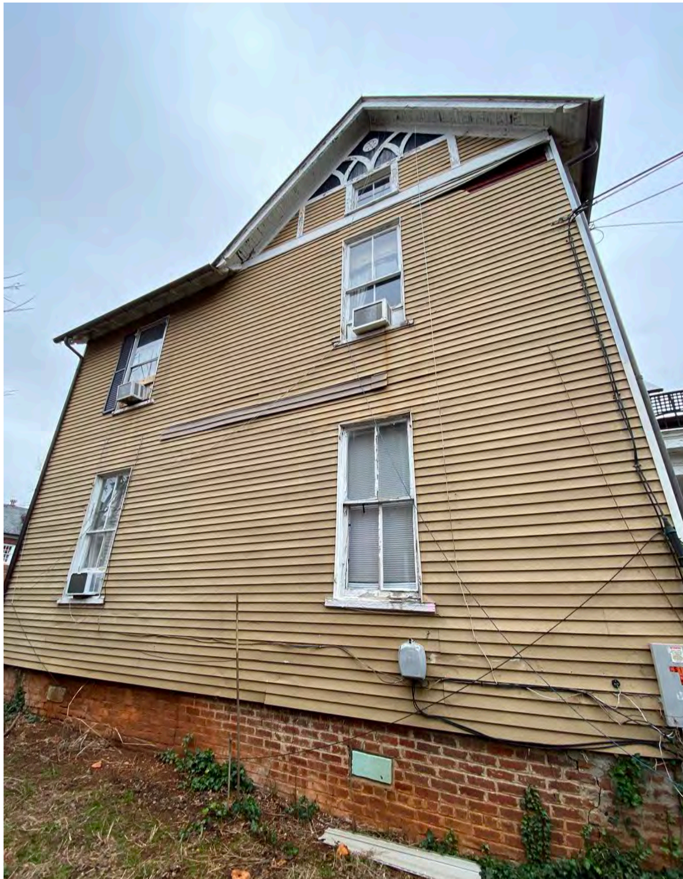
Existing Exterior SOUTH SIDE OF HOUSE
