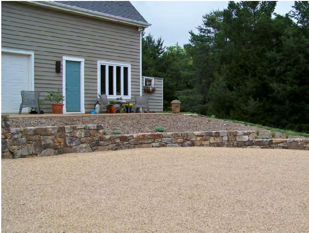
Proposed Fieldstone Retaining Walls and Free-Standing Walls: All proposed walls to be CMU block walls with fieldstone veneer in a dry-laid appearance laying style with raked joints. The proposed walls to have the same appearance as the above precedent images.
