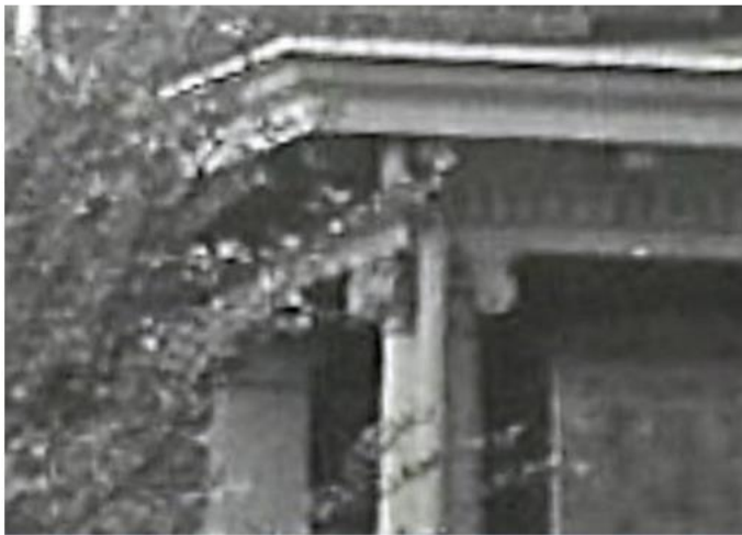
Original porch at 116 West Jefferson
