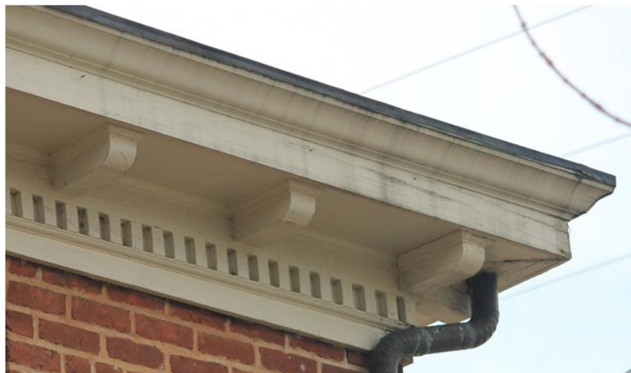
Cornice at 116 West Jefferson St
