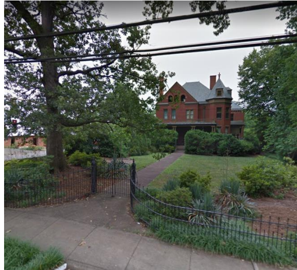
Figure 2: Metal fence at 620 Park Street. Image from Google Street View, 2017
