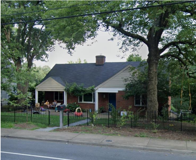
Figure 1: Metal fence at 728 Park Street. Image from Google Street View, 2019.
