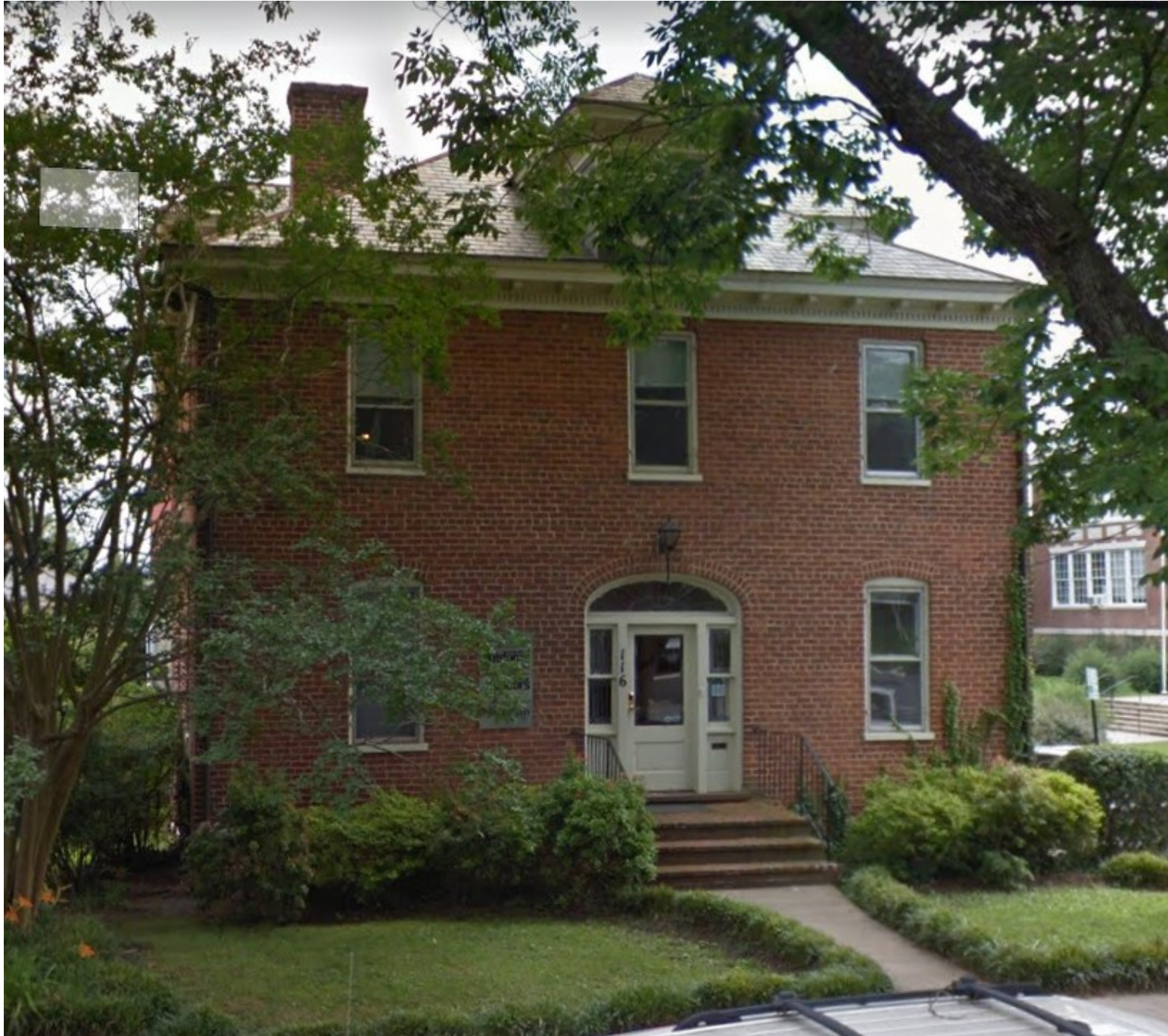
116 West Jefferson Street - Revercomb House c.1913 - Photo from Google street view (June 2018)
