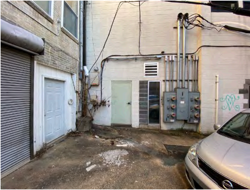
VIEW EAST PAST FACADE
