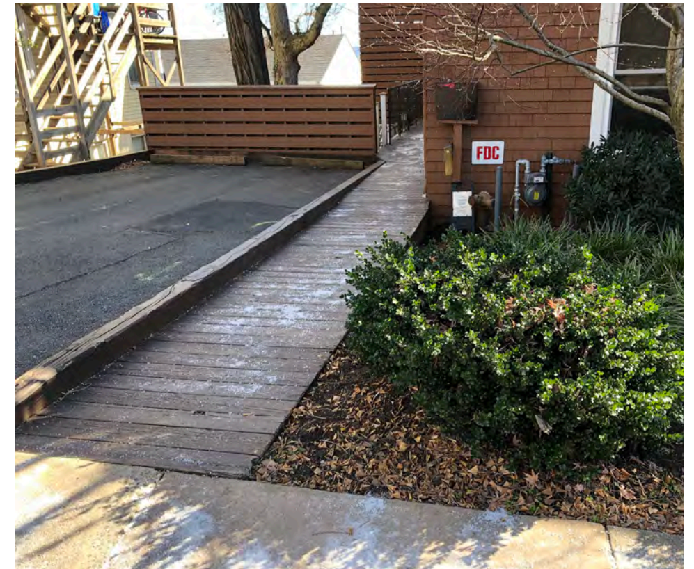
5. EXISTING PARKING AND WALKWAY
