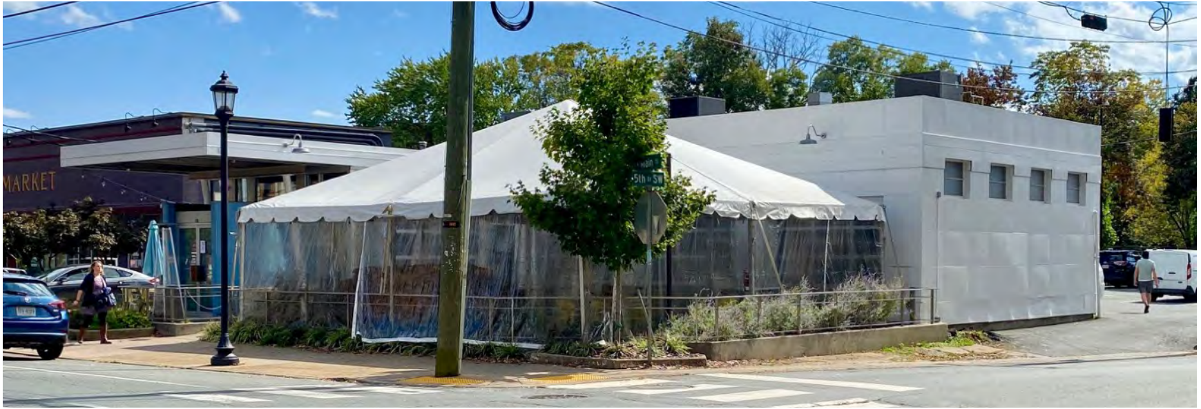
NORTHWEST FACADE WITH TEMPORARY TENT
