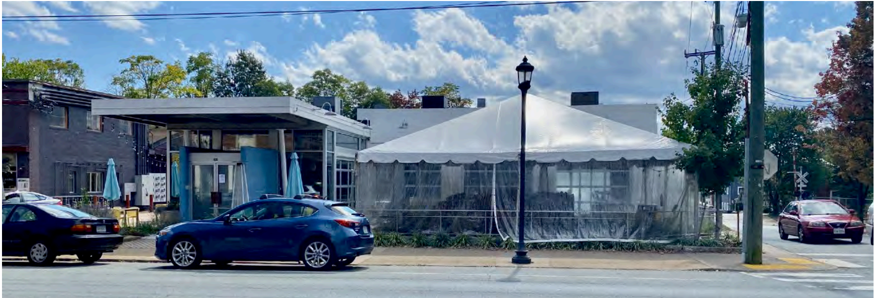
NORTH FACADE WITH TEMPORARY TENT
