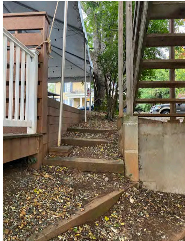
3. EXISTING NORTH TIMBER STAIRS
