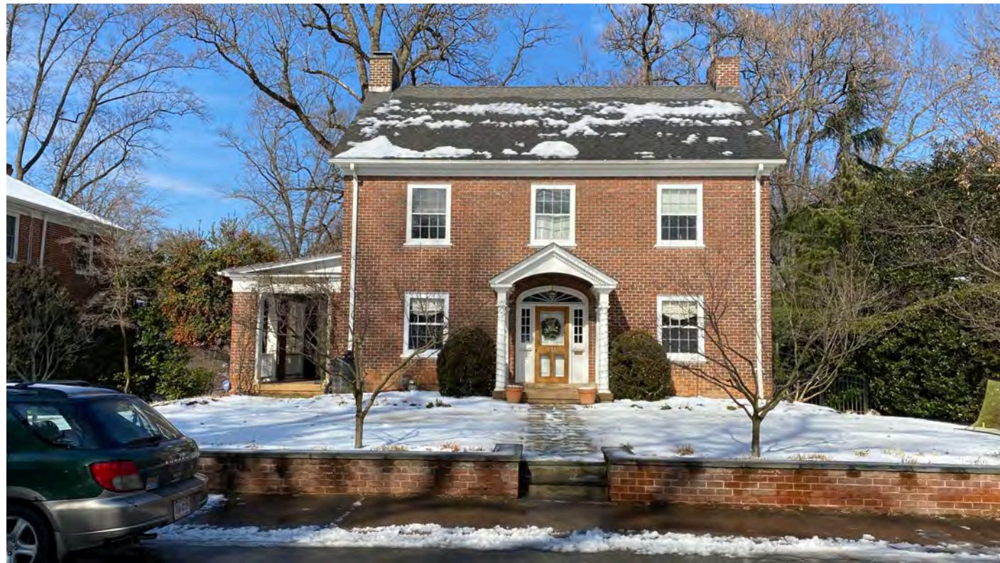
735 Northwood Dormer Addition + Tesla Roof + Copper Gutters
