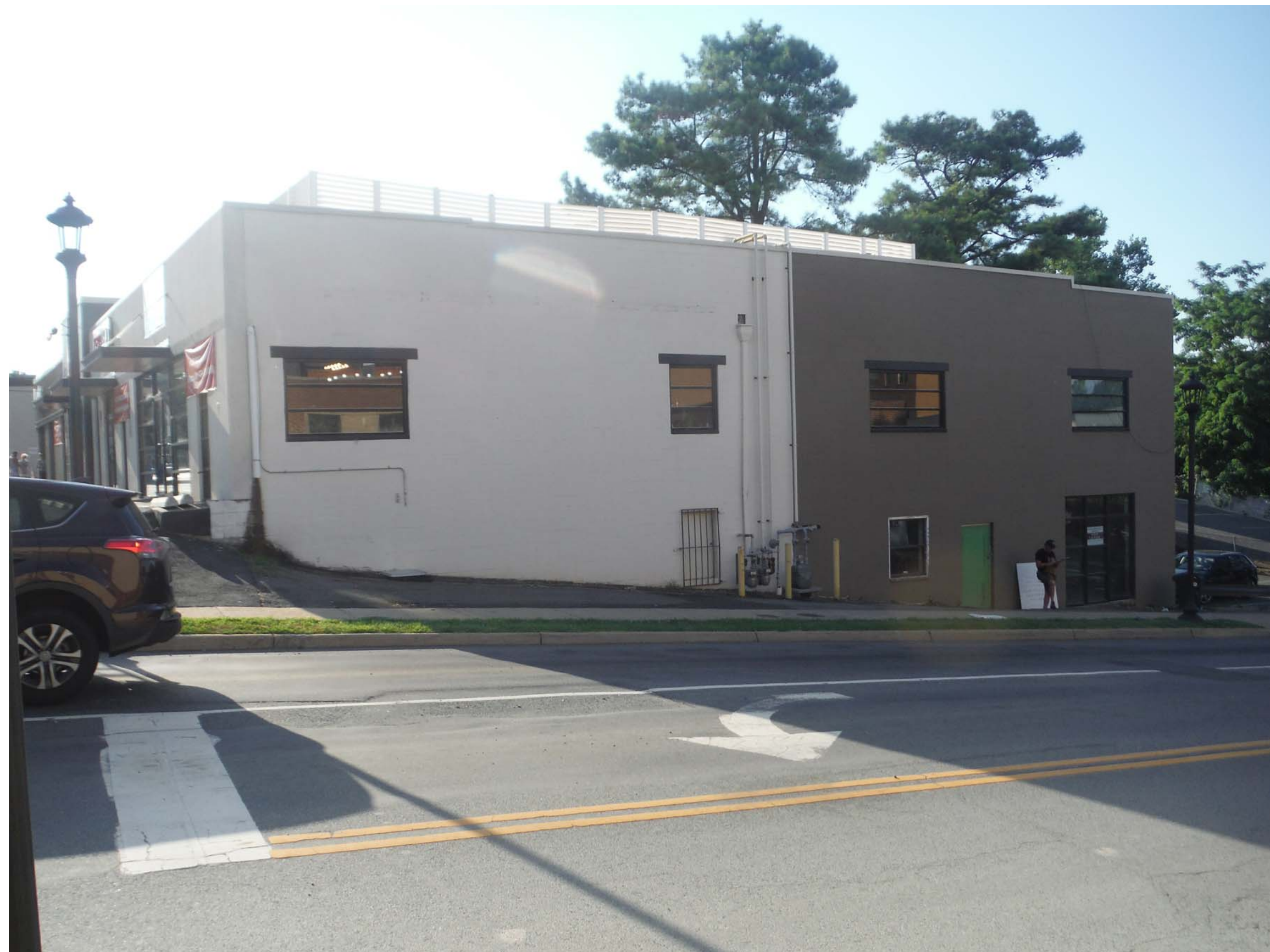
EXISTING PHOTO - EAST
