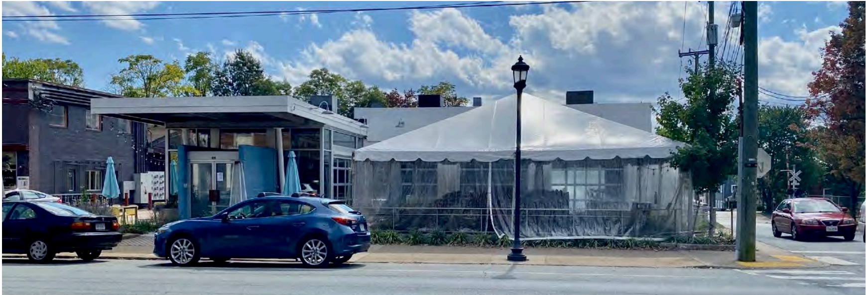
NORTH FACADE WITH TEMPORARY TENT
