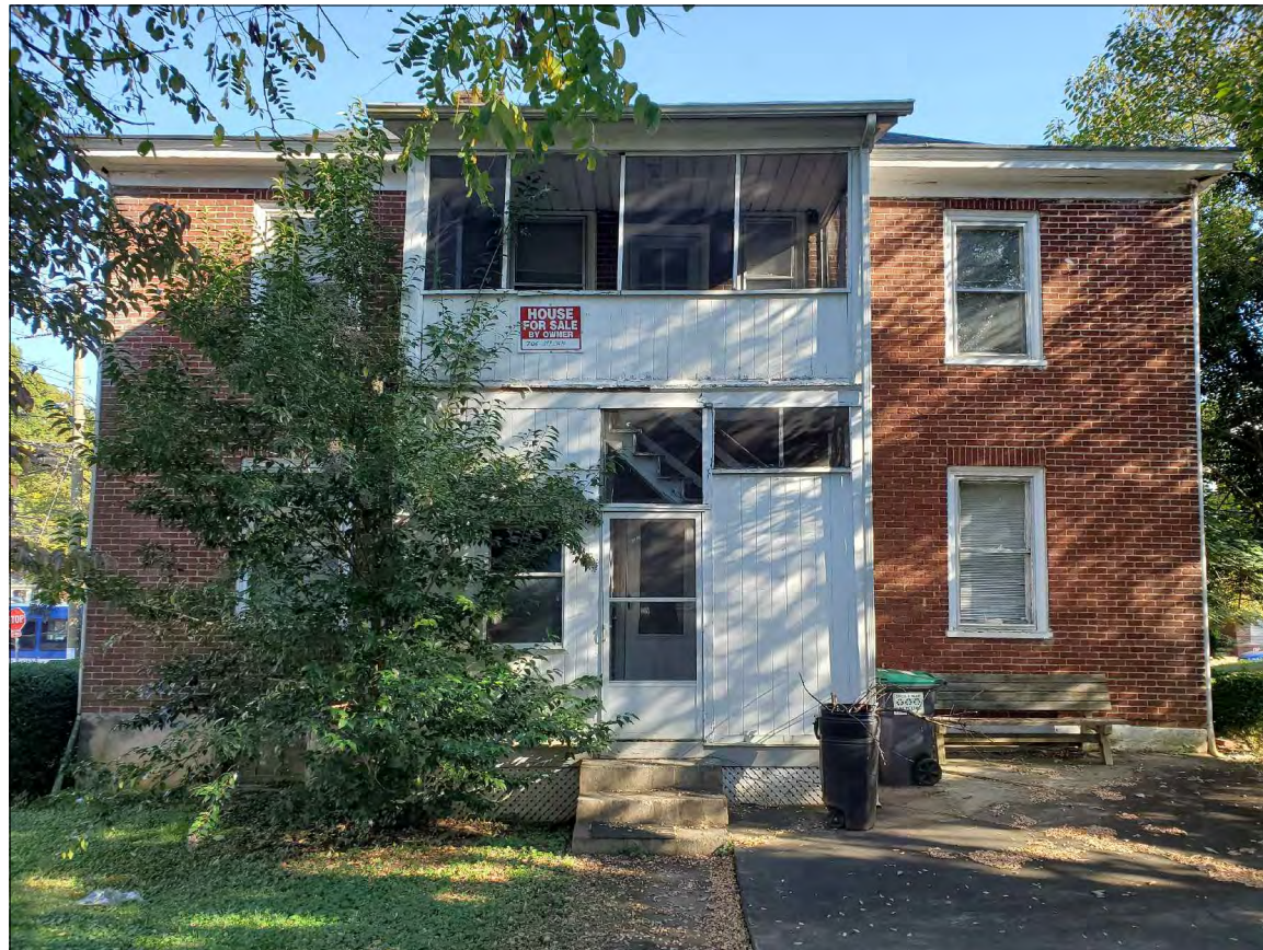
REAR OF RESIDENCE FROM ALLEY
