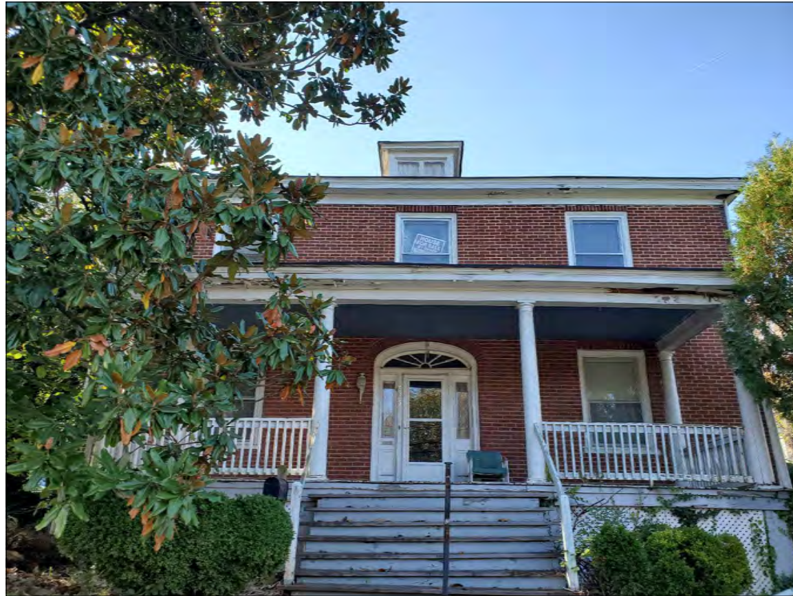
FRONT OF RESIDENCE FROM 14TH STREET
