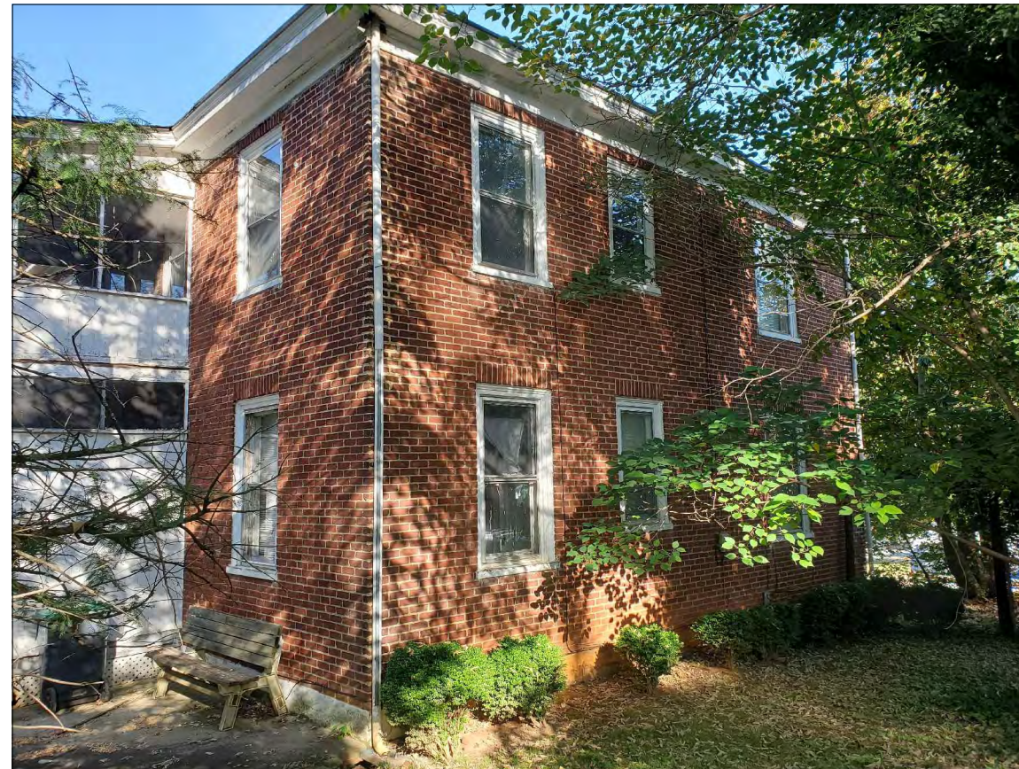
SIDE OF RESIDENCE FROM ADJACENT PROPERTY
