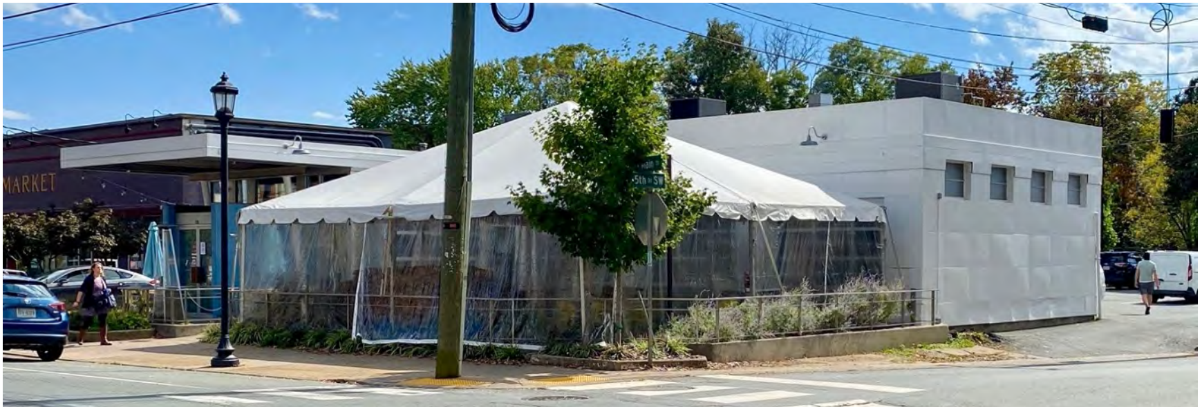
NORTHWEST FACADE WITH TEMPORARY TENT
