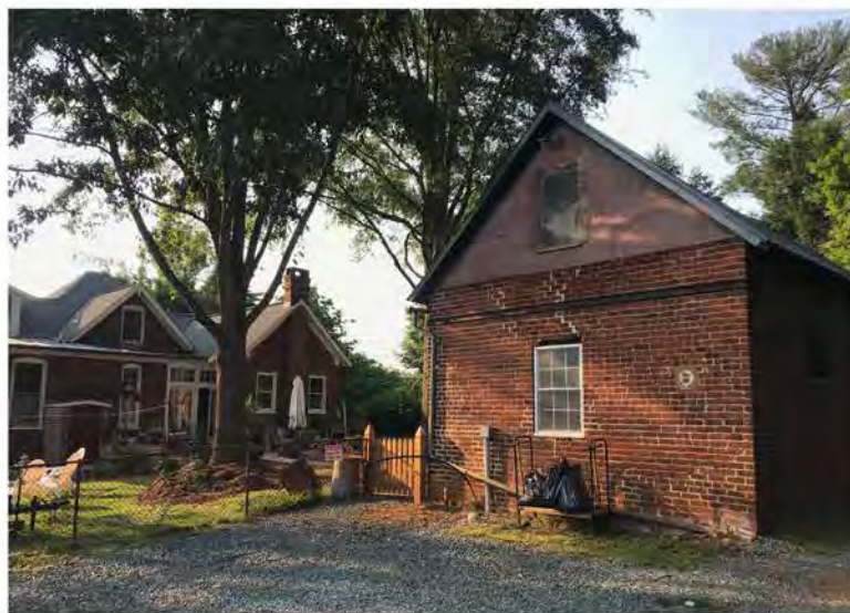
VIEW FROM ALLEY TO HOUSE & CARRIAGE HOUSE (SOURCE G+G)
