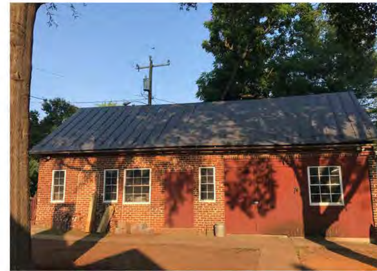
VIEW FROM MAIN HOUSE EAST PORCH TO CARRIAGE HOUSE (SOURCE G+G)
