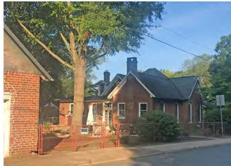
REAR POST RENOVATION, VIEW FROM HAZEL STREET (SOURCE: G+G)
