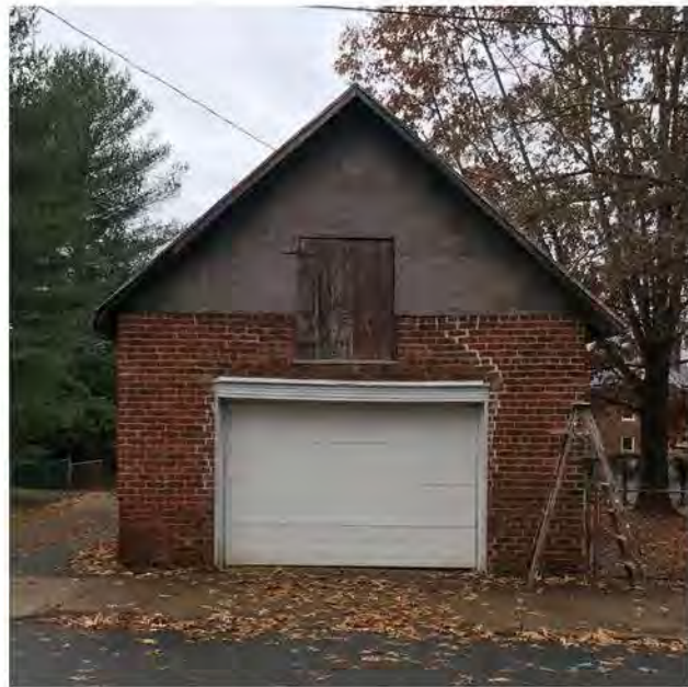
HAZEL ST (NORTH) FACADE
