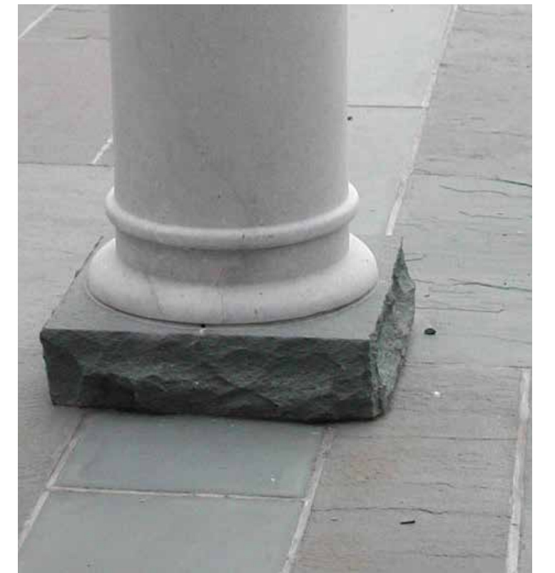
BLUESTONE PAVING AT COLUMN
