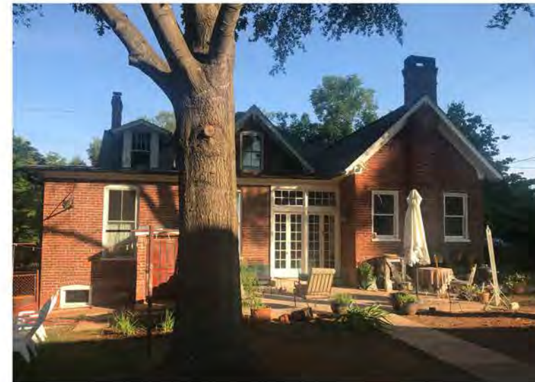
REAR POST RENOVATION, VIEW FROM CARRIAGE HOUSE (SOURCE: G+G)
