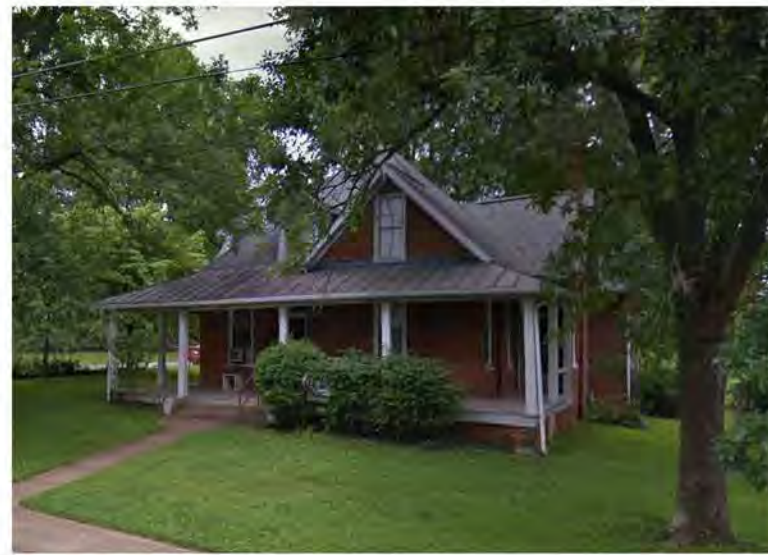
FRONT PRE-RENOVATION (SOURCE GOOGLE)
