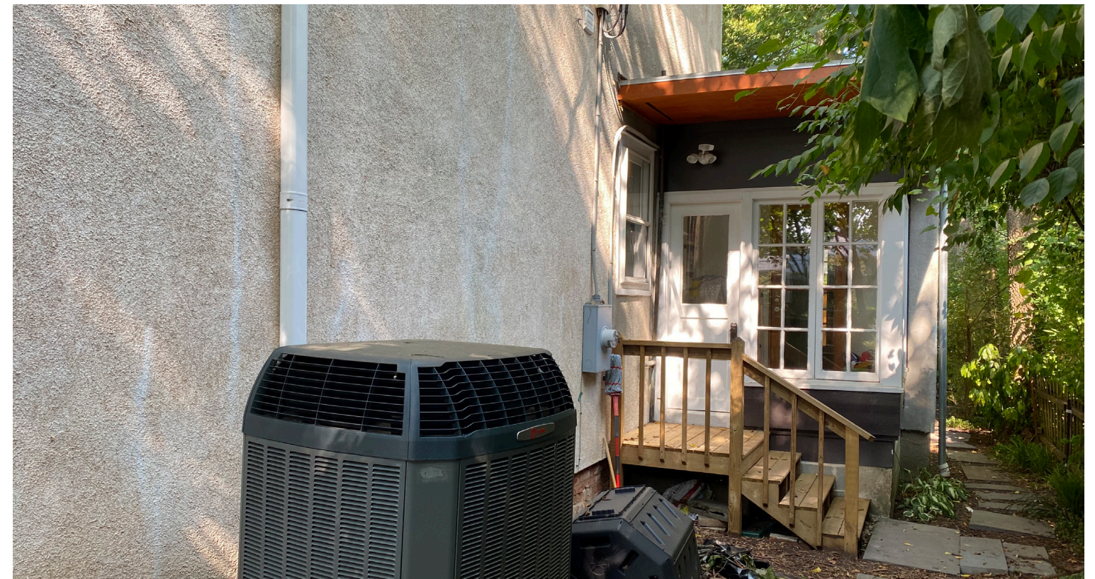
EXISTING CONDITIONS - NORTHEAST
