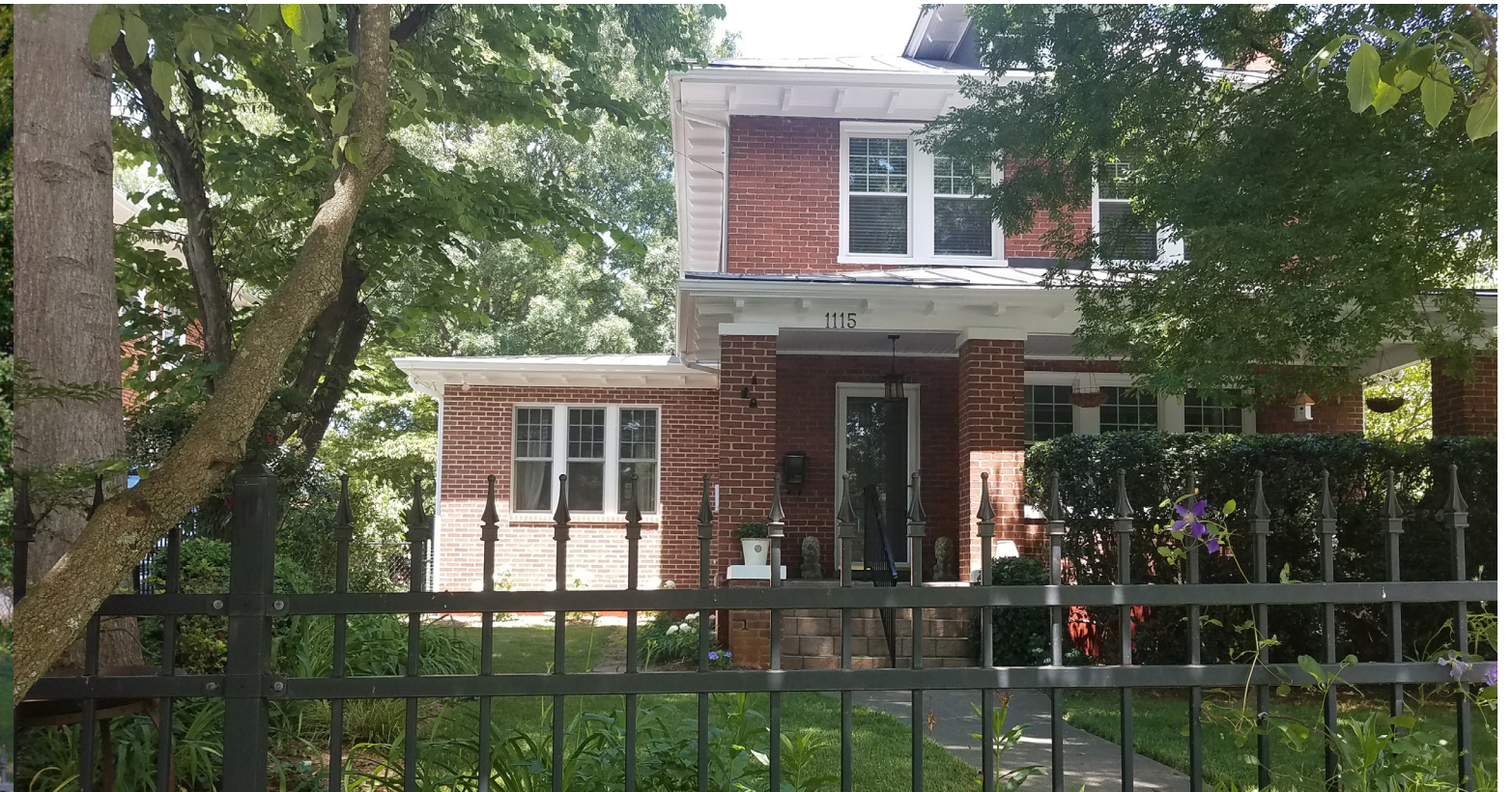
APPROVED ADDITION, COMPLETED
