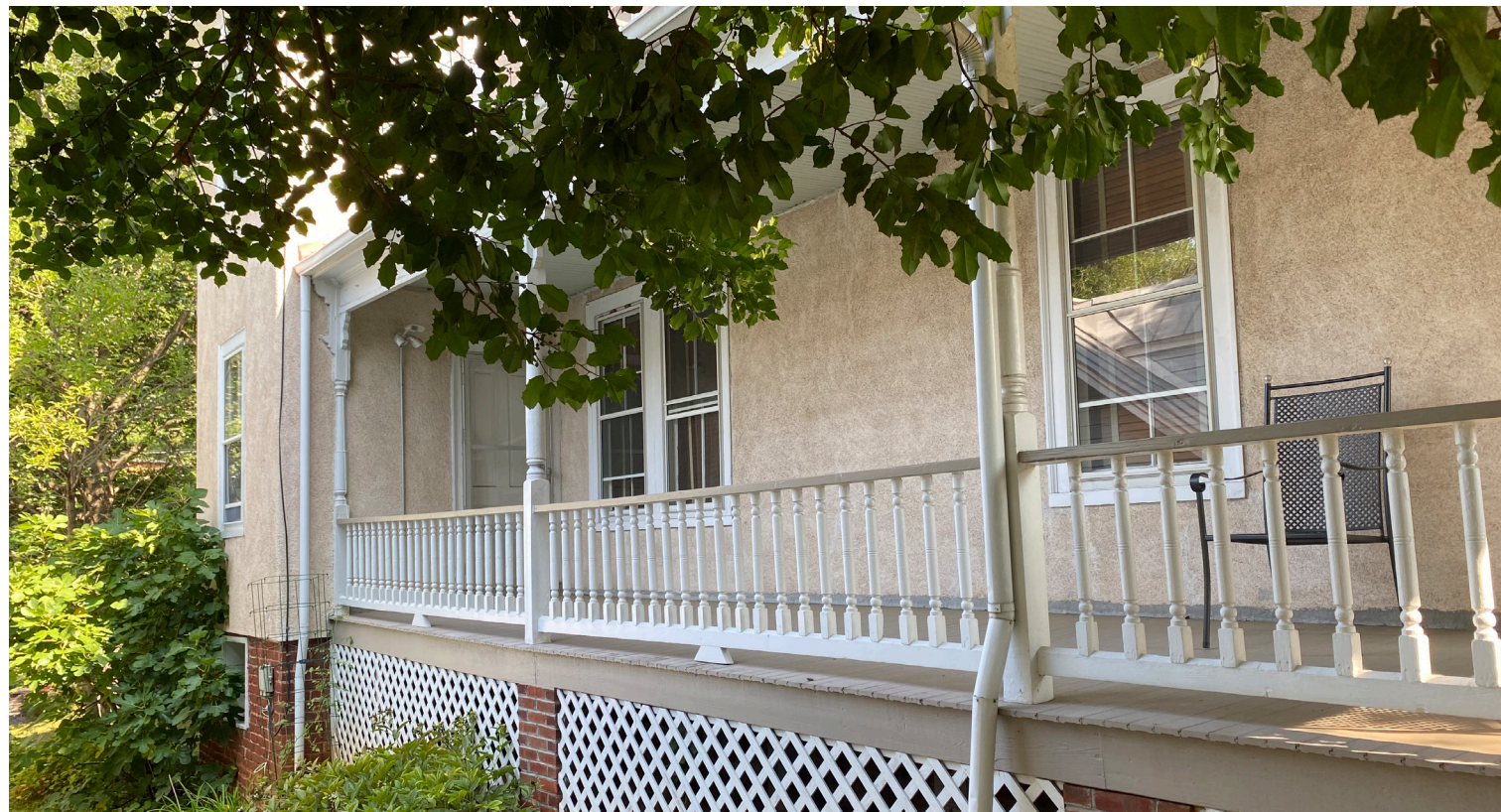
EXISTING CONDITIONS - SOUTHEAST
