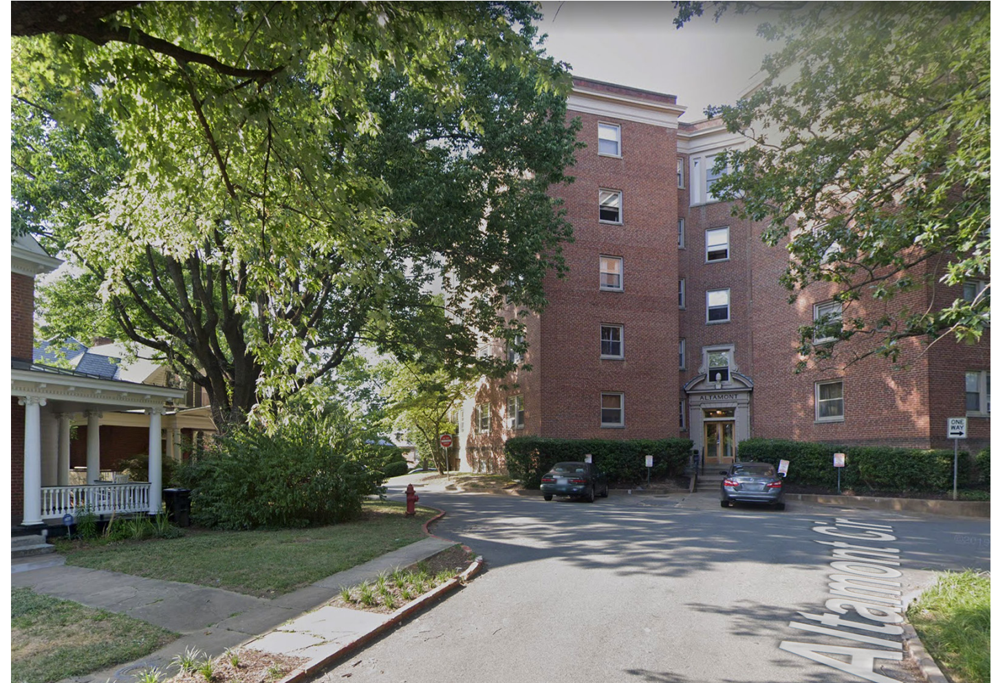
Altamont Circle Apartments
