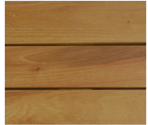
Black Locust Decking (multi-coat clear finish) at balcony floors, stair treads and landings
