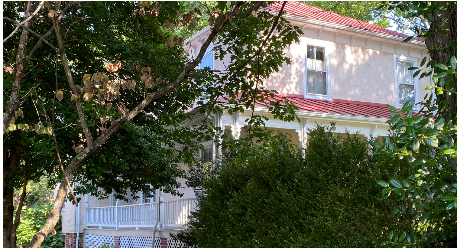
EXISTING CONDITIONS - SOUTHEAST
