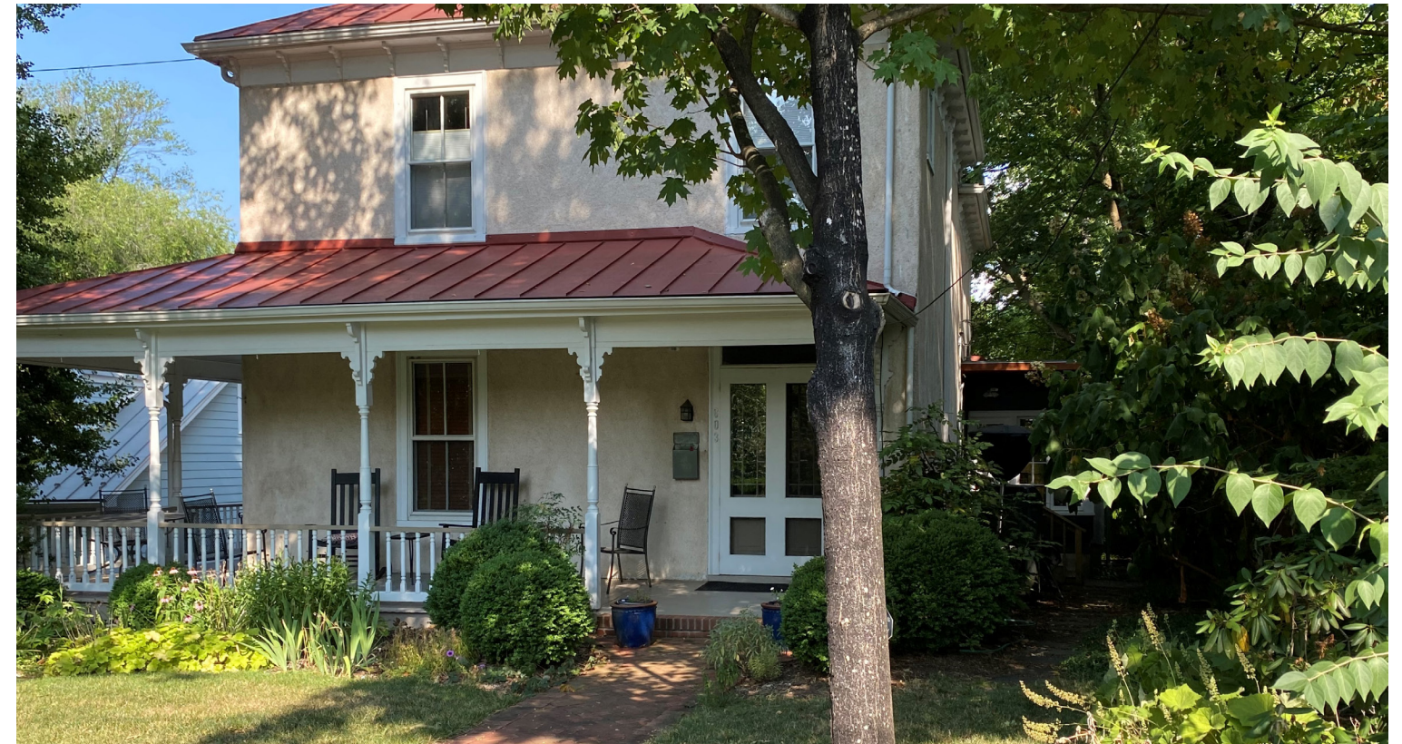
EXISTING CONDITIONS - NORTHEAST
