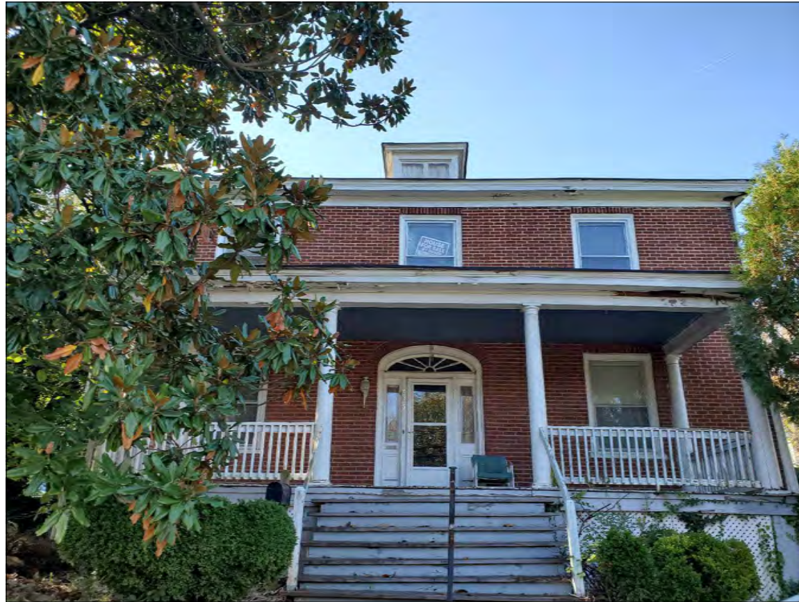
FRONT OF RESIDENCE FROM 14TH STREET
