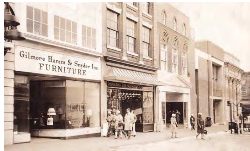
EAST MAIN FACADE, C. 1974
