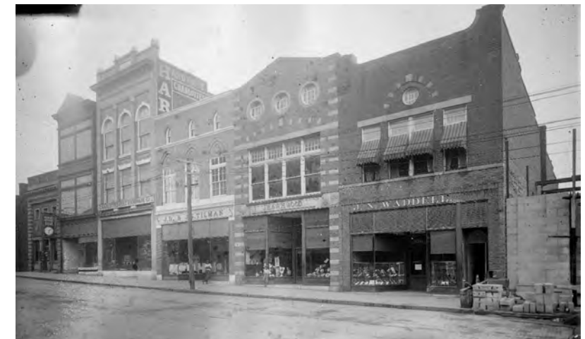
EAST MAIN FACADE, C. 1916
