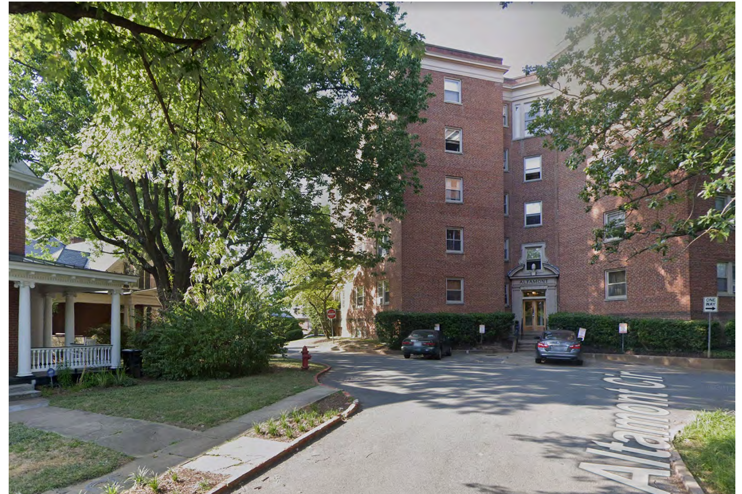
Altamont Circle Apartments
