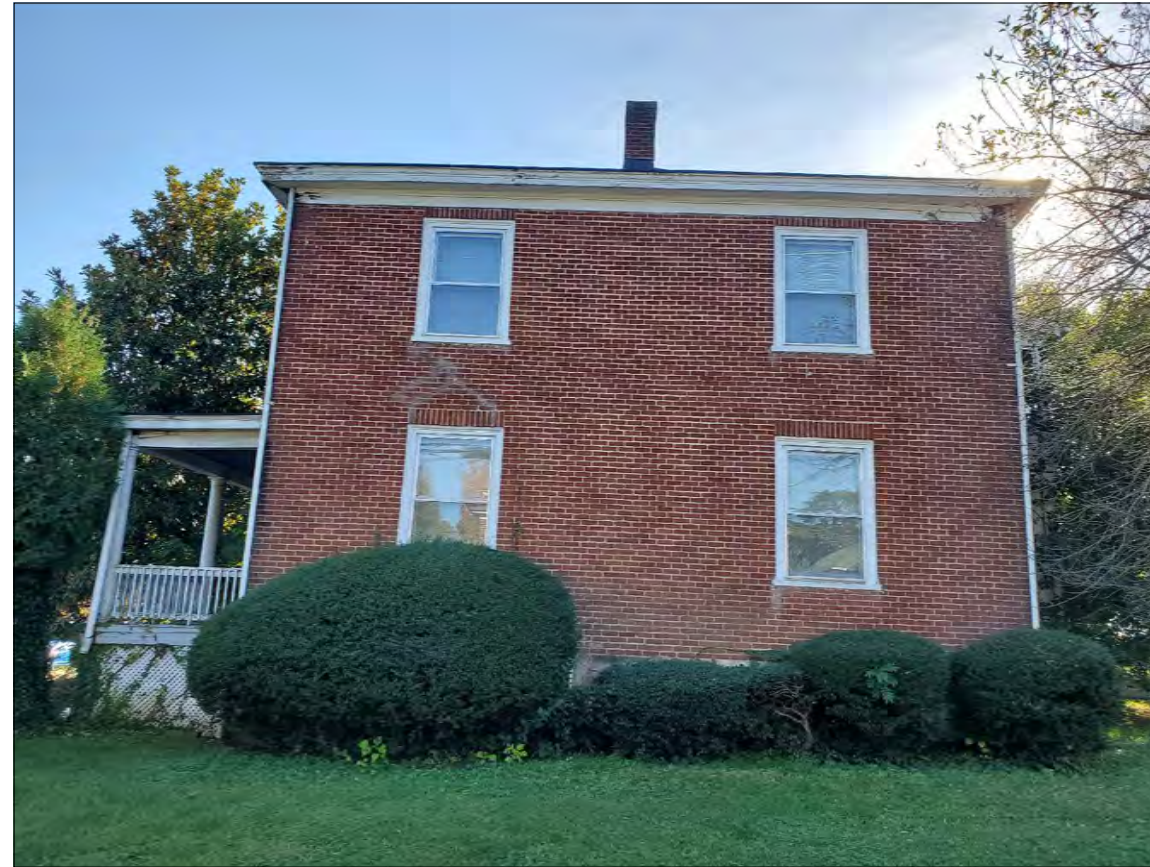
SIDE OF RESIDENCE FROM GORDON AVENUE
