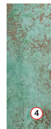
Copper (vertical seam panels -- treated to produce a verdigris patina)
