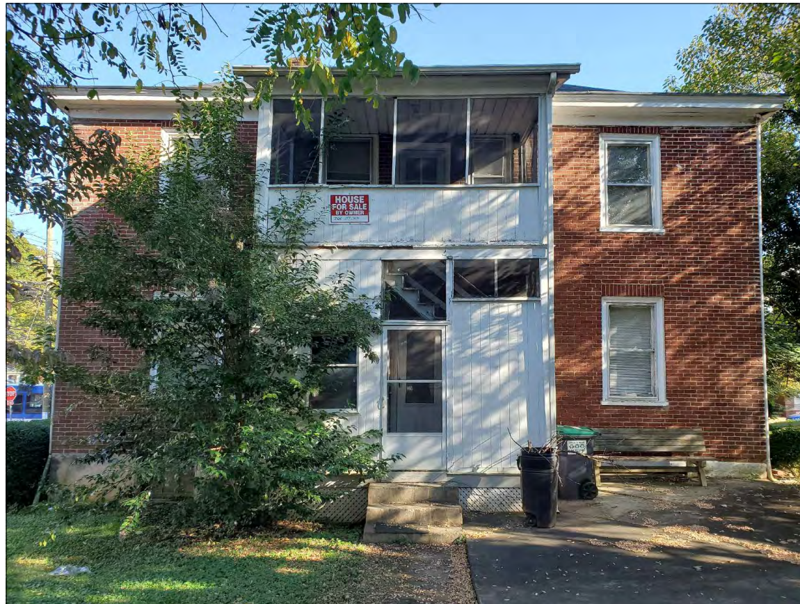
REAR OF RESIDENCE FROM ALLEY
