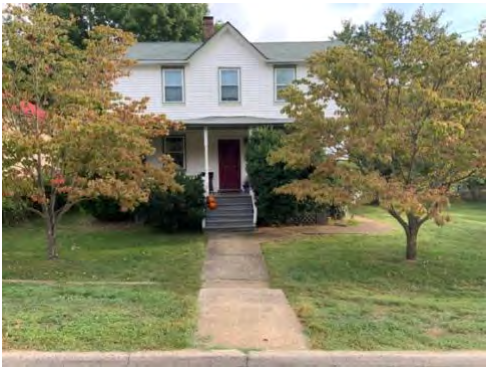
Western contiguous house, 1615 East Market Street
