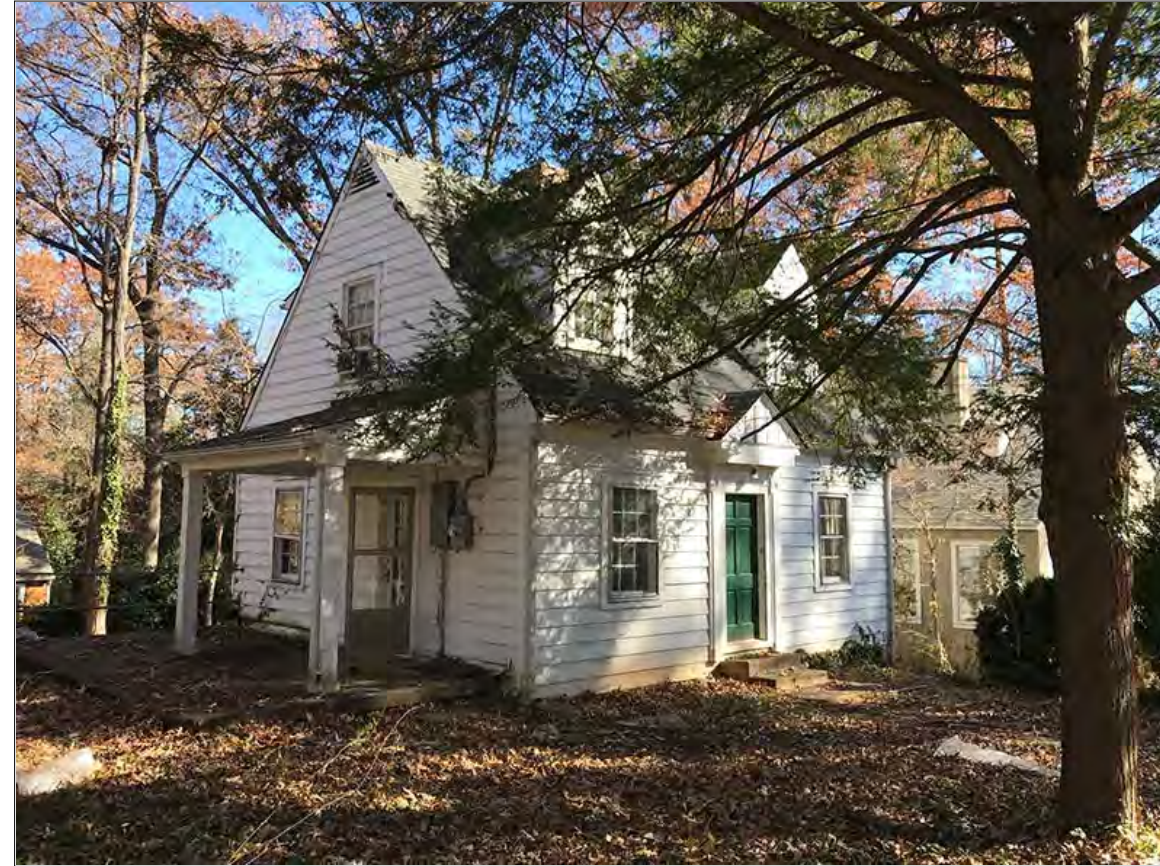
VIEW OF WEST CORNER
