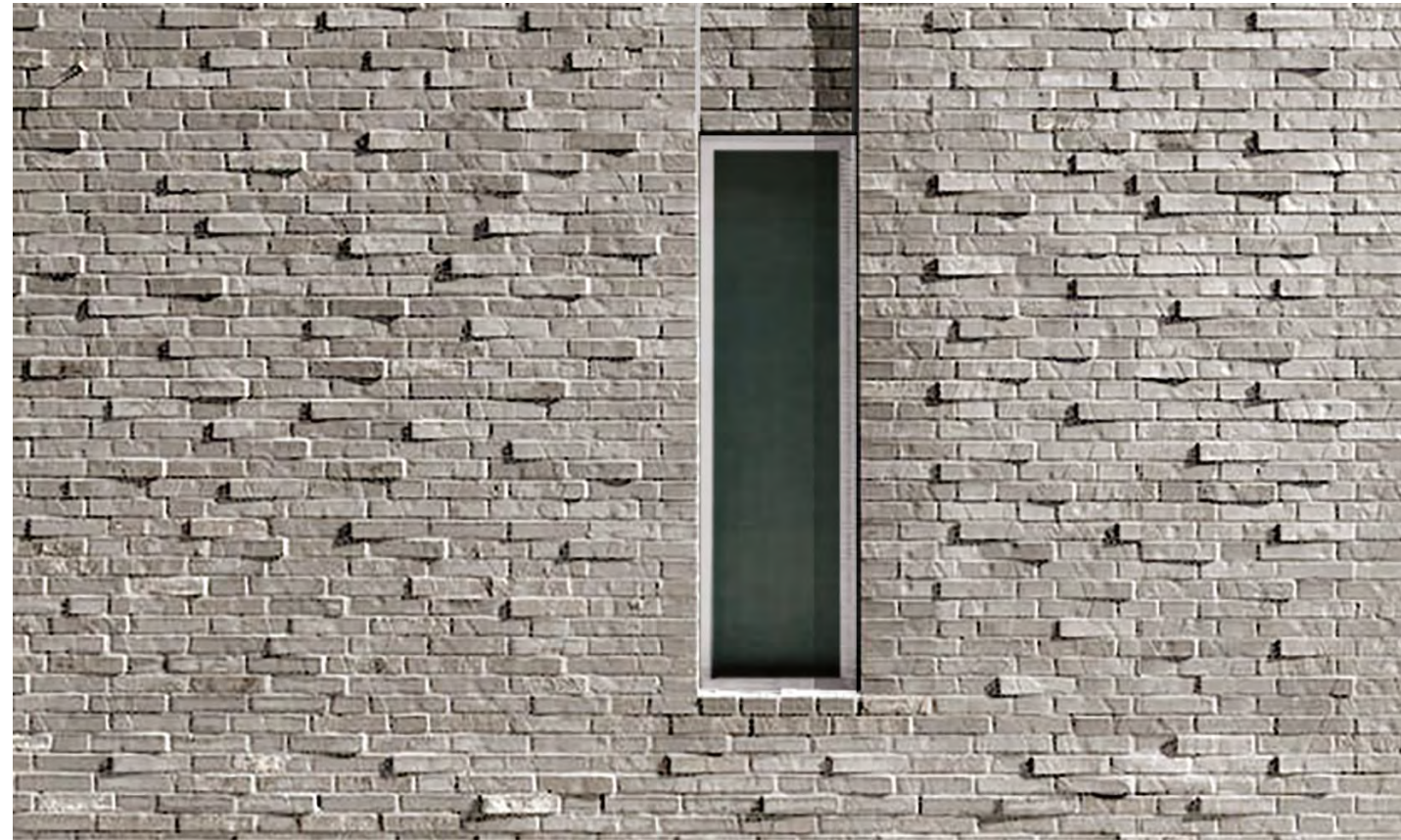
SELECTED TEXTURE FOR HYPHENS - ANGLED BRICK WITH RAKED JOINTS
