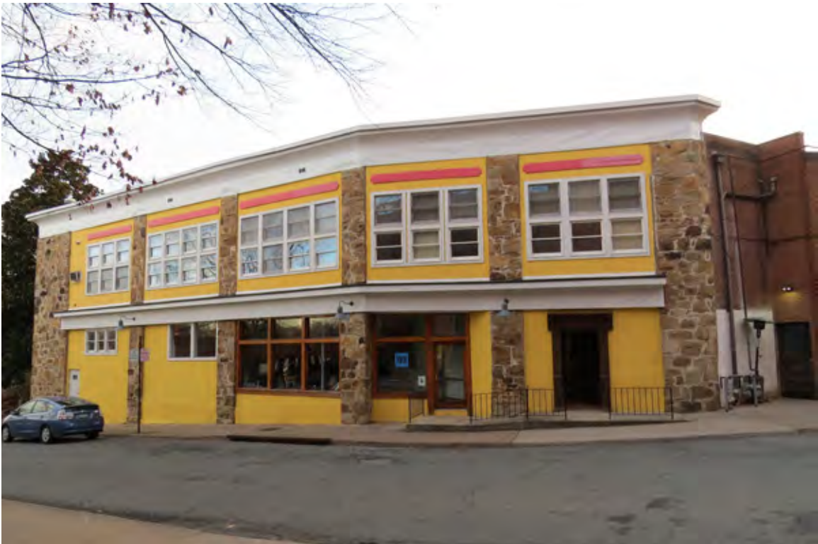
Adjacent structure at southwest corner
