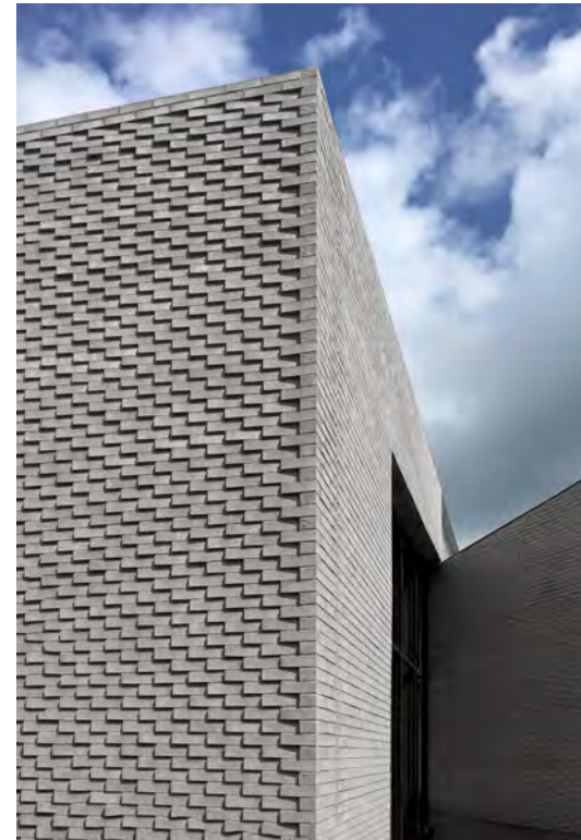
SELECTED TEXTURE FOR HYPHENS - ANGLED BRICK WITH RAKED JOINTS
