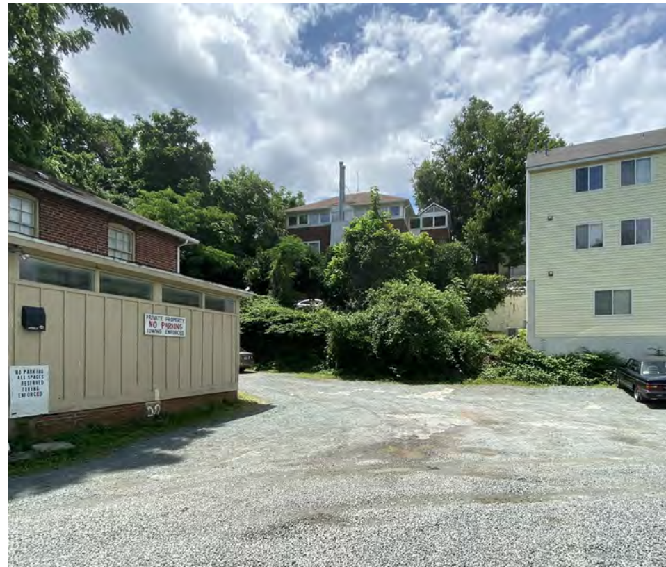
4. 1996 ADDITION EAST (ELLIEWOOD AVENUE)
