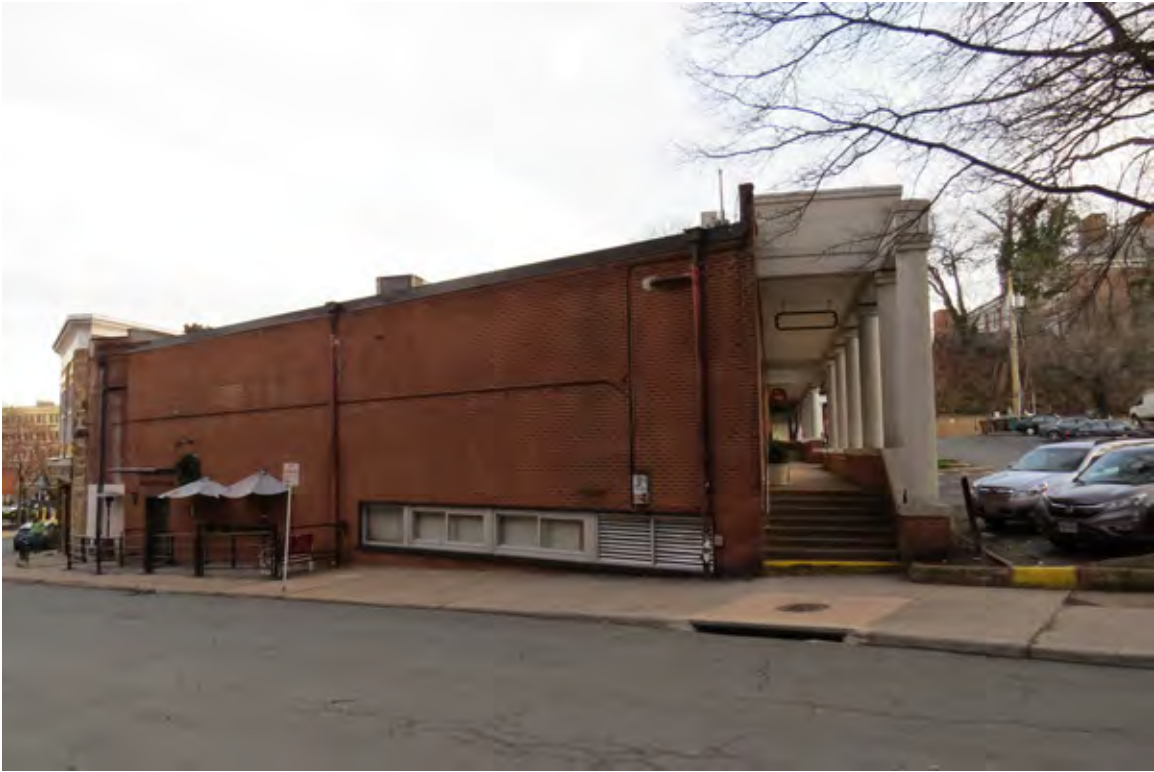
South façade, added after the original construction.
