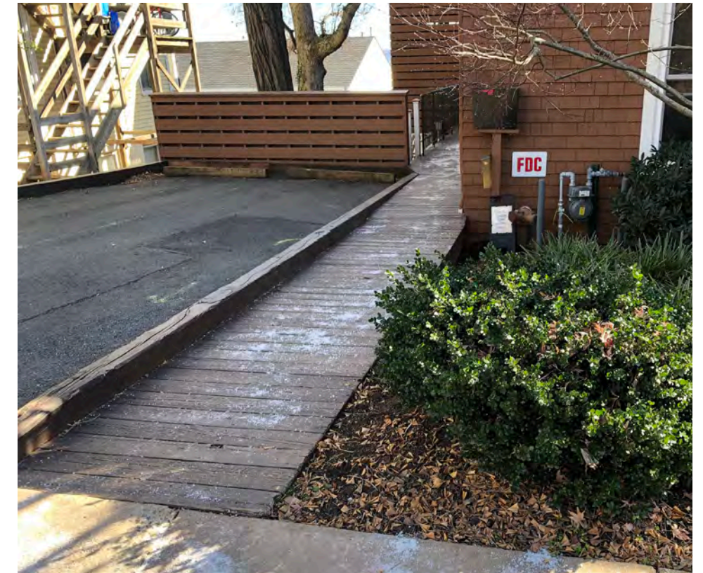
5. EXISTING PARKING AND WALKWAY
