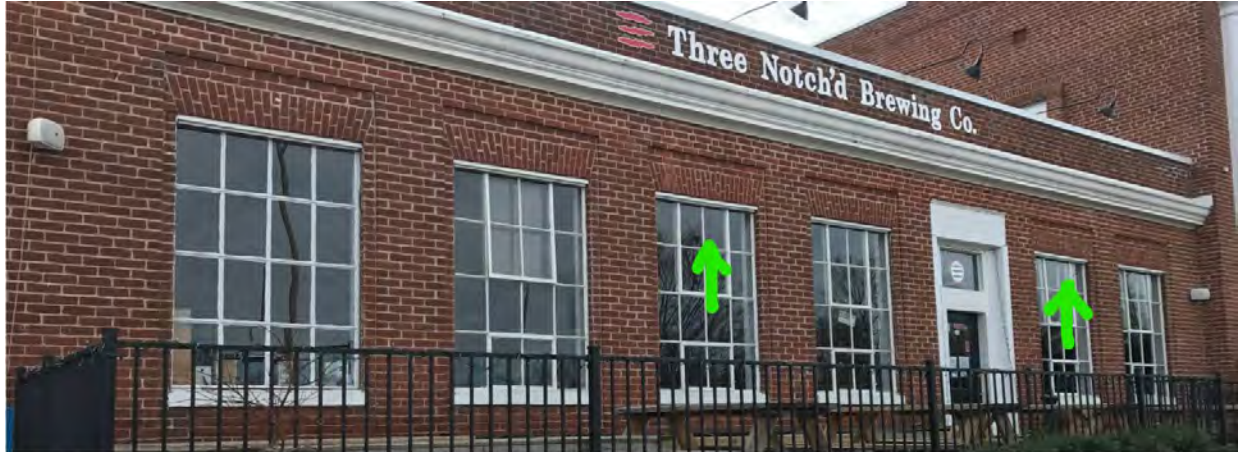
EXISTING CONDITIONS, NORTH ELEVATION AT GRADY AVENUE
