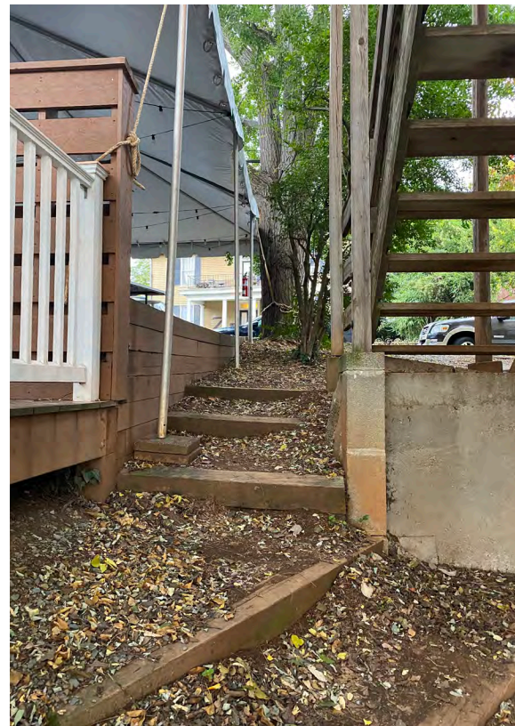
3. EXISTING NORTH TIMBER STAIRS
