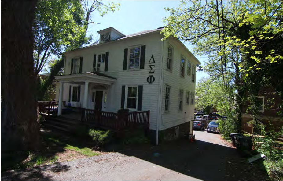
Driveway facing South-West
