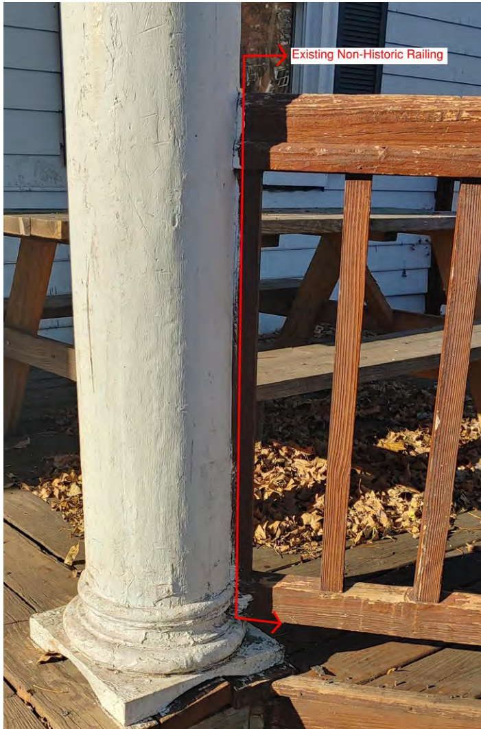
Existing Historic Column Base
