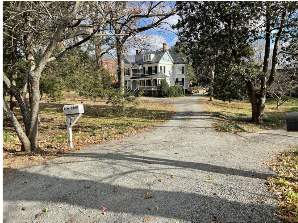
616 Park Street - Southwest View
