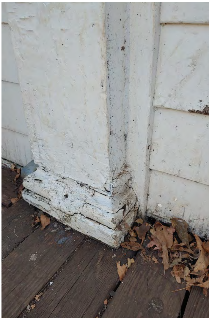
Existing Historic Front Porch Pilaster Base
