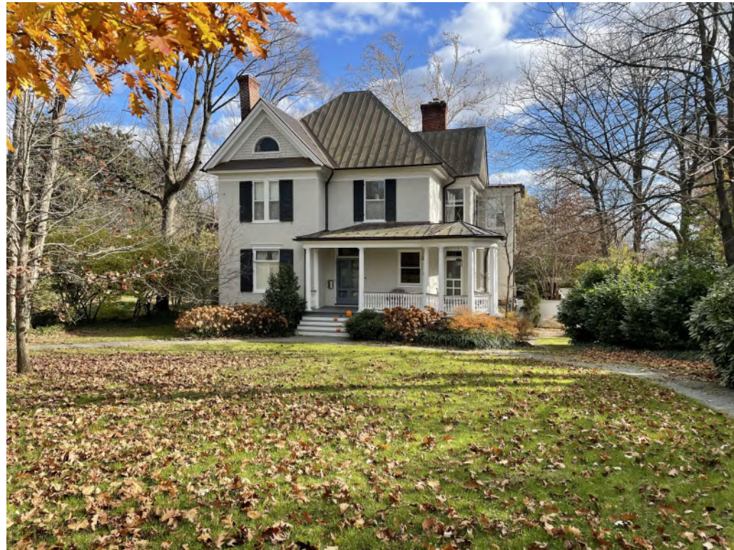
West Elevation - Park Street
