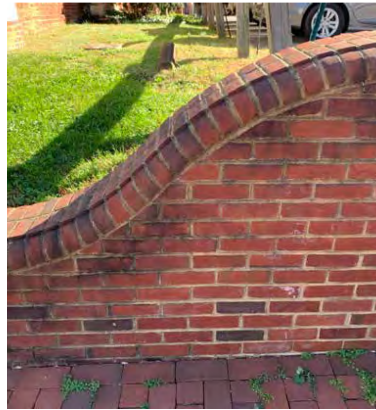
BRICK WALL - SITE PRECEDENT
