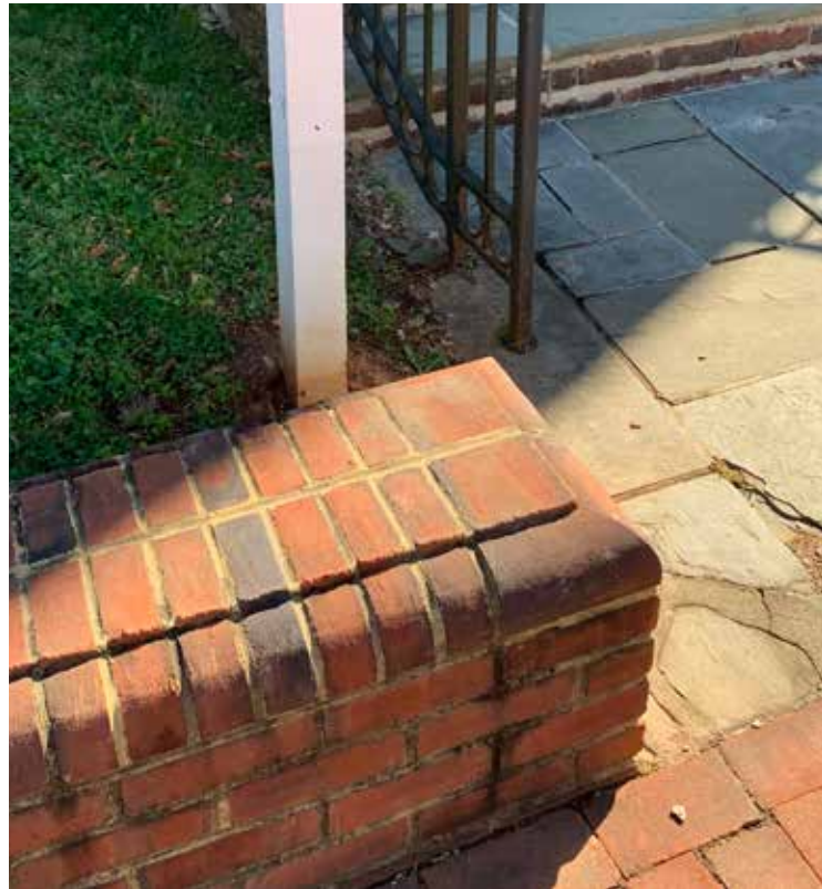
BRICK WALL - SITE PRECEDENT
