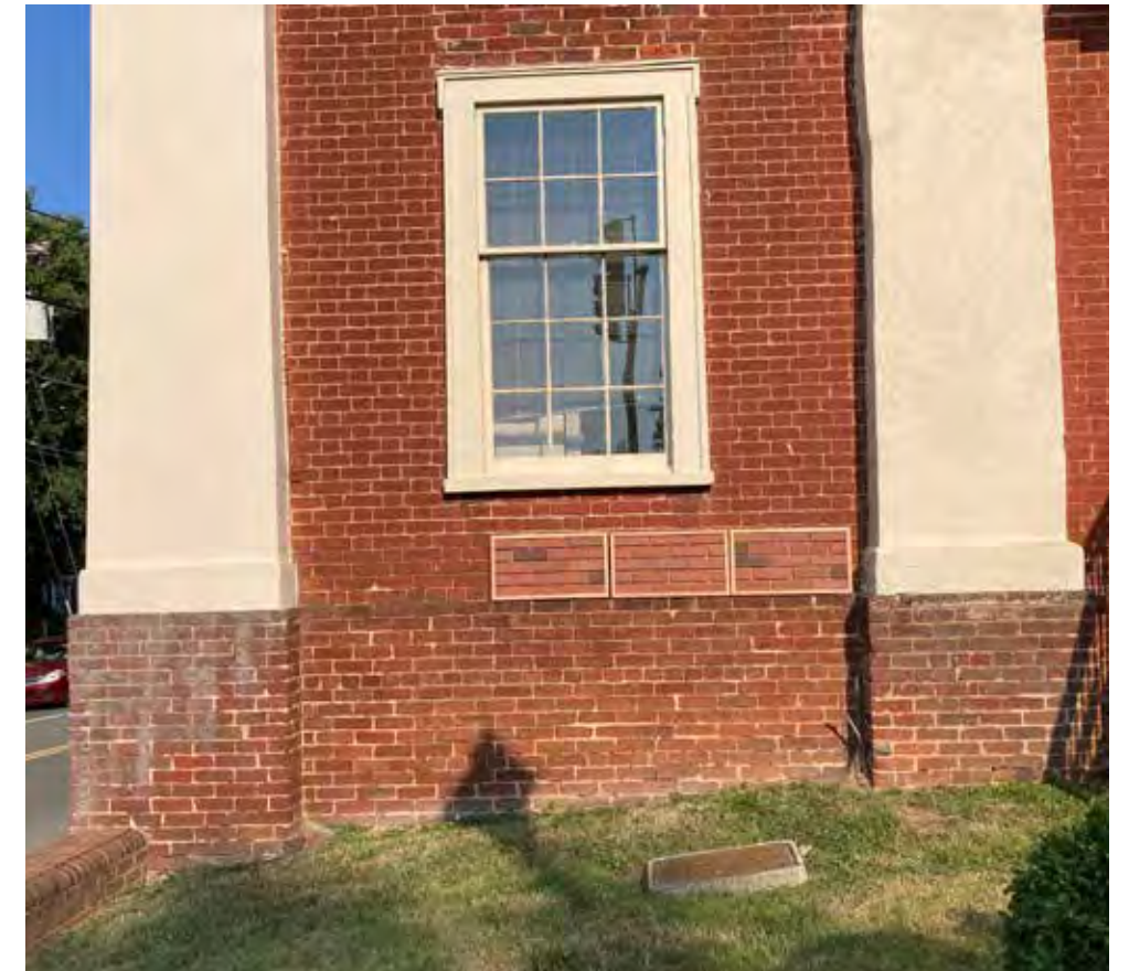
BRICK SAMPLE BOARD OPTIONS AT LEVY FACADE
