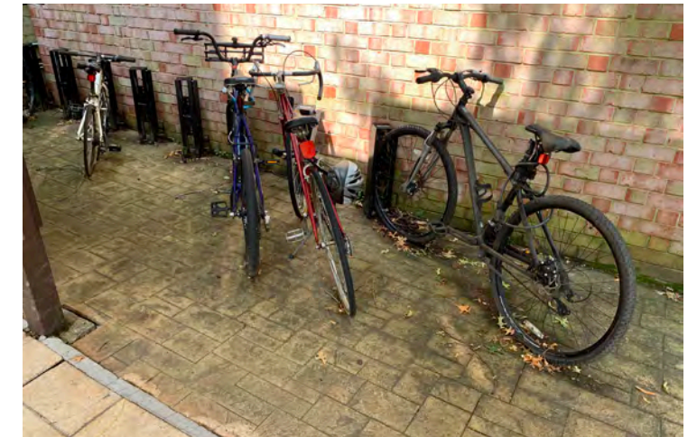
CERAMIC TILES ARE SLIP HAZARDS; BEVELED EDGES ARE NOT ADA-COMPLIANT; PAVING AT BASE OF CANOPY POST FAILING
