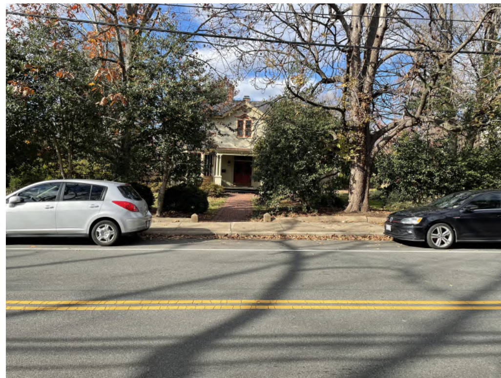
611 Park Street - East/ Park St
