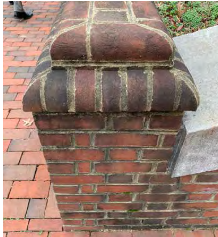
BRICK WALL - SITE PRECEDENT
