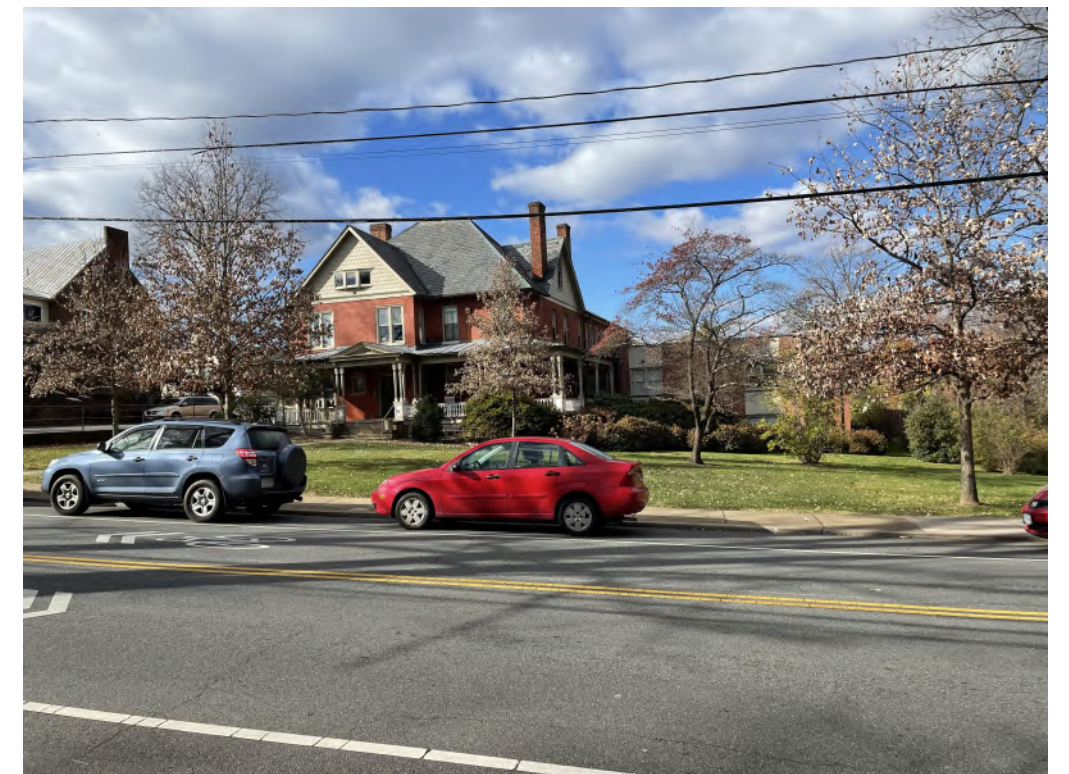
601 Park Street - East/ Park St
