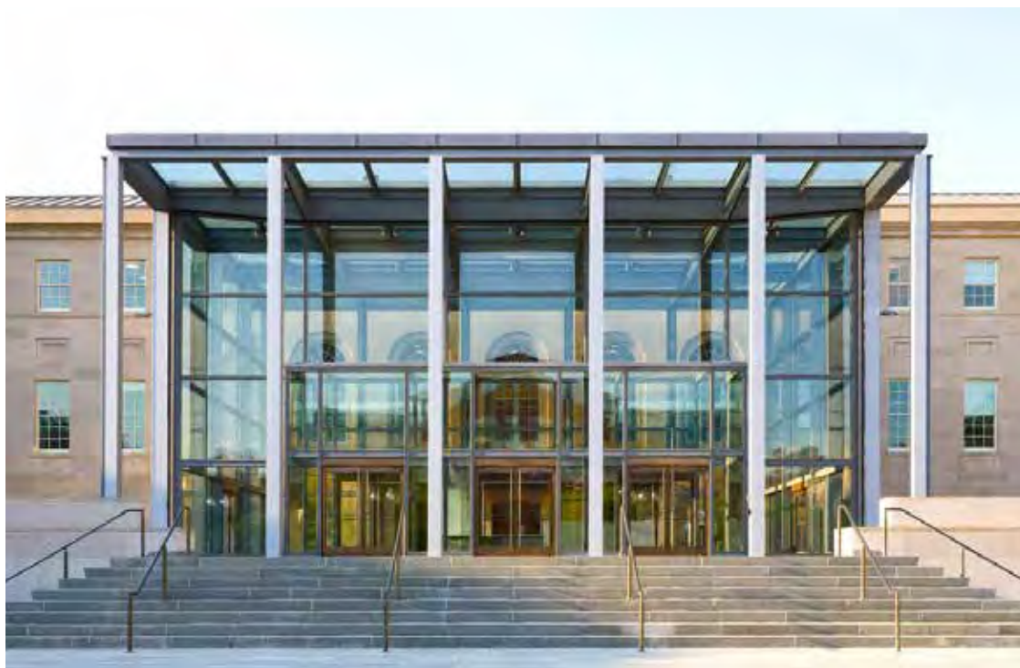
DC COURTHOUSE - WASHINGTON, DC
