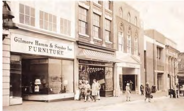
EAST MAIN FACADE, C. 1974
