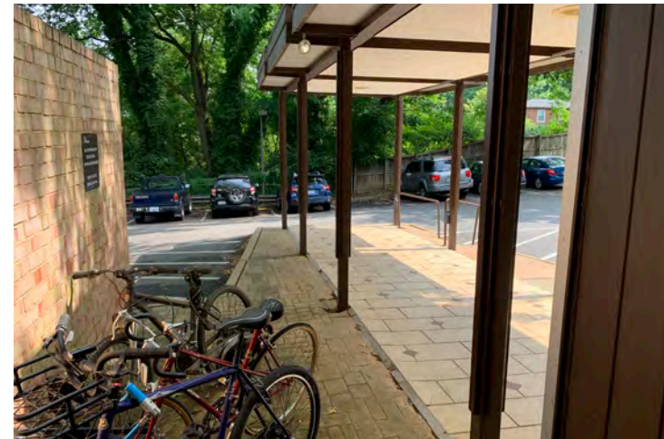
SPACE OF PASSAGE OF BIKES IS TIGHT
