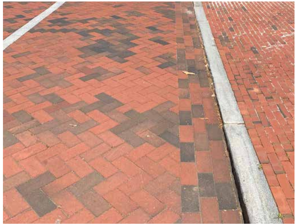
PAVING AT SITE, PARK ST
