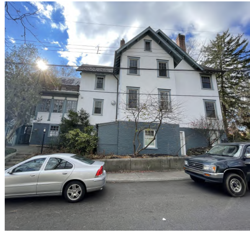
534 Park Street - North/ Farish St
