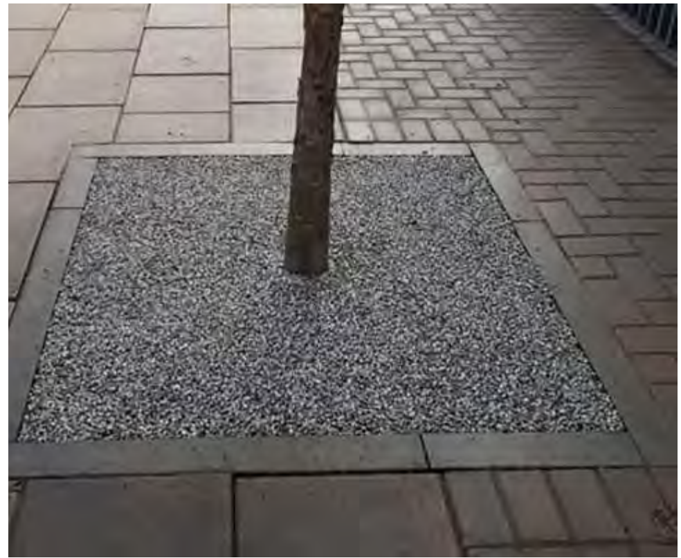
CRUSHED GRAVEL TREE PIT
