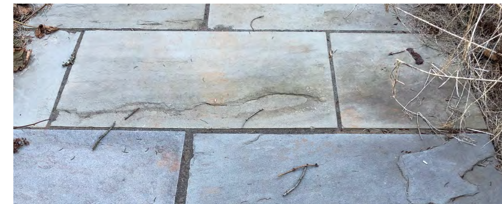
Existing bluestone and stone wall on site
