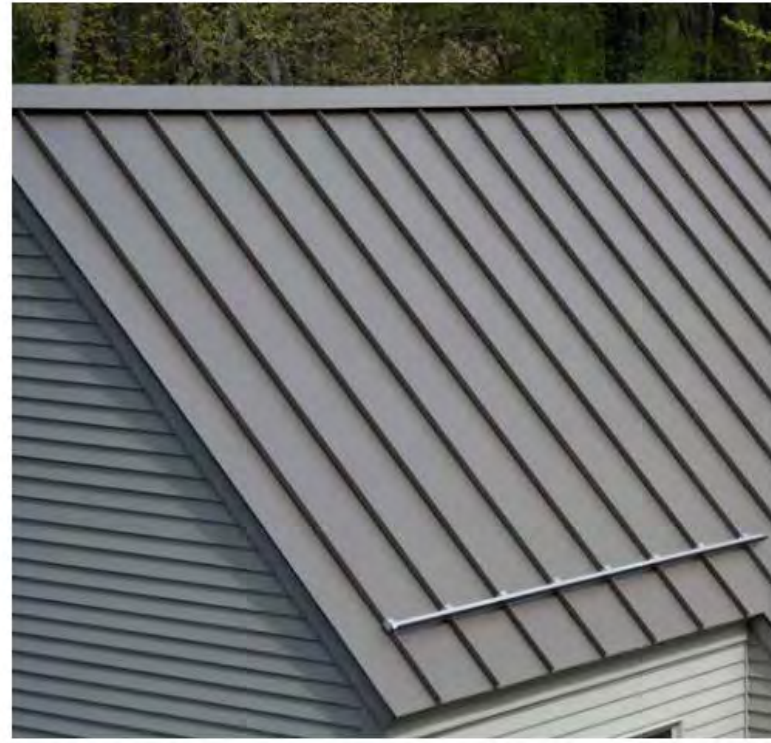
STANDING SEAM ROOF
