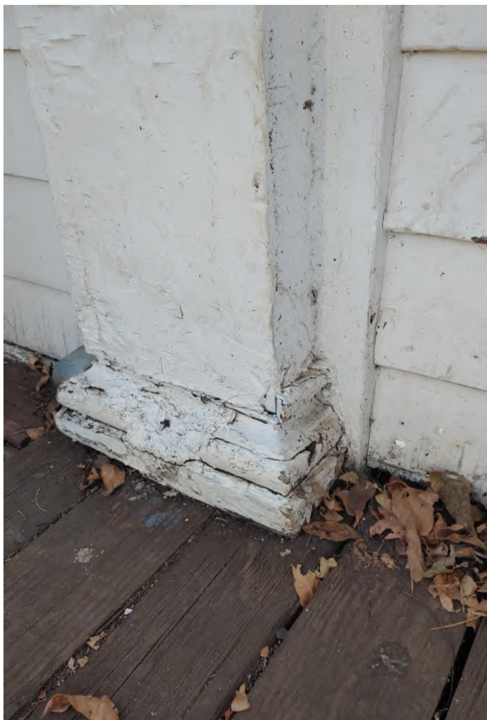
Existing Historic Front Porch Pilaster Base
