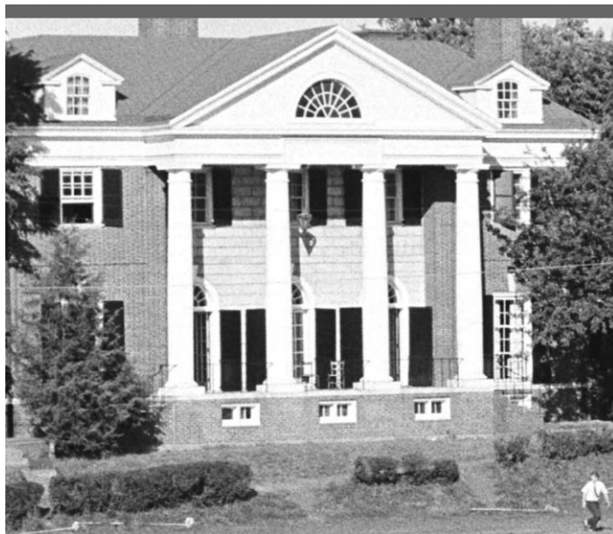
Figure 1: 1965 photo of 159 Madison Lane with view of basement-level windows.
