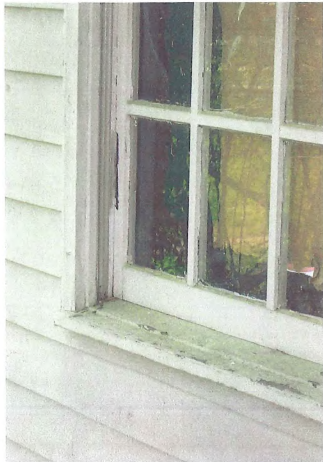
SOUTH "PORCH" WINDOW |
