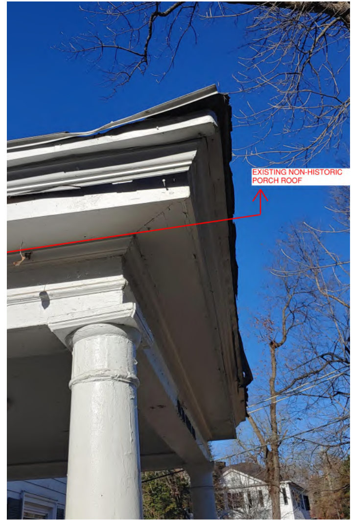
Existing Historic Front Porch Column Capital and Entablature
