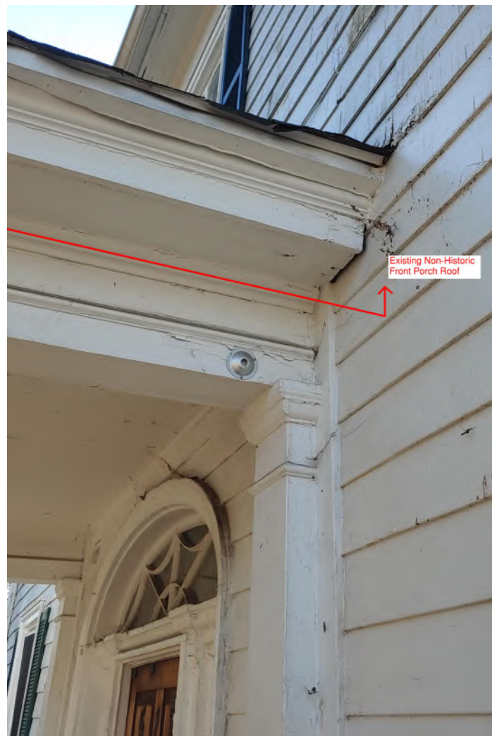
Existing Historic Front Porch Pilaster Capital and Entablature
