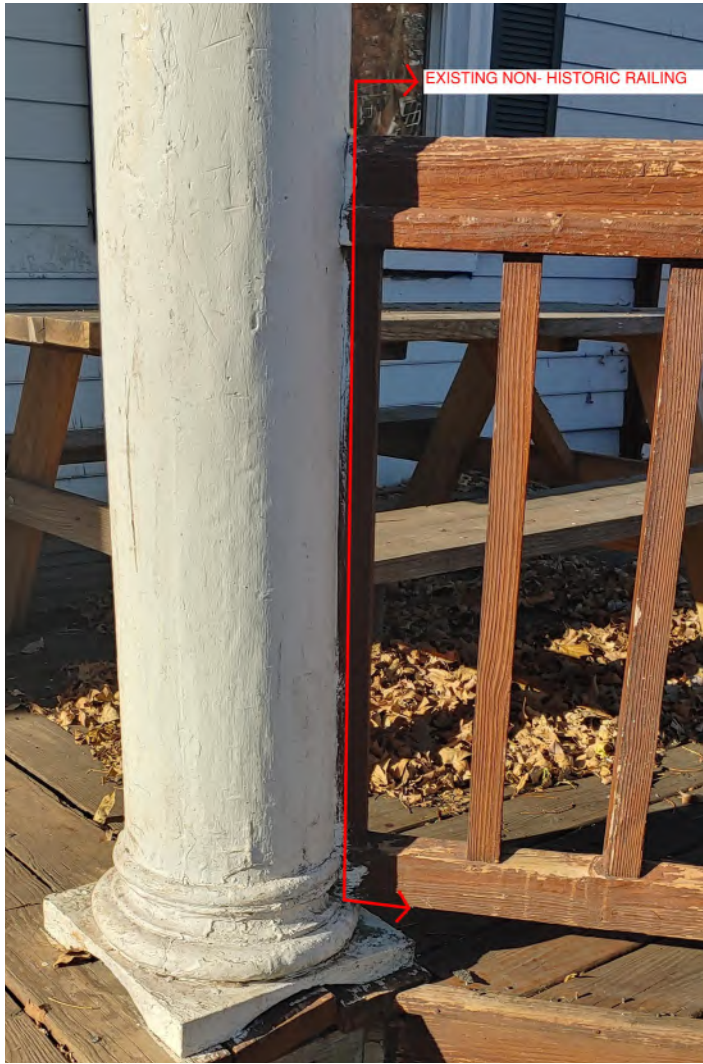
Existing Historic Column Base
