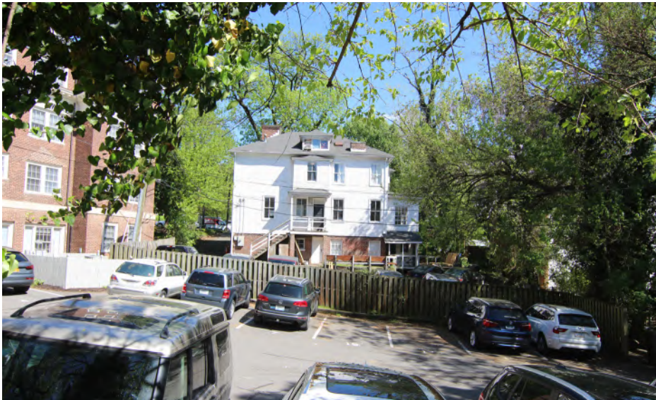
Adjacent Property facing East
