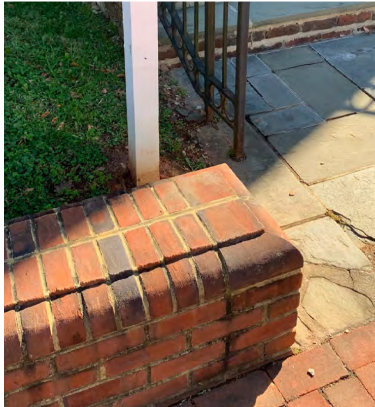
BRICK WALL - SITE PRECEDENT
