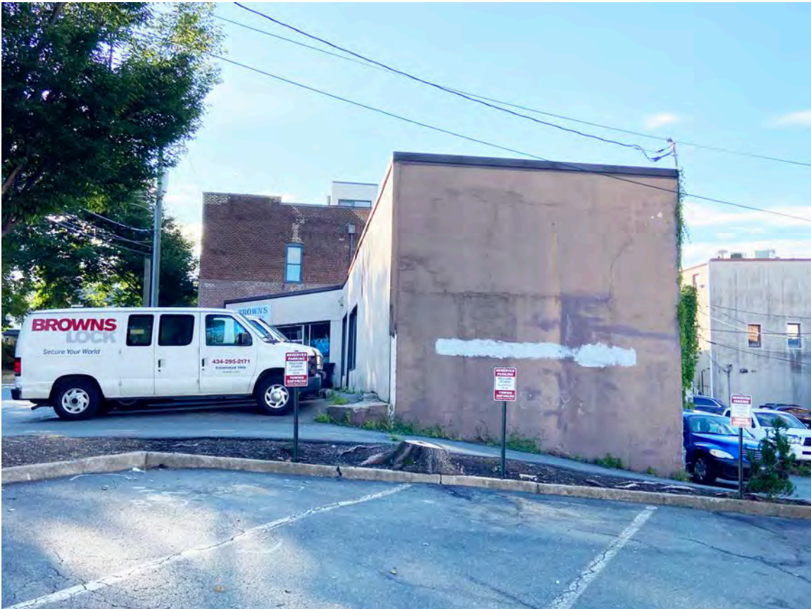
View of west façade from the parking lot of 218 West Market Street
