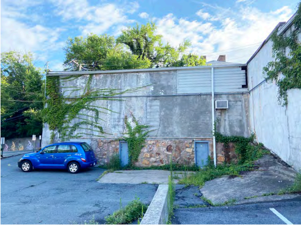
View of western half of the south façade
