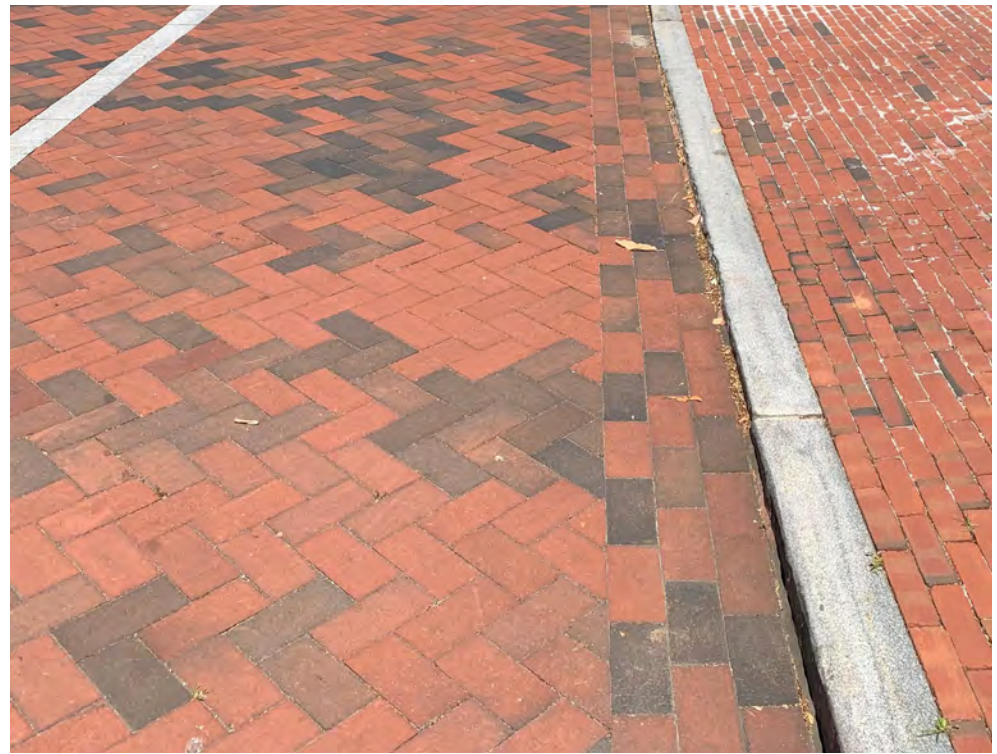
PAVING AT SITE, PARK ST
