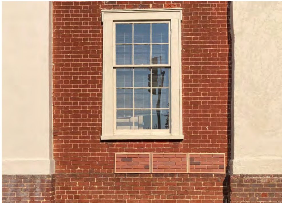
BRICK SAMPLE BOARD OPTIONS AT LEVY FACADE
