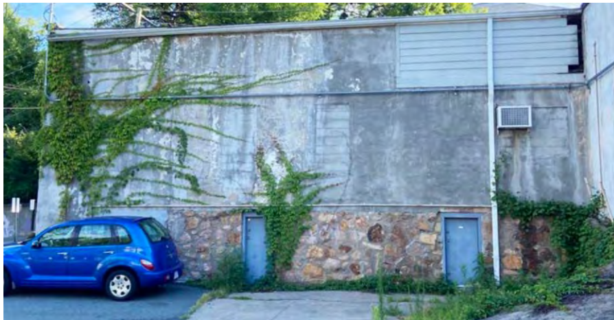
South elevation of 210 West Market Street
