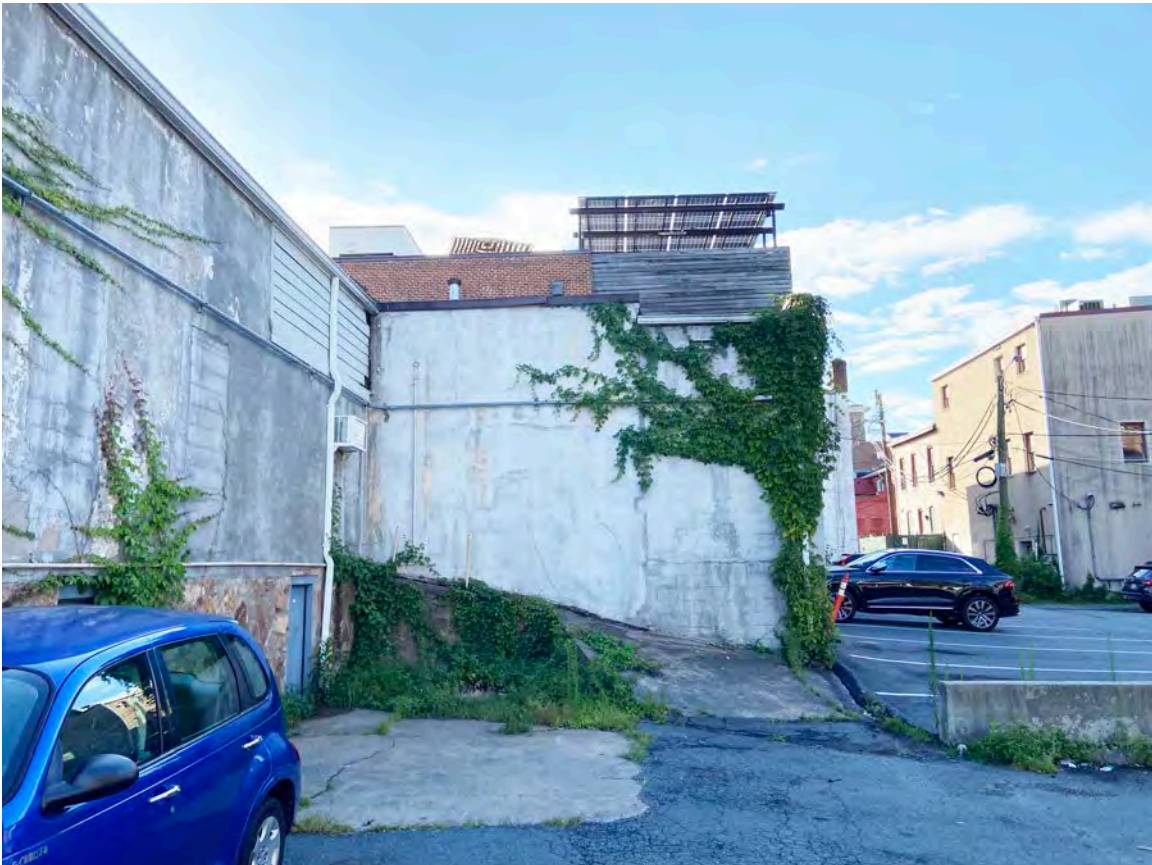
View of south façade looking east
