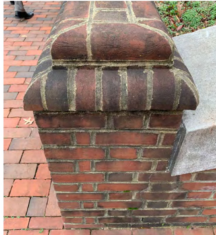
BRICK WALL - SITE PRECEDENT
