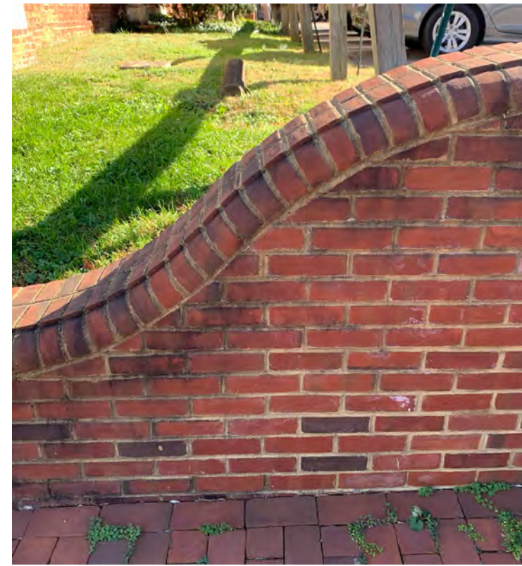
BRICK WALL - SITE PRECEDENT
