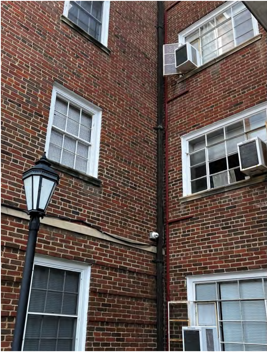
Front bay and wing (north side)
