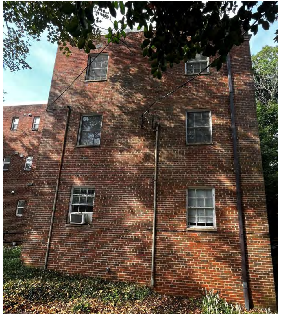
Rear NW wing (north side)
