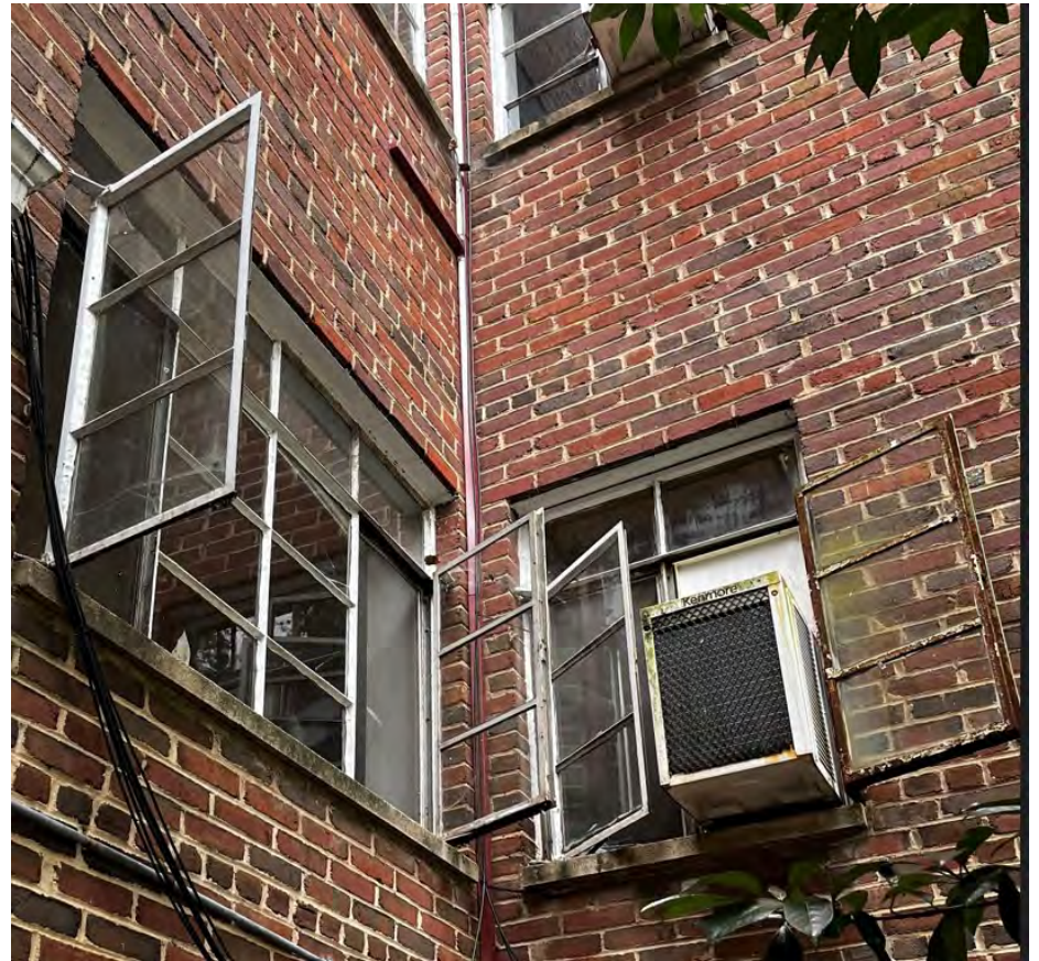
Casements in west bay
