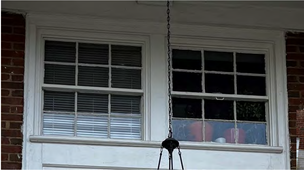
Windows above entry door — front portico (south elevation)
