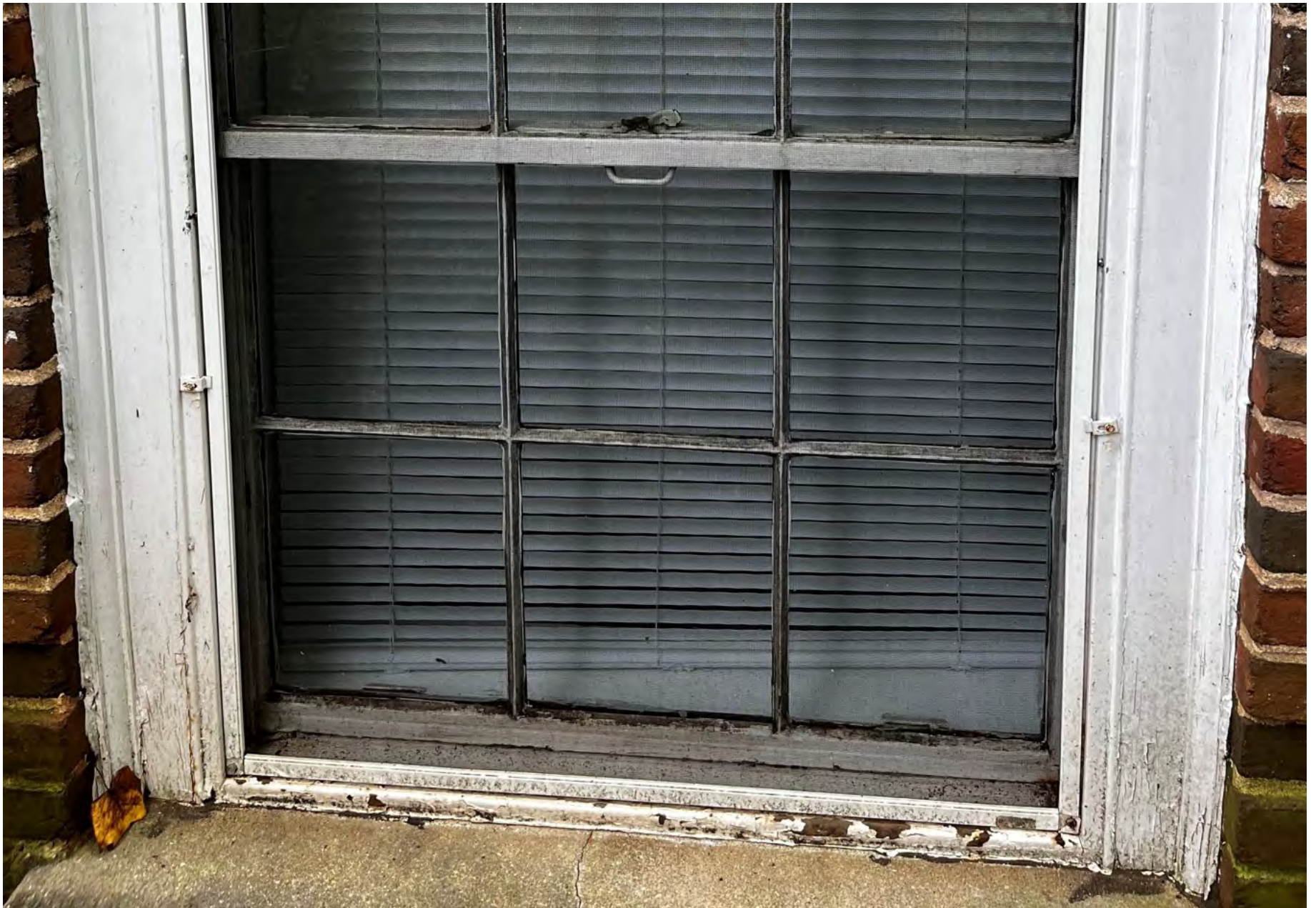
1st Floor window — Front (SW) wing (south elevation)
