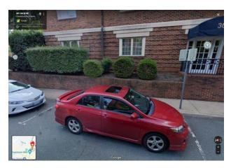
1. Brick retaining walls against sidewalk to reduce height of foundation (Queen Charlotte)
