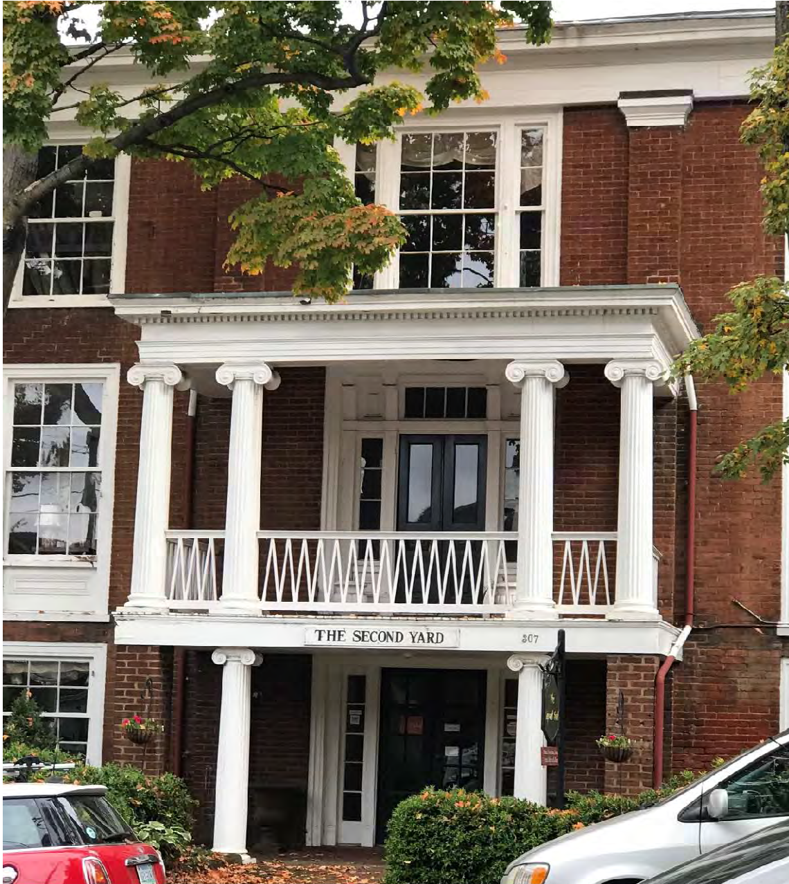
PHOTO 18 - SCISSOR RAILING TO BE USED ON PORTICO – THE SECOND YARD ON MARKET STREET
