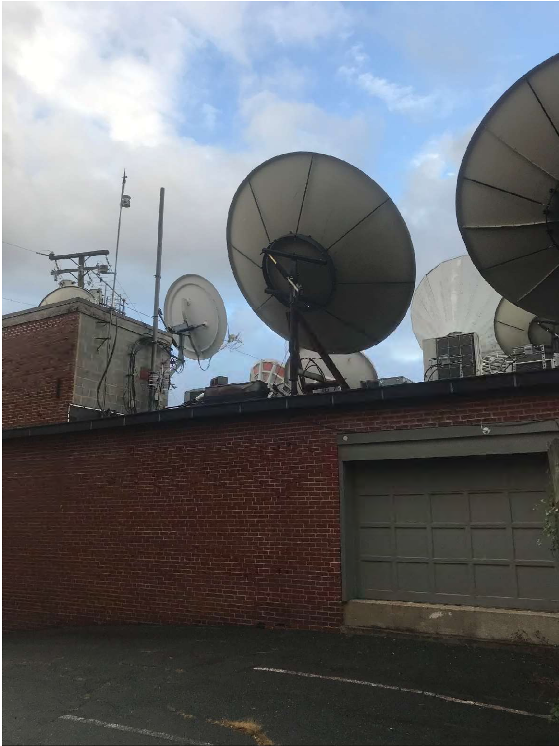
PHOTO 28 - VIEW OF SATELLITE DISHES FROM COURTYARD – TERRACE ESSENTIAL TO BLOCK THESE EYESORES
