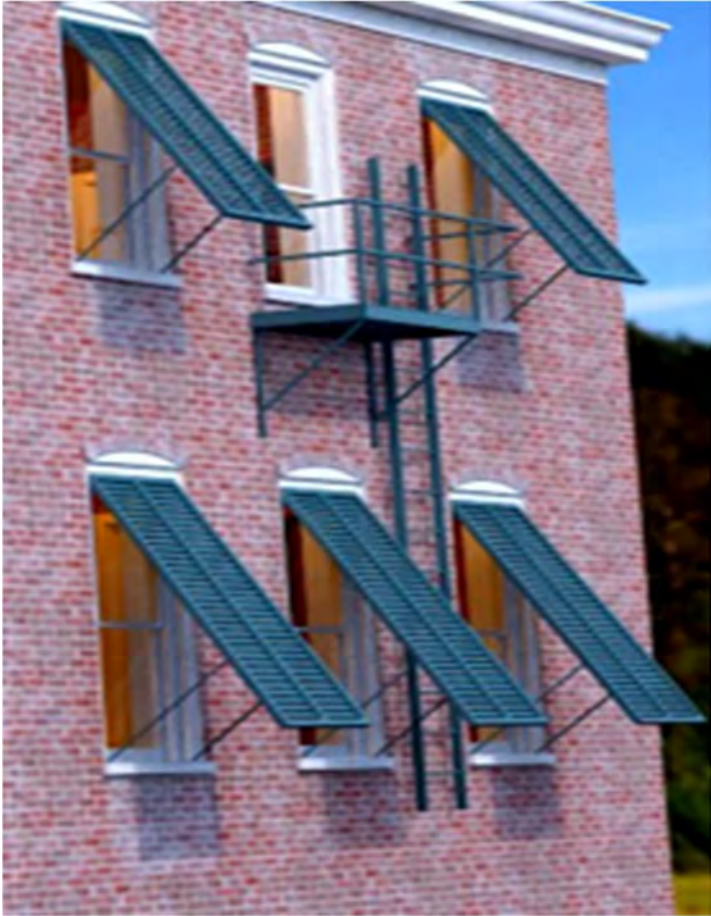
PHOTO 30 - BERMUDA SHUTTERS ON BACK OF BUILDING – NECESSARY TO BLOCK VIEWS OF SATELLITE DISHES
