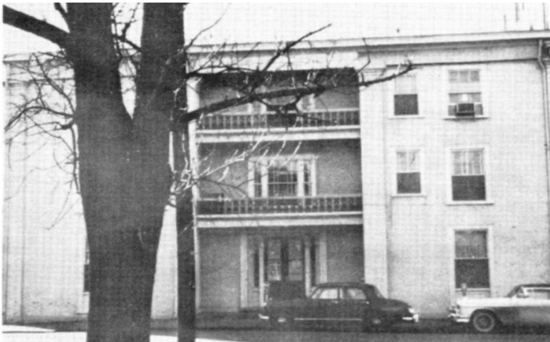
PHOTO 2A & 2B – HISTORIC PHOTOS OF BUILDING EXTERIOR HAVING BEEN PAINTED WHITE
