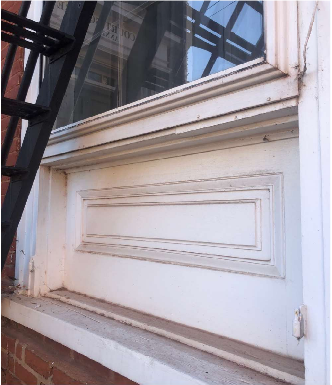
PHOTO 12 A – ORIGINAL SHUTTER PINS
