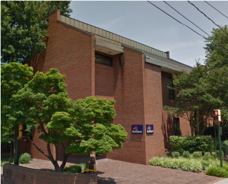
Image 3. Former bank on subject property, to remain (credit: Google)
