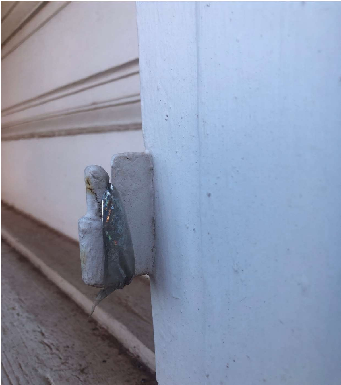
PHOTO 12 B – ORIGINAL SHUTTER PINS
