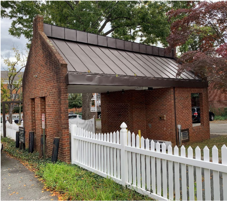
Image 2. Drive-through structure to be demolished
