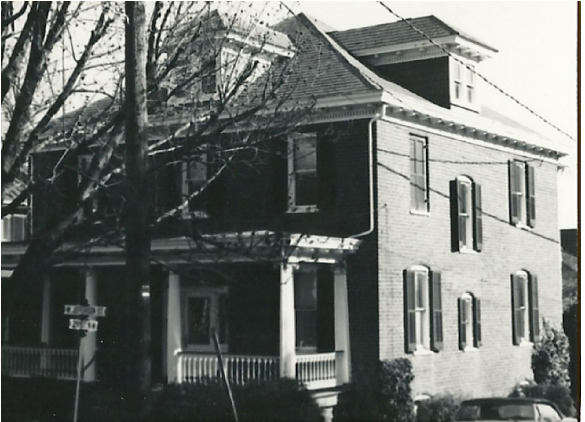
116 West Jefferson Street - Revercomb House c.1913 - Photos from City Historic Survey (1970s -1980s)
