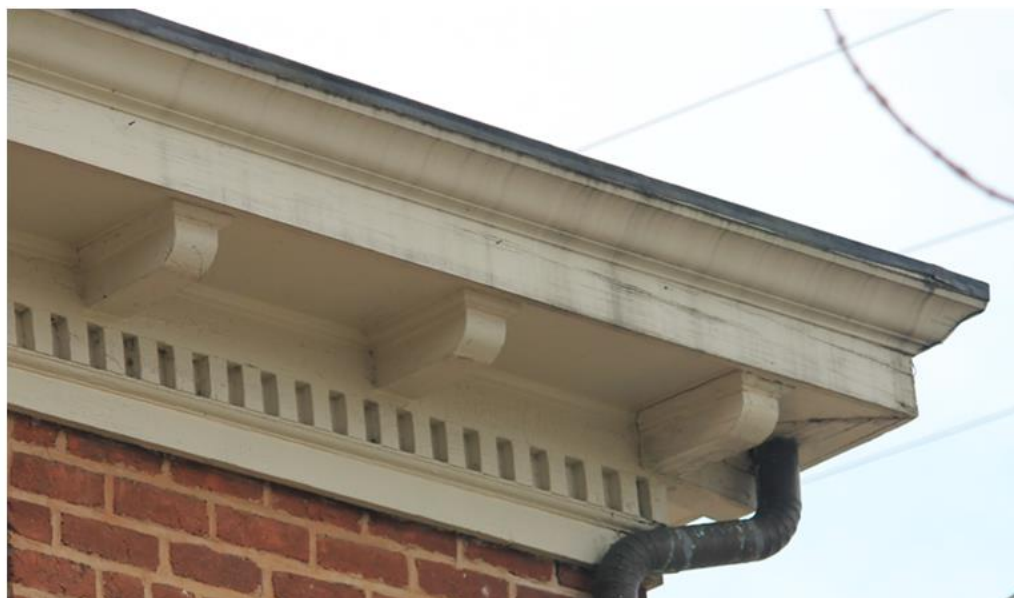
Cornice at 116 West Jefferson St
