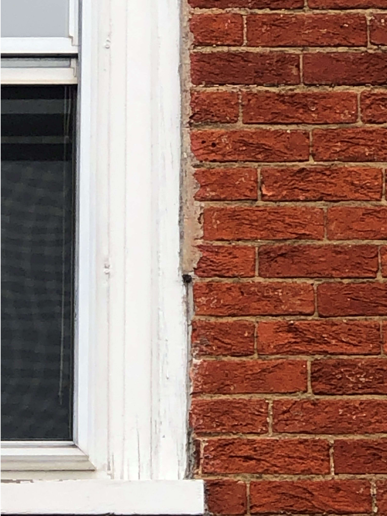
UNORIGINAL WINDOW – NOTE MORTAR AT EDGES
