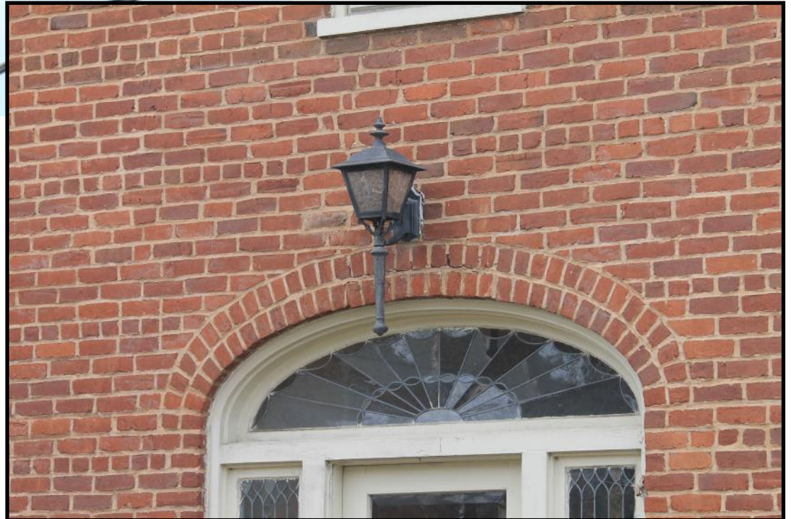
Above Front Door (North Elevation)
