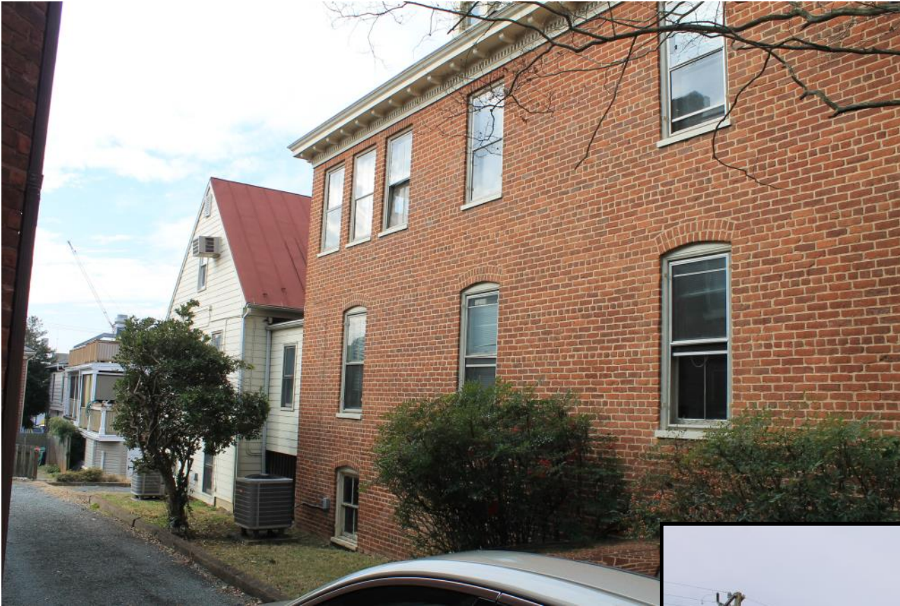
East Elevation—from W. Jefferson
