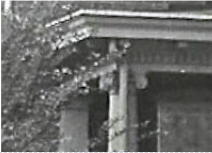
Original porch at 116 West Jefferson
