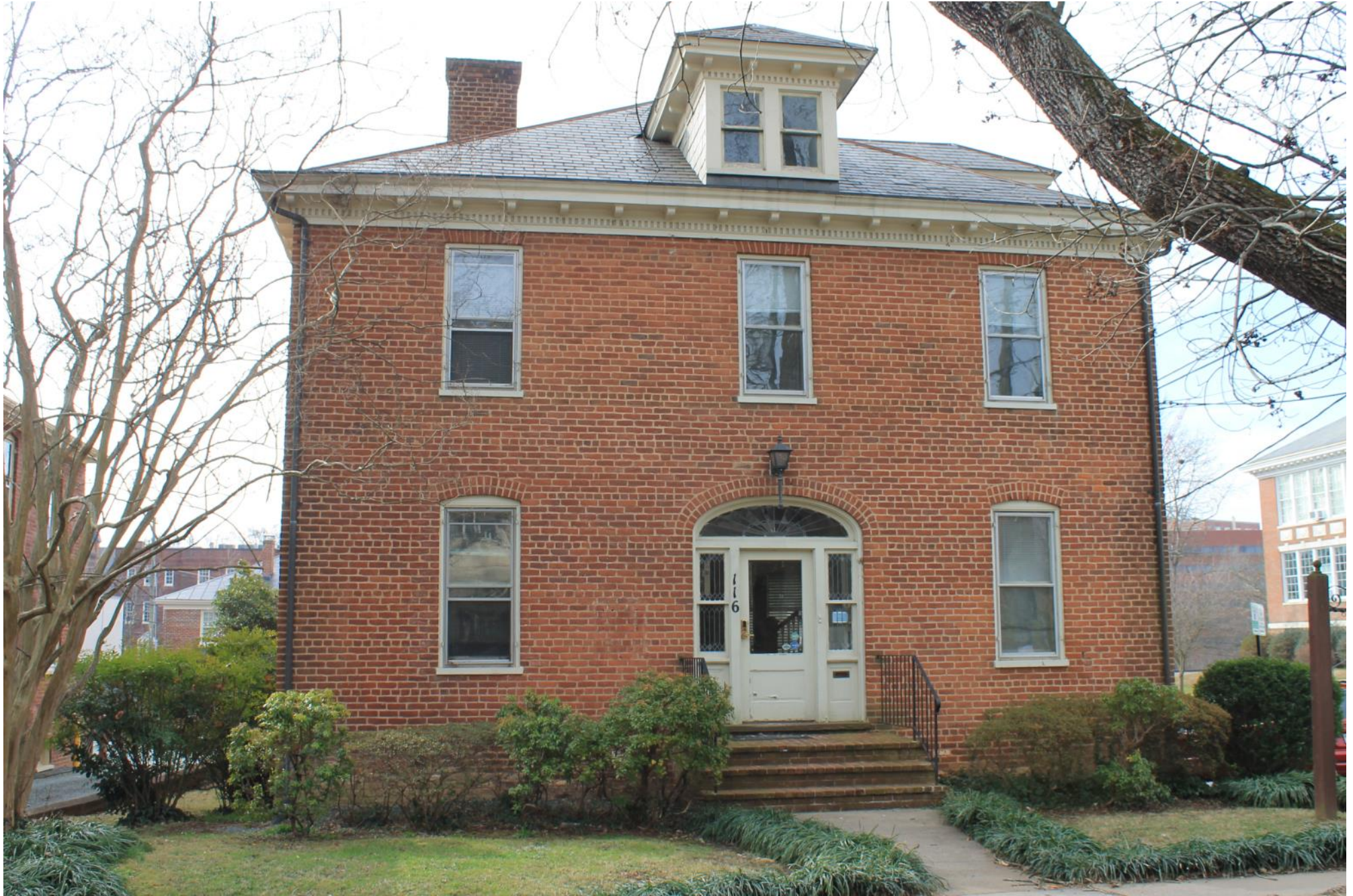
North Elevation—from W. Jefferson
