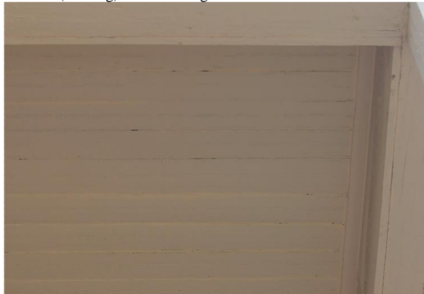
Ceiling at rear porch (upper) - 116 West Jefferson St.
