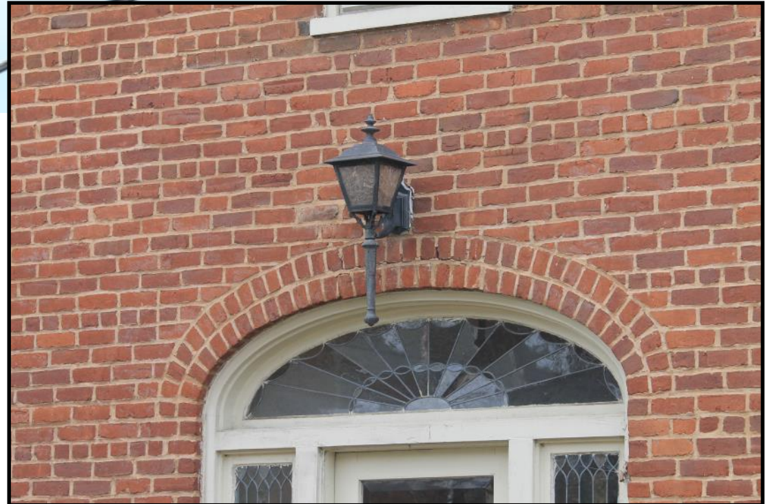
Above Front Door (North Elevation)
