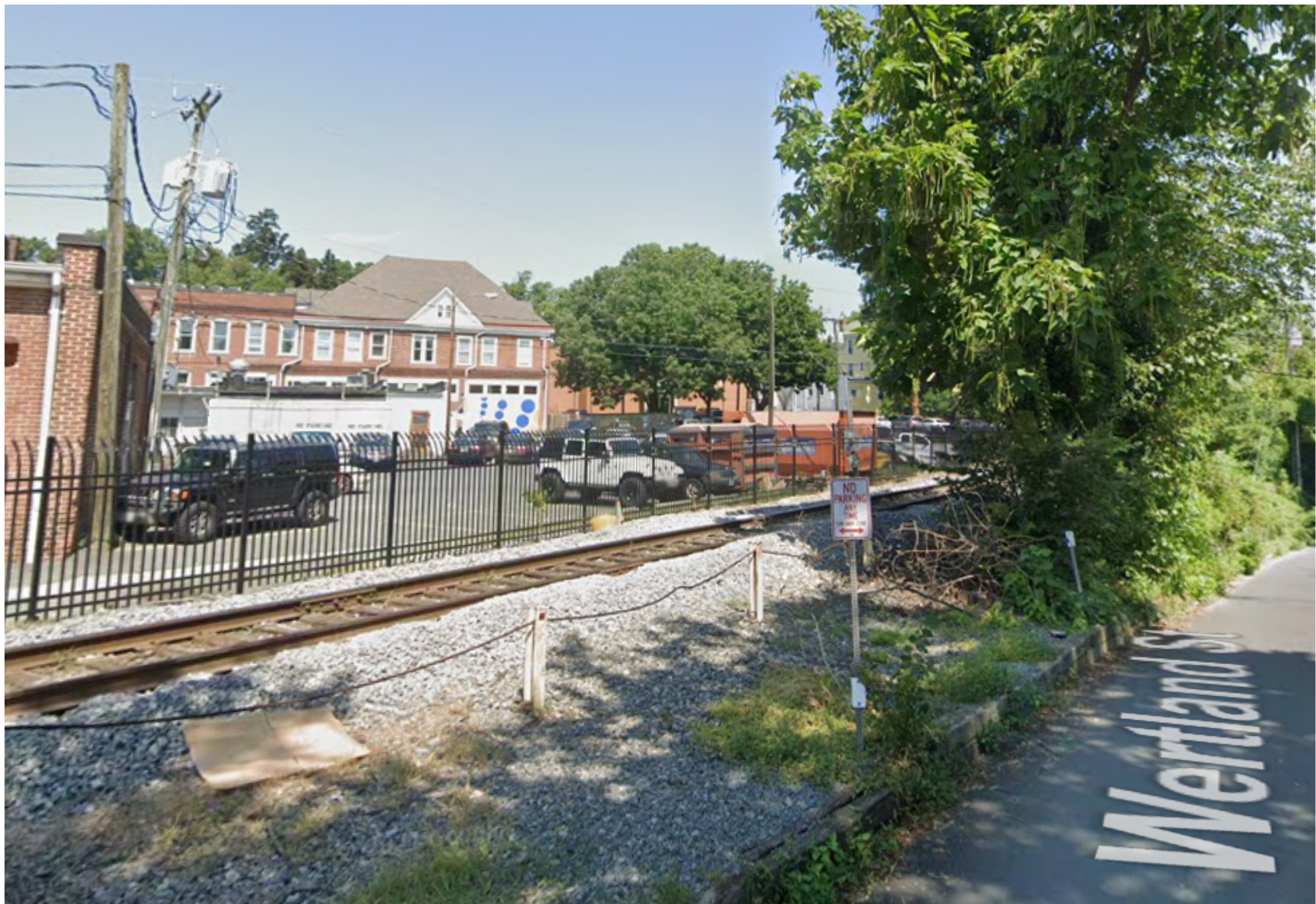
East Elevation - Wertland / 15th Street NW View Note rear portion of building not visible from street
