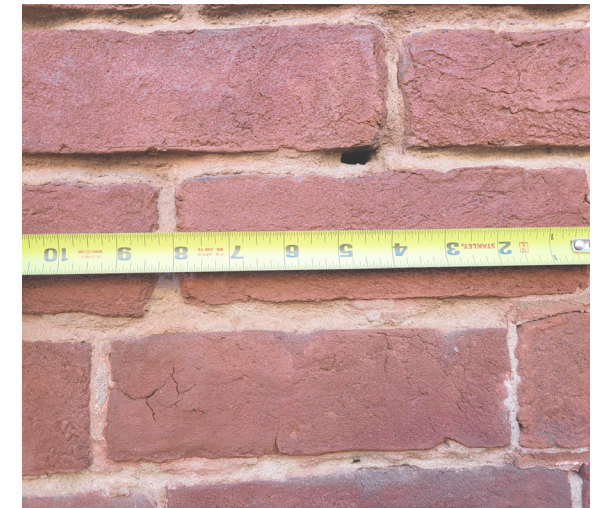
MEASUREMENT OF EXISTING BRICK ON HISTORIC WERTENBAKER HOUSE
