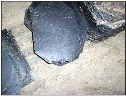
Right: New rubber slate (center; left) next to historic slate (right).
