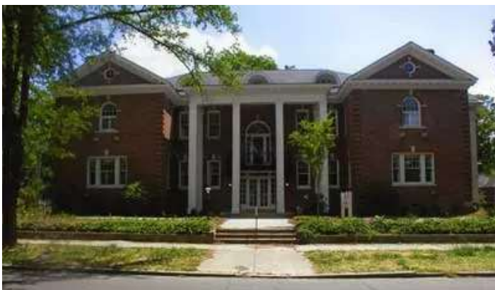
Front of the King's Daughters Home. The solar panels are installed on the facade that faces the street at the right edge of this photograph.
