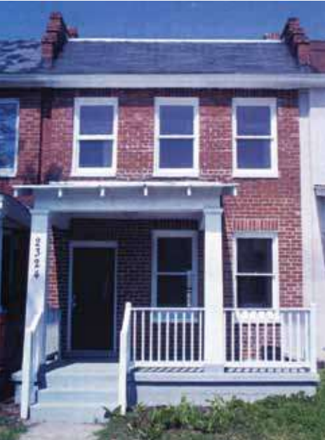
Recommended: [72-73] Solar panels were installed appropriately on the rear portion of the roof on this historic row house that are not visible from the primary elevation.
