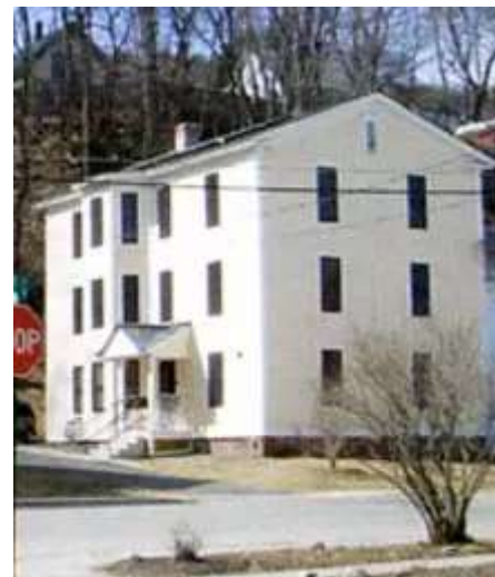
Low-profile solar collectors located on the south side of the gable roof are minimally visible.
