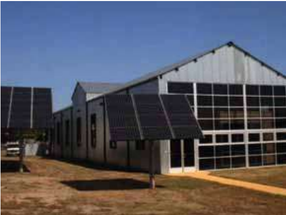
Recommended: [74] Free-standing solar panels have been installed here that are visible but appropriately located at the rear of the property and compatible with the character of this industrial site.
