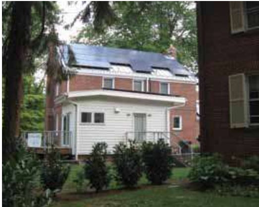
Not Recommended: [75] Solar roof panels have been installed at the rear, but because the house is situated on a corner, they are highly visible and negatively impact the character of the historic property.
