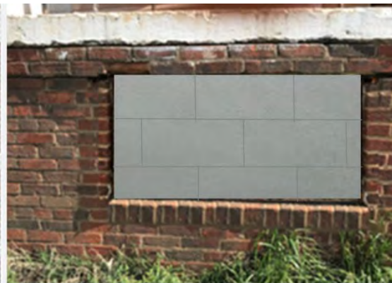
Conceptual - parged, struck lines
