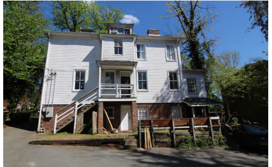
Parking area facing East
