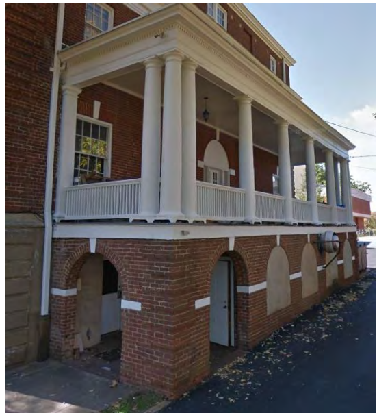
Figure 2: Filled-in arched basement openings at 165 Rugby Road
