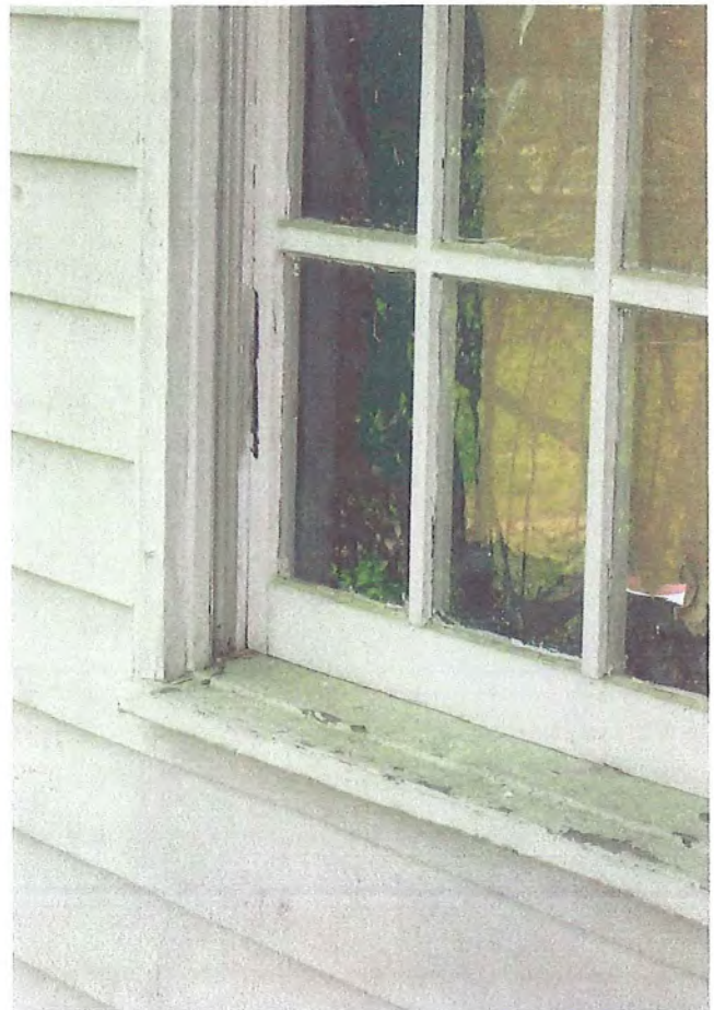
SOUTH "PORCH" WINDOW |
