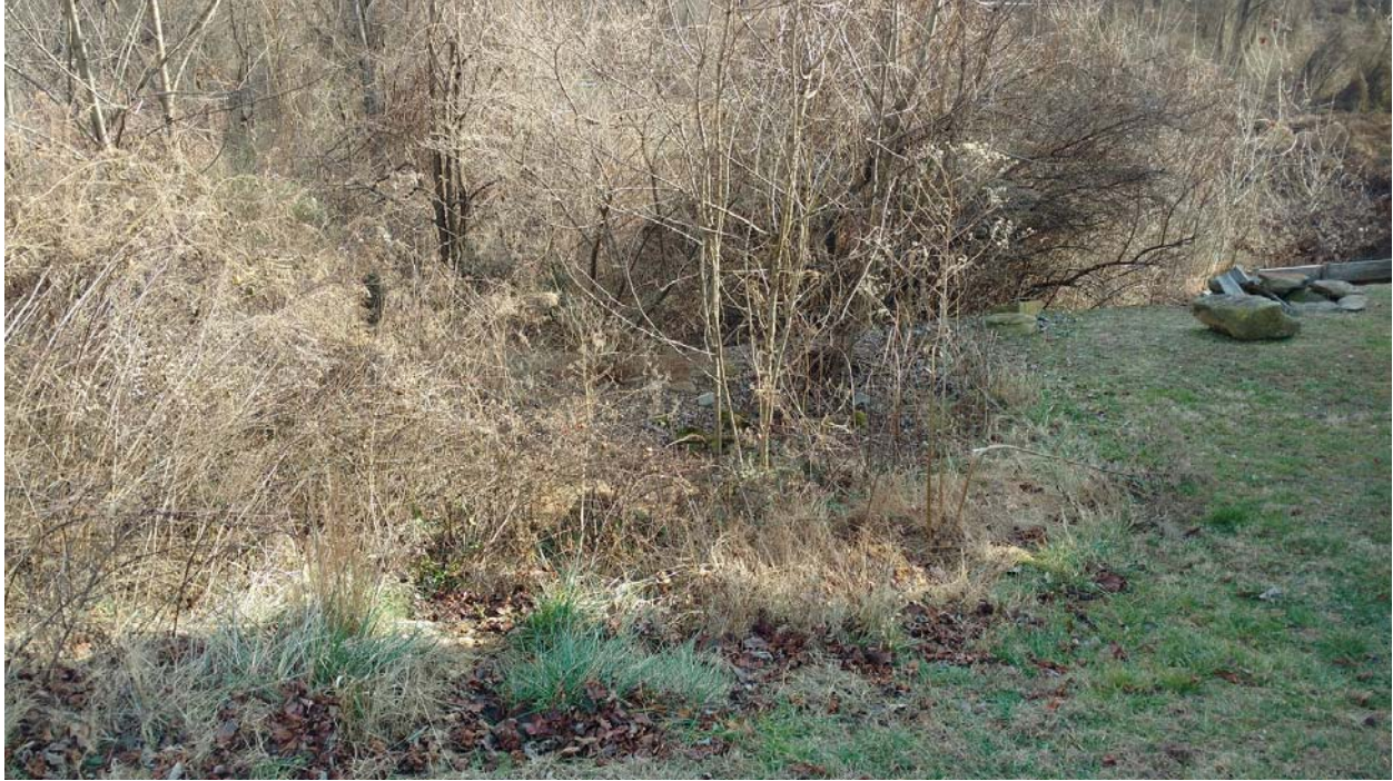
Critical slope area
