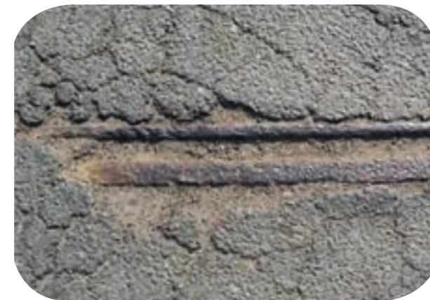
STREETCAR RAIL IN PAVING accompanies panel on streetcars
