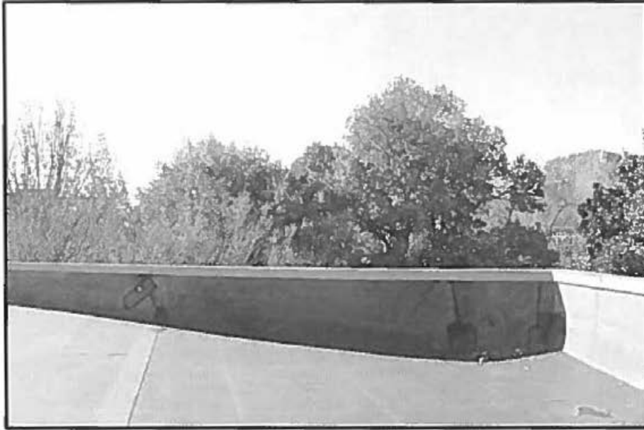
Figure 6. Views from Roof Level of 1521 University Avenue Collocation Site (UVA MC N010), Charlottesville, Virginia, Looking South.
