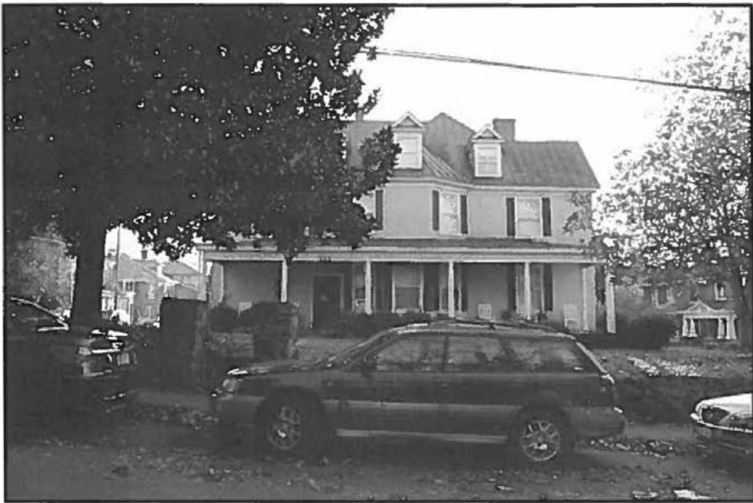
Photo 21. View of Turner-LaRowe House (VDHR #104-0234), Looking East.
