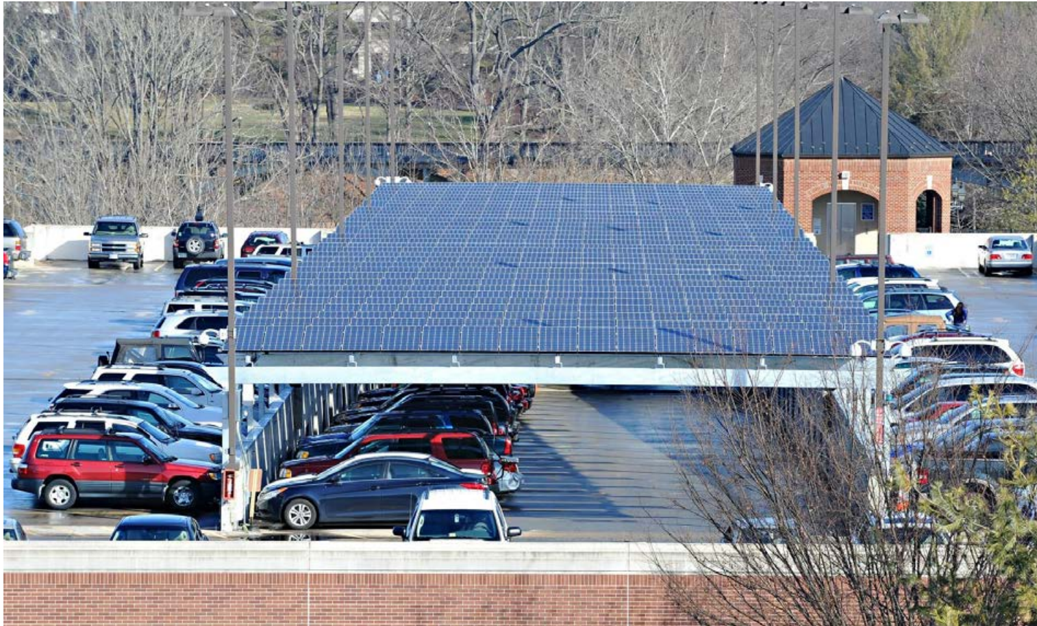
Parking Garage Canopies
