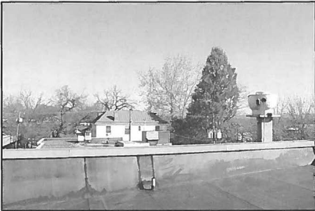
Figure 8. Views from Roof Level 1521 University Avenue Collocation Site (UVA MC N010), Charlottesville, Virginia, Looking North.
