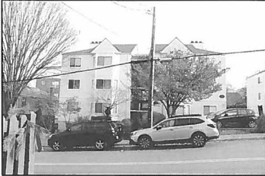
Photo 27. View of Modern Apartment Building, Former Location of McConnell-Neve House (VDHR #104-0397), Looking Southeast (Resource as Plotted in VCRIS Appears to have been Demolished).
