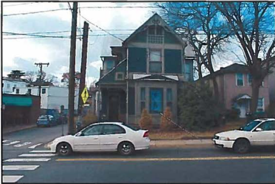
Photo 23. View of King-Runkle House (VDHR #104-0248), Looking West.
