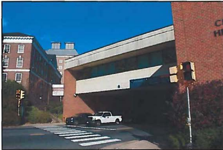
Photo 12. View to Proposed Small Cell Antenna Site from the Barringer Mansion (VDHR #104-0022), Looking Northeast (Not Visible).
