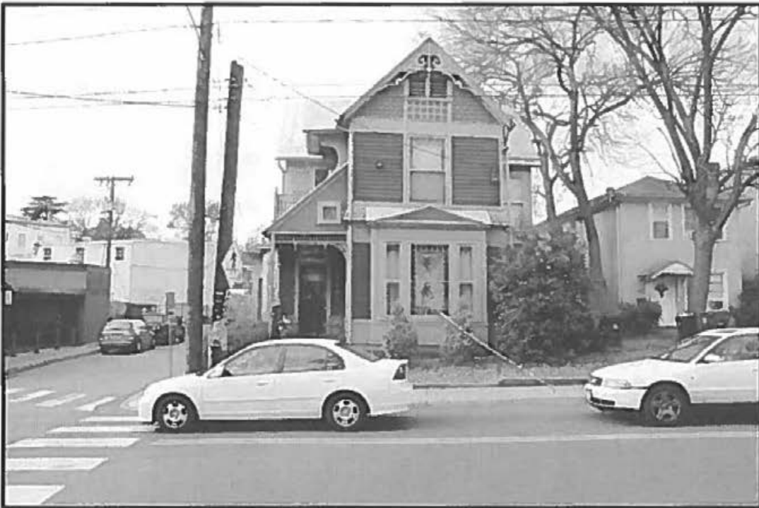
Photo 23. View of King-Runkle House (VDHR #104-0248), Looking West.
