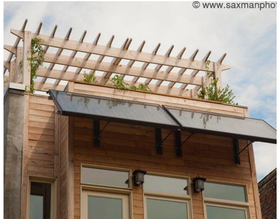
Building-integrated solar energy systems in residential districts
