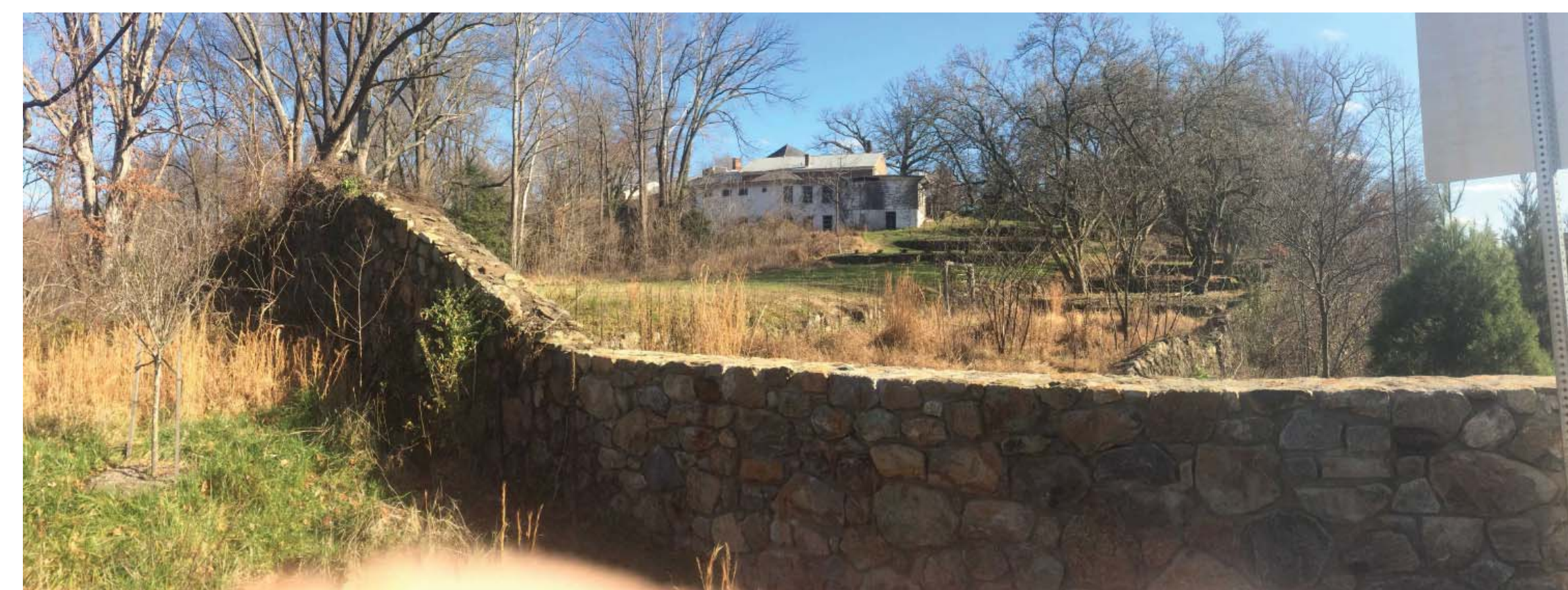
View from Rt. 250 at property line
