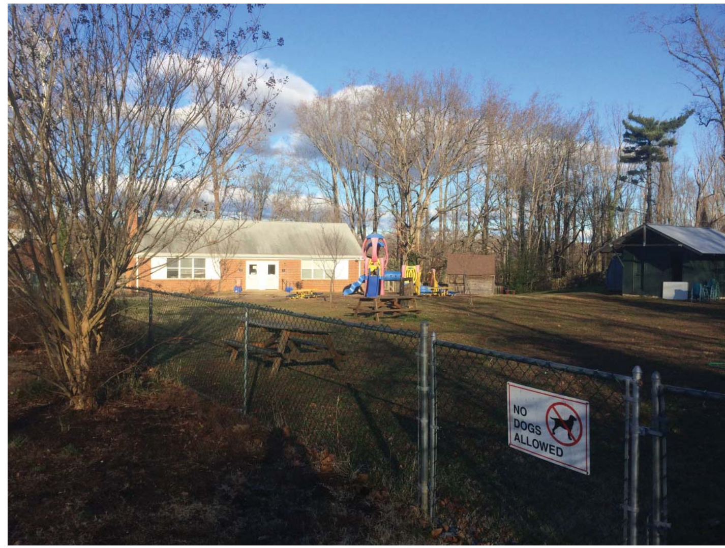
View of existing classroom and playground
