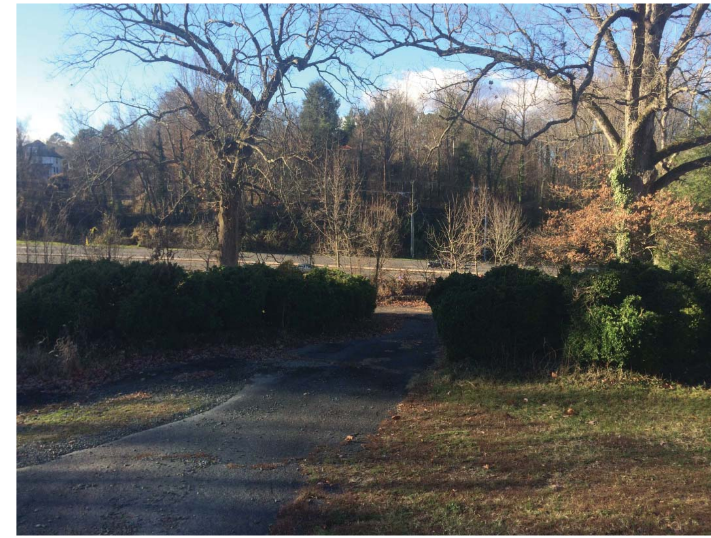
Abandoned entrance at Rt. 250
