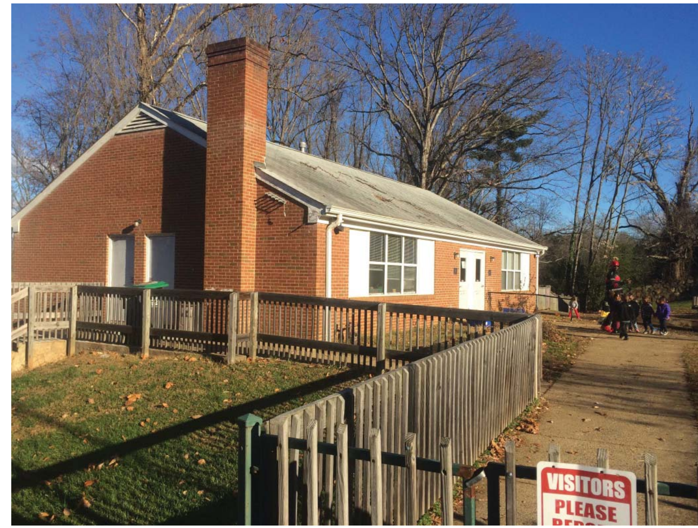
Existing classroom building
