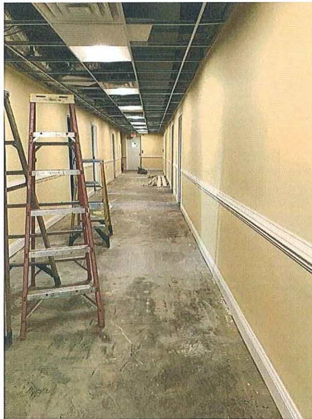
New floors are going in next!
