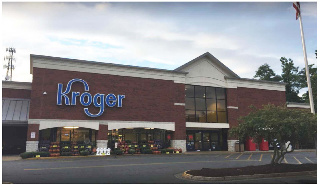
Kroger (South of Hydraulic Rd.)
