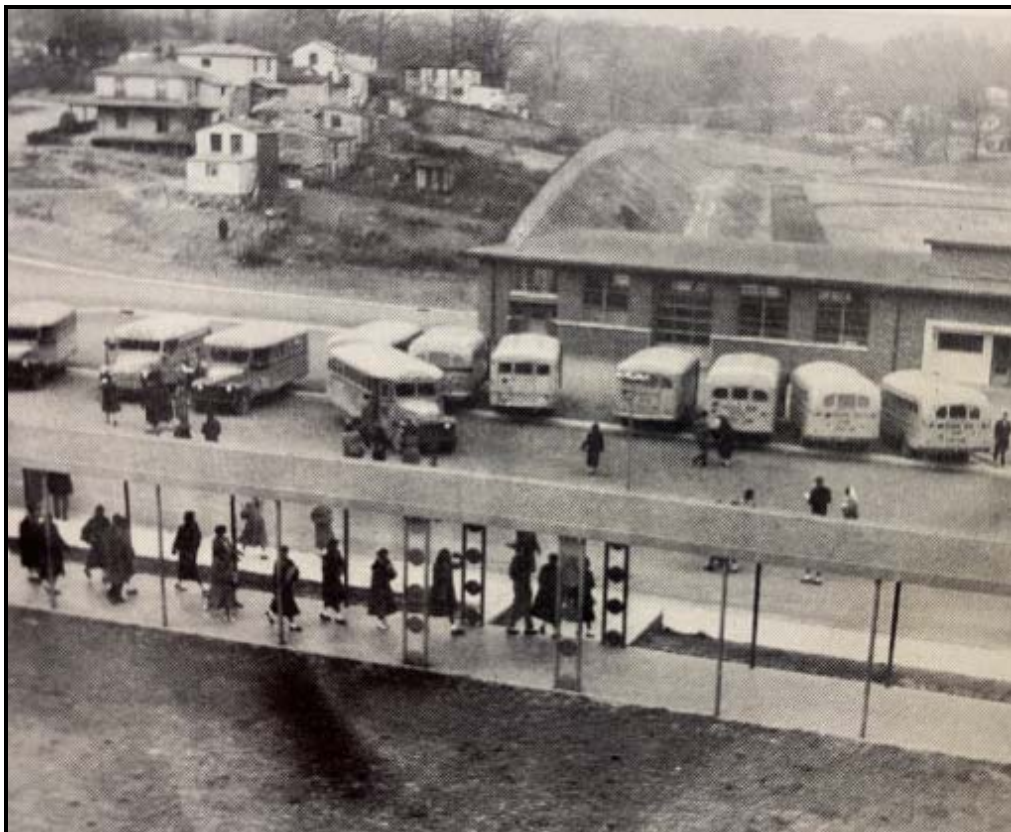
Figure 2: View from rear of school, looking west towards the covered walkway and detached manual arts building (1952).
