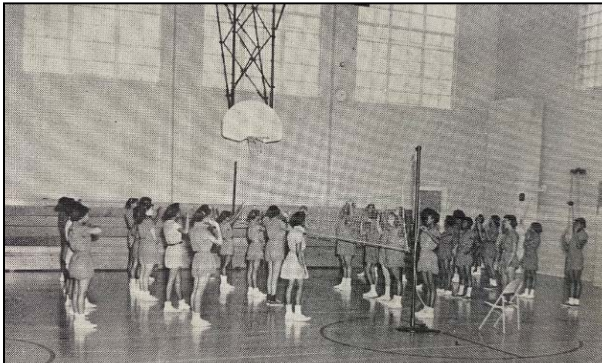
Fig. 8: view of gymnasium (1953) .
