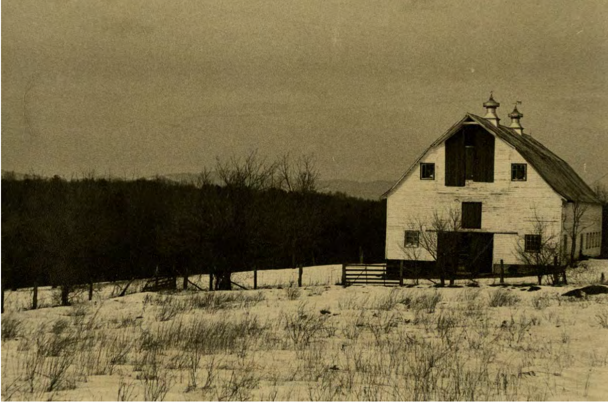
Historic Image 14. The dairy barn, built in 1937-1938. Date unknown. (Special Collections, University of Virginia Library)
