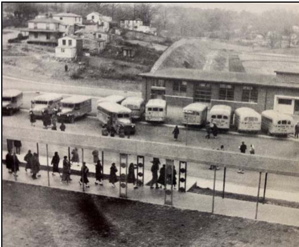
Figure 2: View from rear of school, looking west towards the covered walkway and detached manual arts building (1952).
