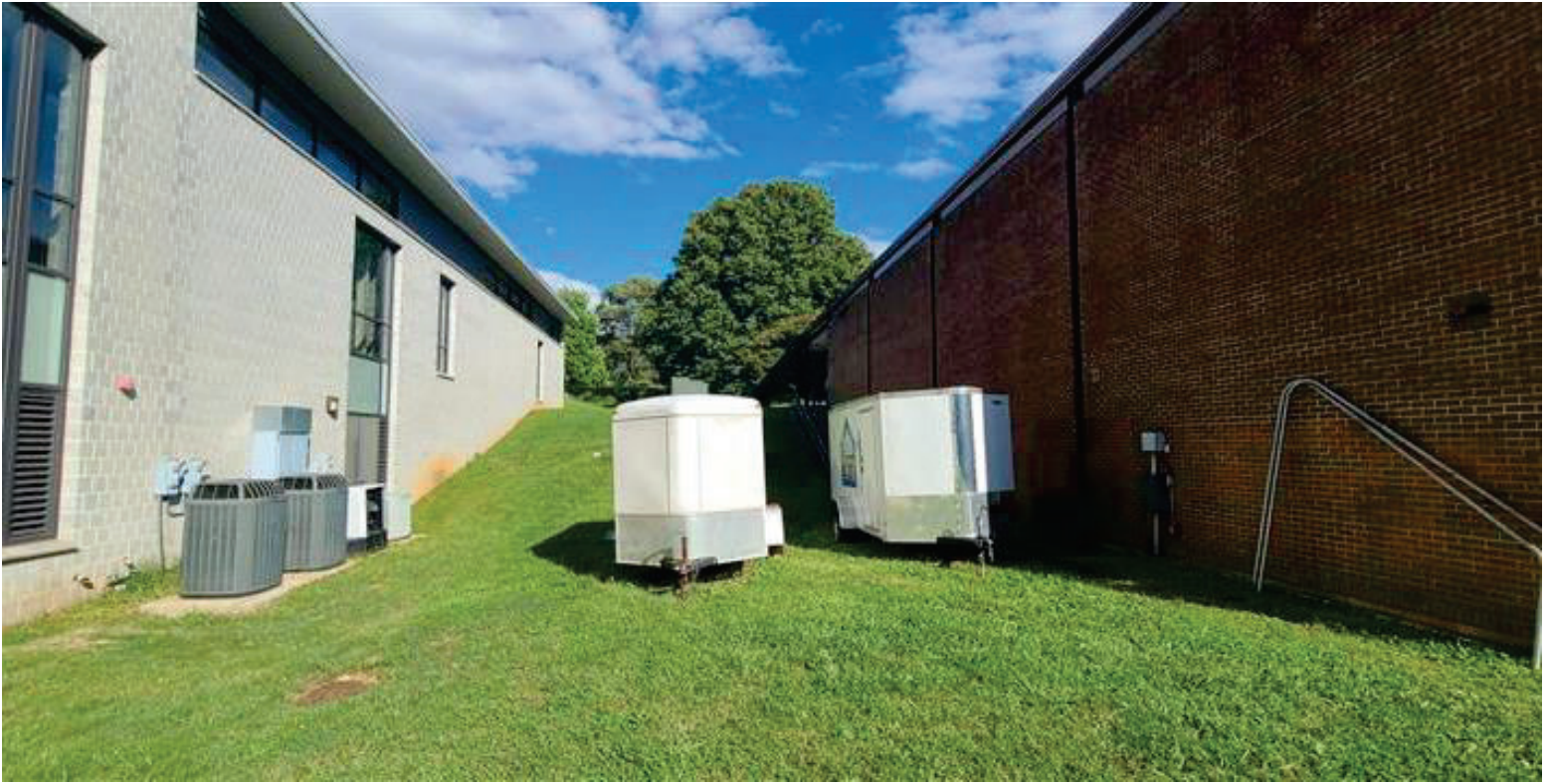
Buford Site – Existing underutilized outdoor space
