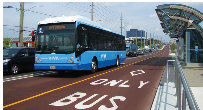
An example of dedicated transit lanes in suburban Toronto, Canada.
