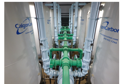
Granular Activated Carbon (GAC) treatment providing superior quality water to our community.
