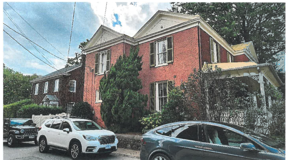
Facing Properties from E. High St./1 st St. N. Intersection
