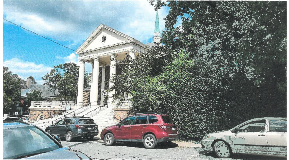
Property from E. Jefferson St./2 nd St. N.E. Intersection
