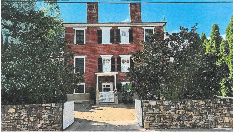
Neighboring Property from 2 nd Street N.E.
