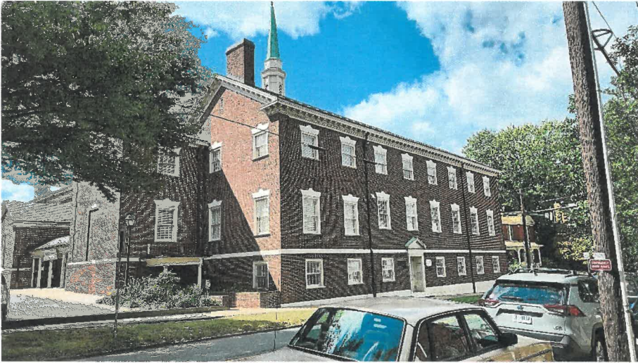
Property from E. High St./2 nd St. N.E. Intersection
