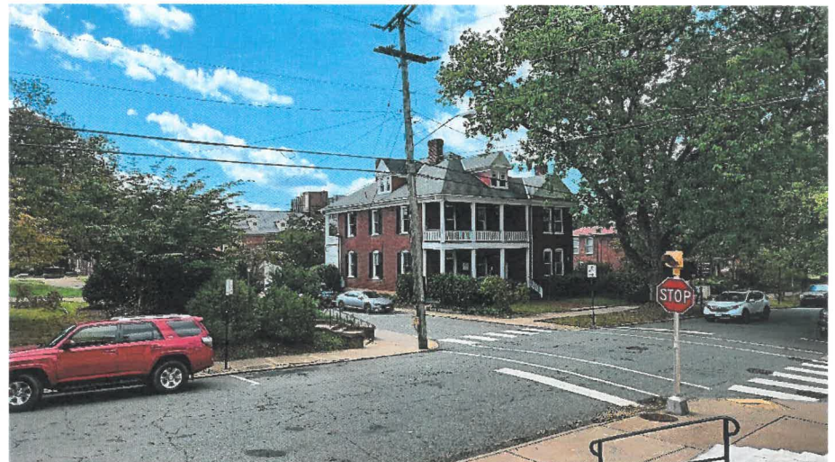
Facing Property from E. Jefferson St.
