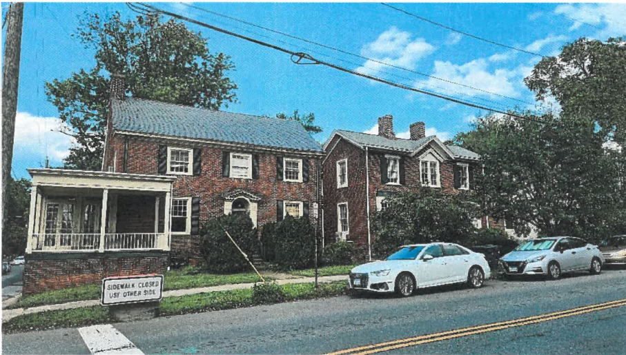
Facing Properties from E. High St./1 st St. N. Intersection
