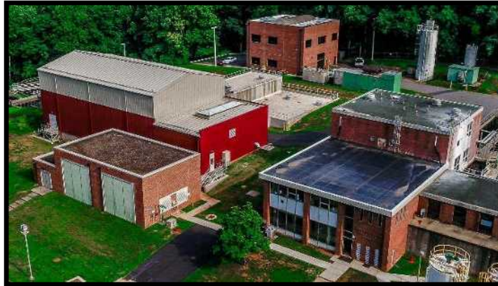
South Rivanna WTP 12 MGD
