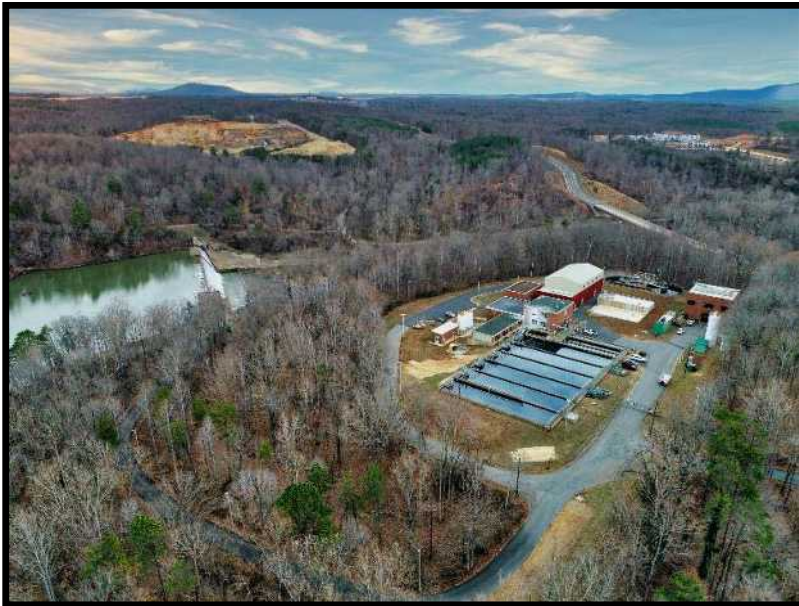
South Rivanna WTP
