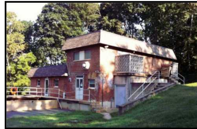
North Rivanna WTP 2 MGD
