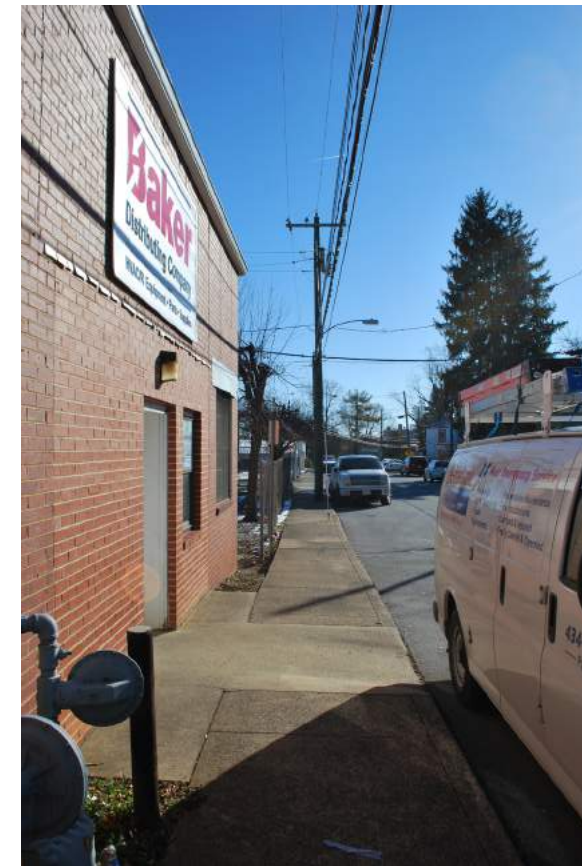
18. EXISTING REAR WING OF DAIRY
