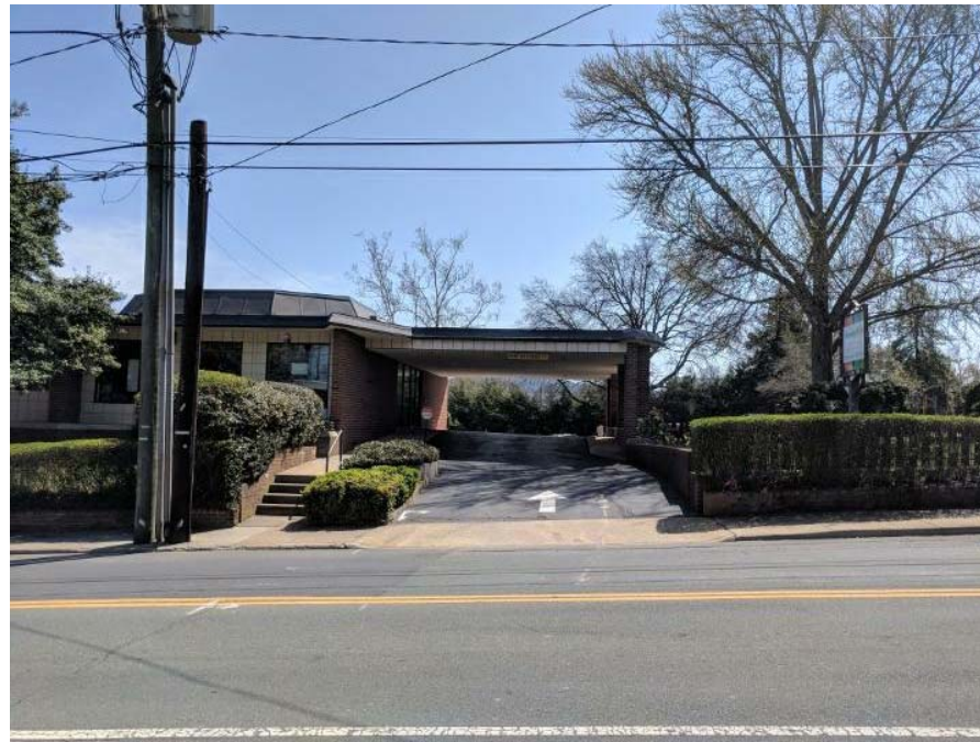
EXISTING PORT COCHERE
