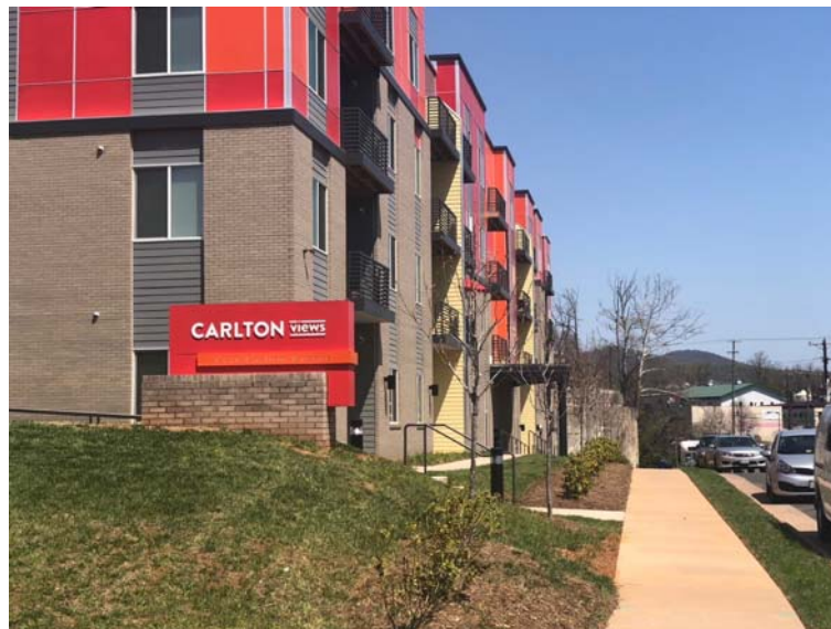
Existing Carlton Views Apartment Building CARLTON VIEWS PUD APPLICATION
