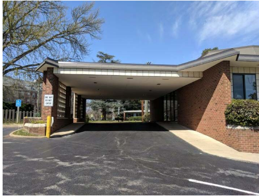
EXISTING PORT COCHERE TO BE REMOVED
