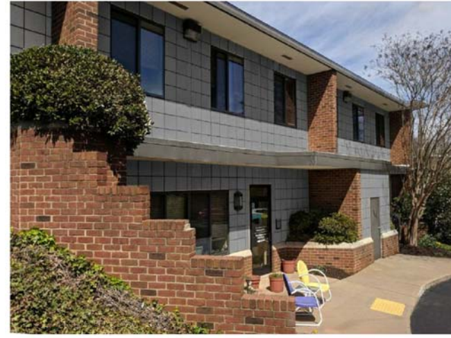
FACADE - AFTER, WITH NEW PAINT
