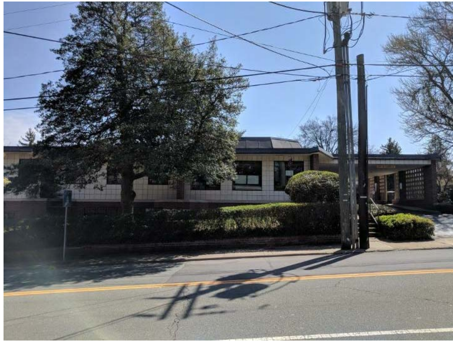
NORTH FACADE TO BE PAINTED
