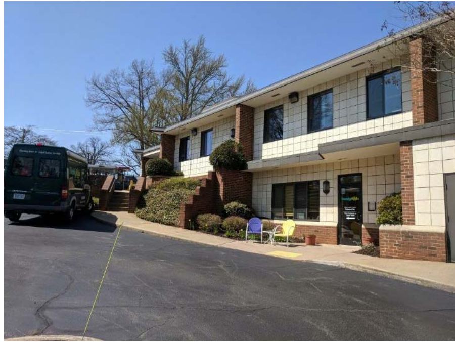
SOUTH FACADE TO BE PAINTED
