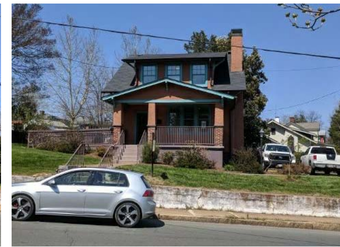
SHELTER 1100 E HIGH ST.
