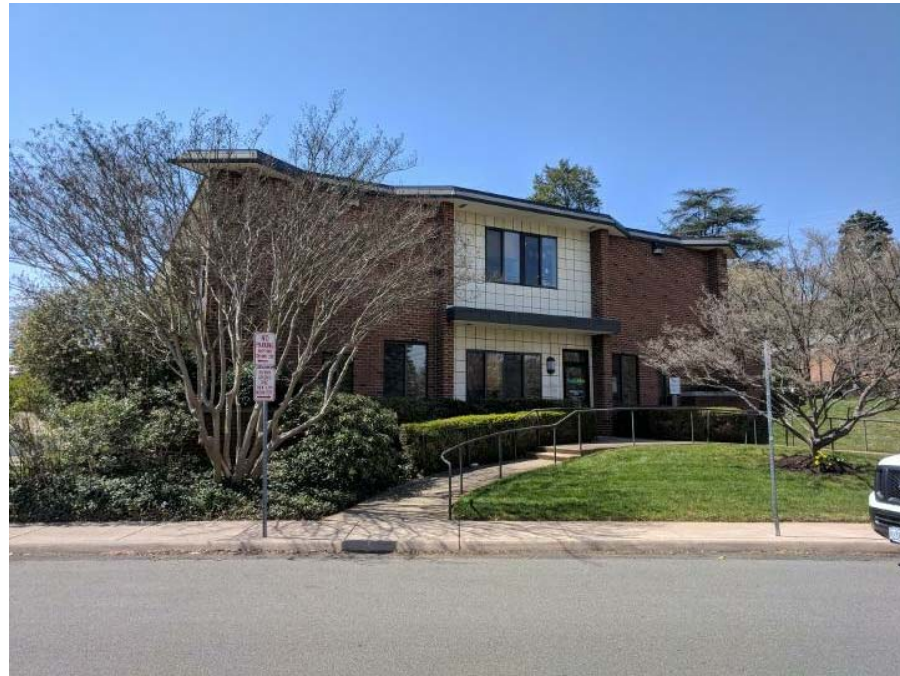
EAST FACADE TO BE REPLACED
