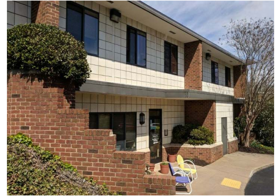
SOUTH FACADE TO BE PAINTED
