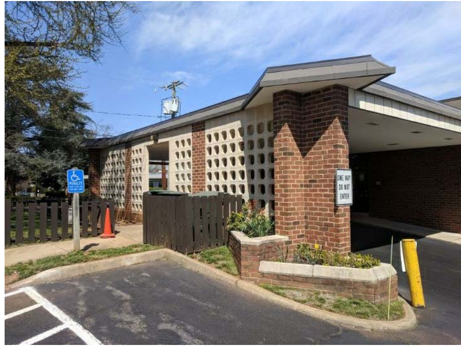
EXISTING PORT COCHERE TO BE REMOVED
