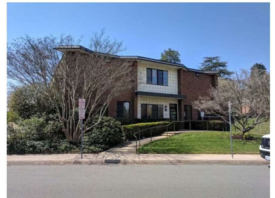
EAST FACADE TO BE REPLACED
