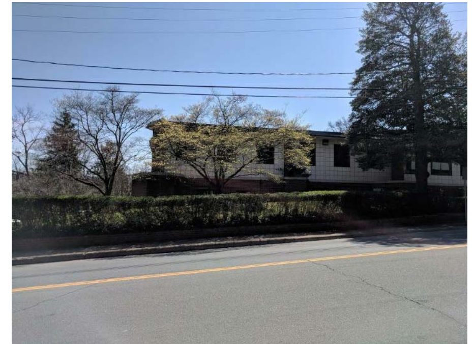
NORTH FACADE TO BE PAINTED
