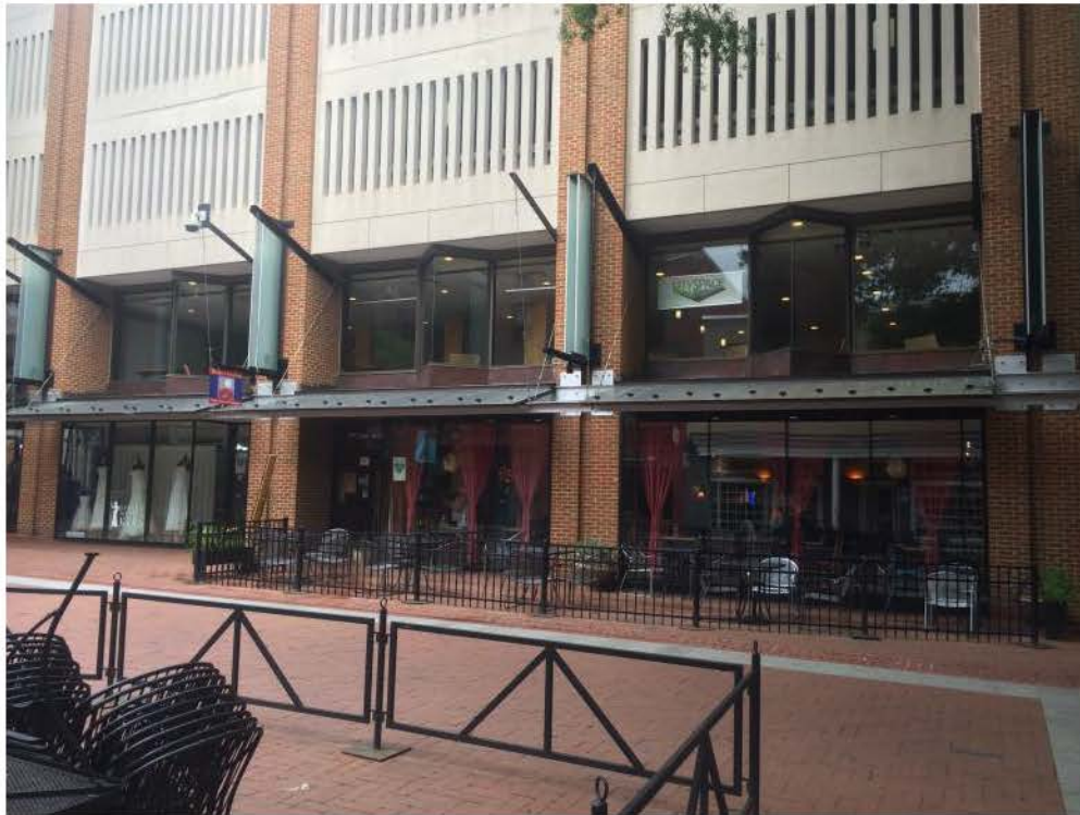
Downtown Mall, Market Street Parking Garage: Cable-supported awnings with standing seam metal
