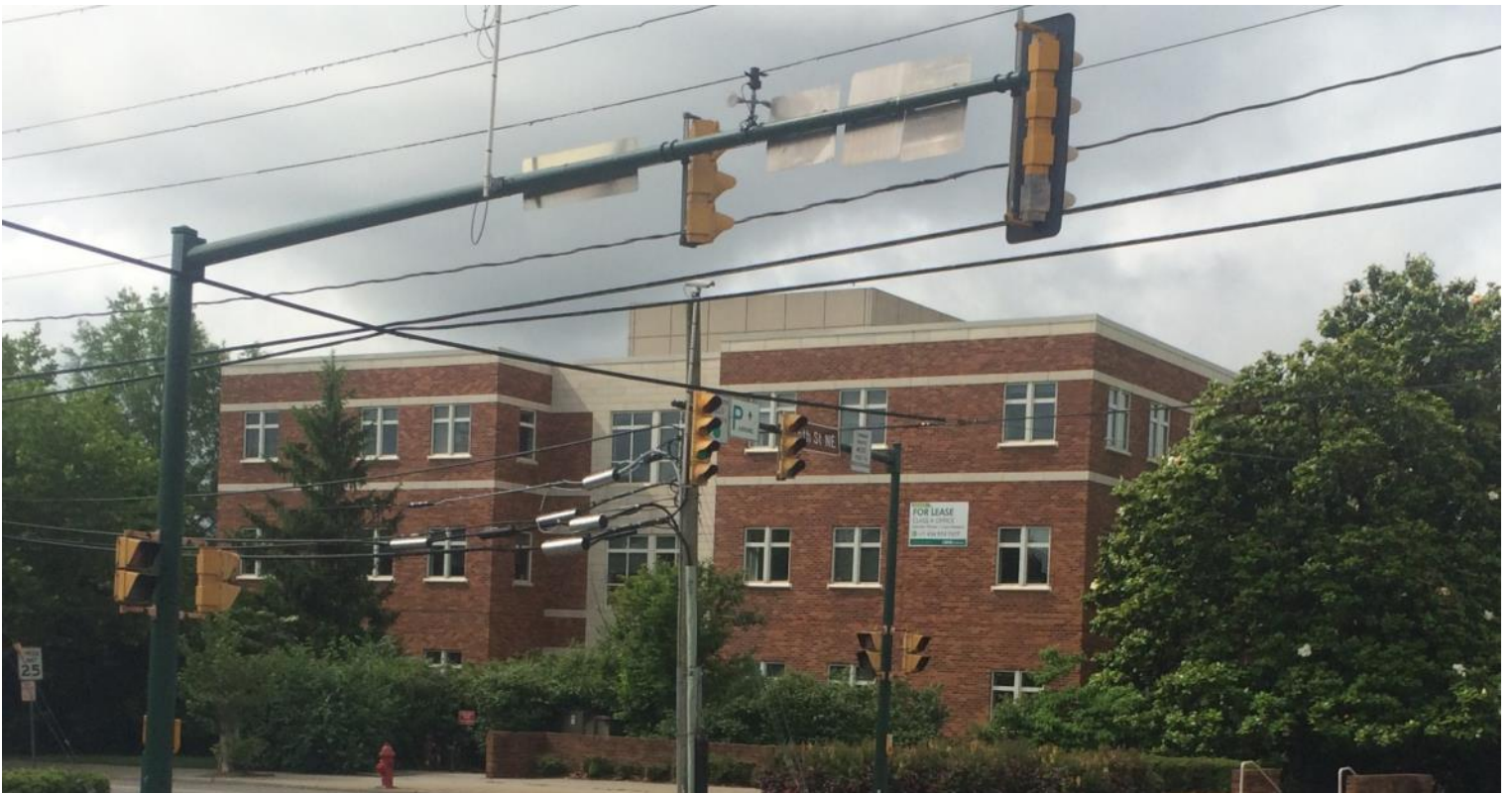
Precast accent bands with brick, punched windows - 701 East Water Street
