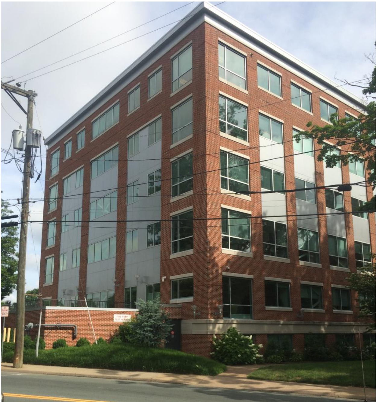
Metal spandrel panels, precast accent band CFA Institute, East High Street
