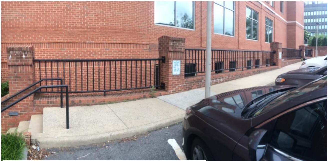
Railing with brick piers at City Hall Annex
