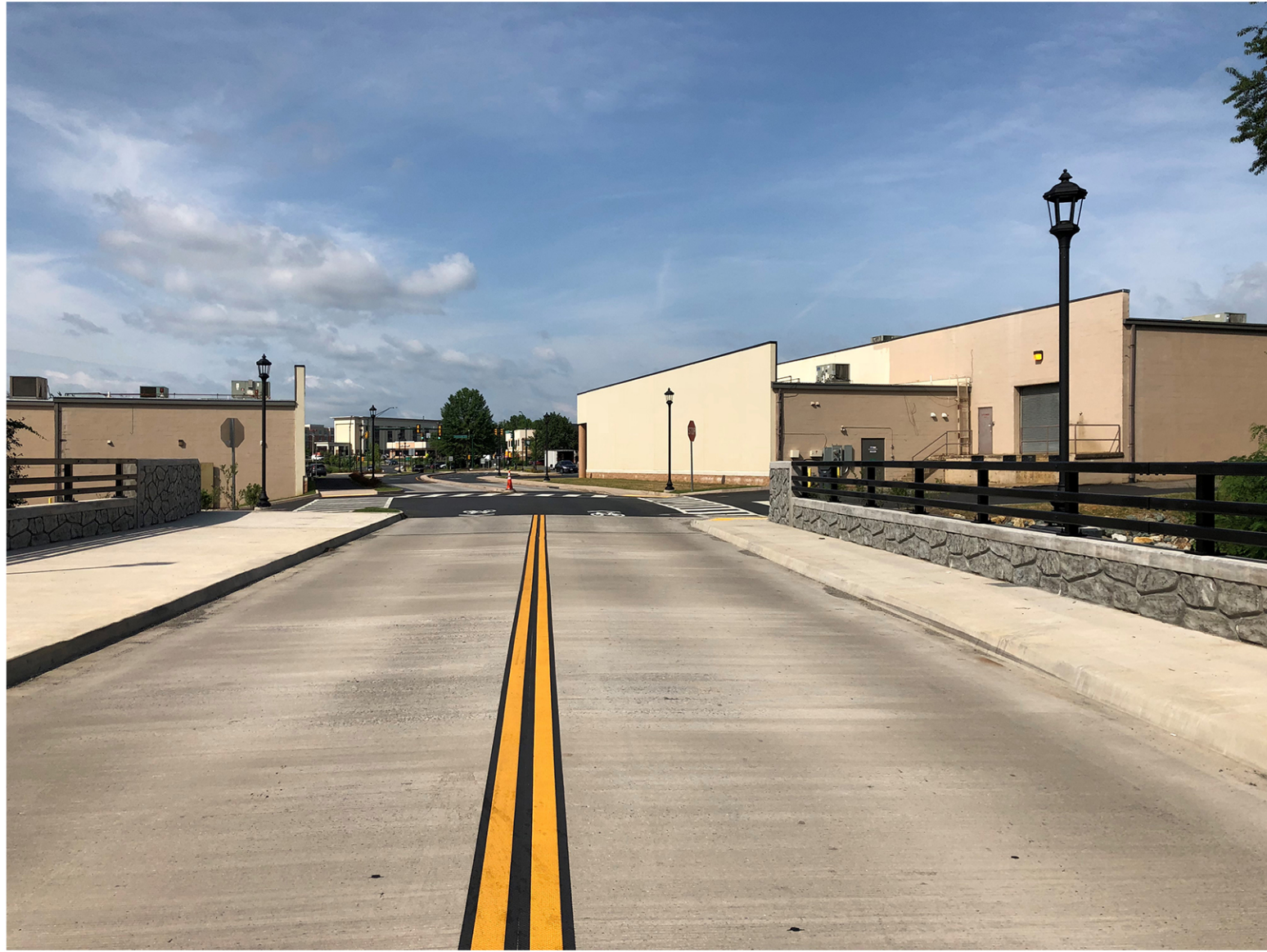
EXISTING TRAVELING SOUTH ON HILLSDALE DRIVE ON NEW BRIDGE LOOKING AT BACK OF NORTH WING
