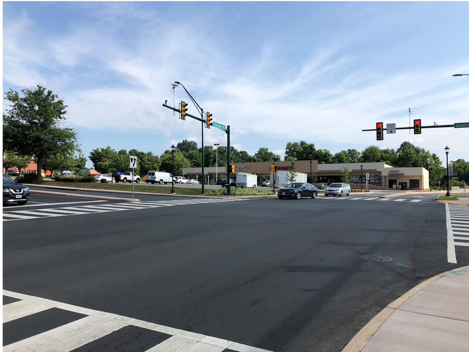
EXISTING INTERSECTION OF SEMINOLE COURT AND HILLSDALE DRIVE
