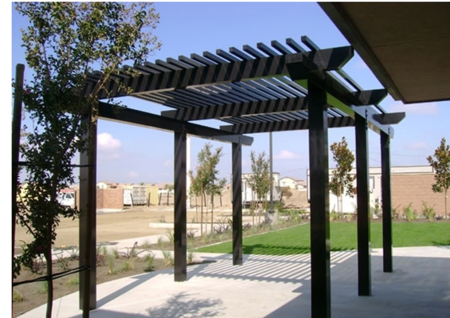
TRELLIS T009 B&C AWNINGS PAINTED BM 1617
