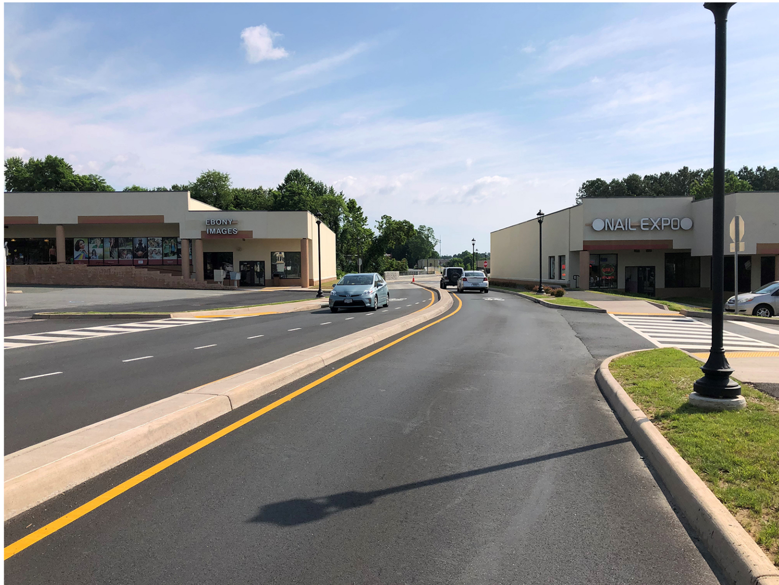
EXISTING TRAVELING NORTH ON HILLSDALE DRIVE
