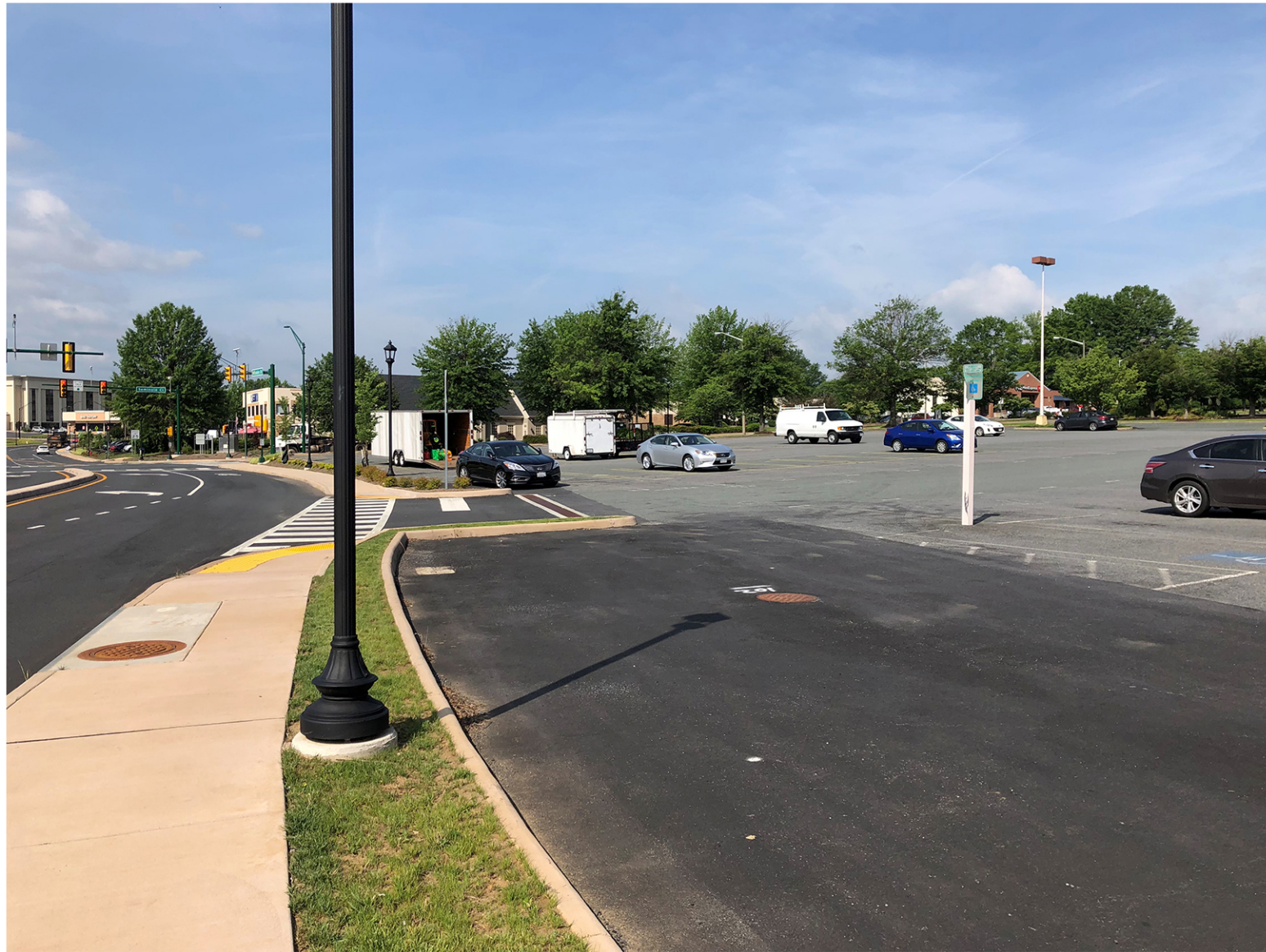
EXISTING NORTH WING PARKING LOT
