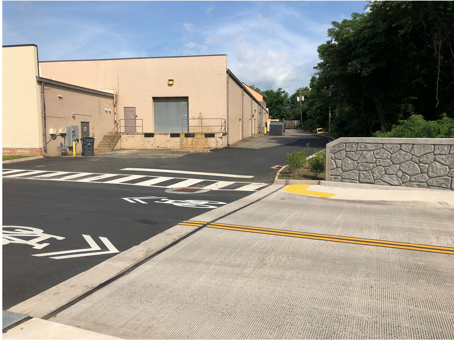
EXISTING AT END OF NEW HILLSDALE DRIVE BRIDGE LOOKING WEST AT REAR OF NORTH WING
