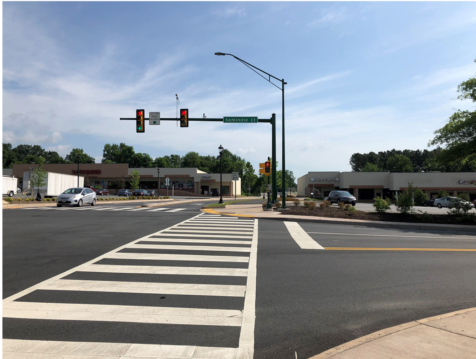
EXISTING SEMINOLE COURT LOOKING TOWARDS NORTH WING
