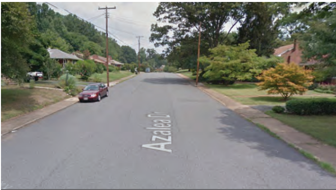
Azalea Drive south of Jefferson Park Avenue – 50’ with parking allowed on both sides and individual driveways; 4’-5’ sidewalks with obstructions both sides of the street.
