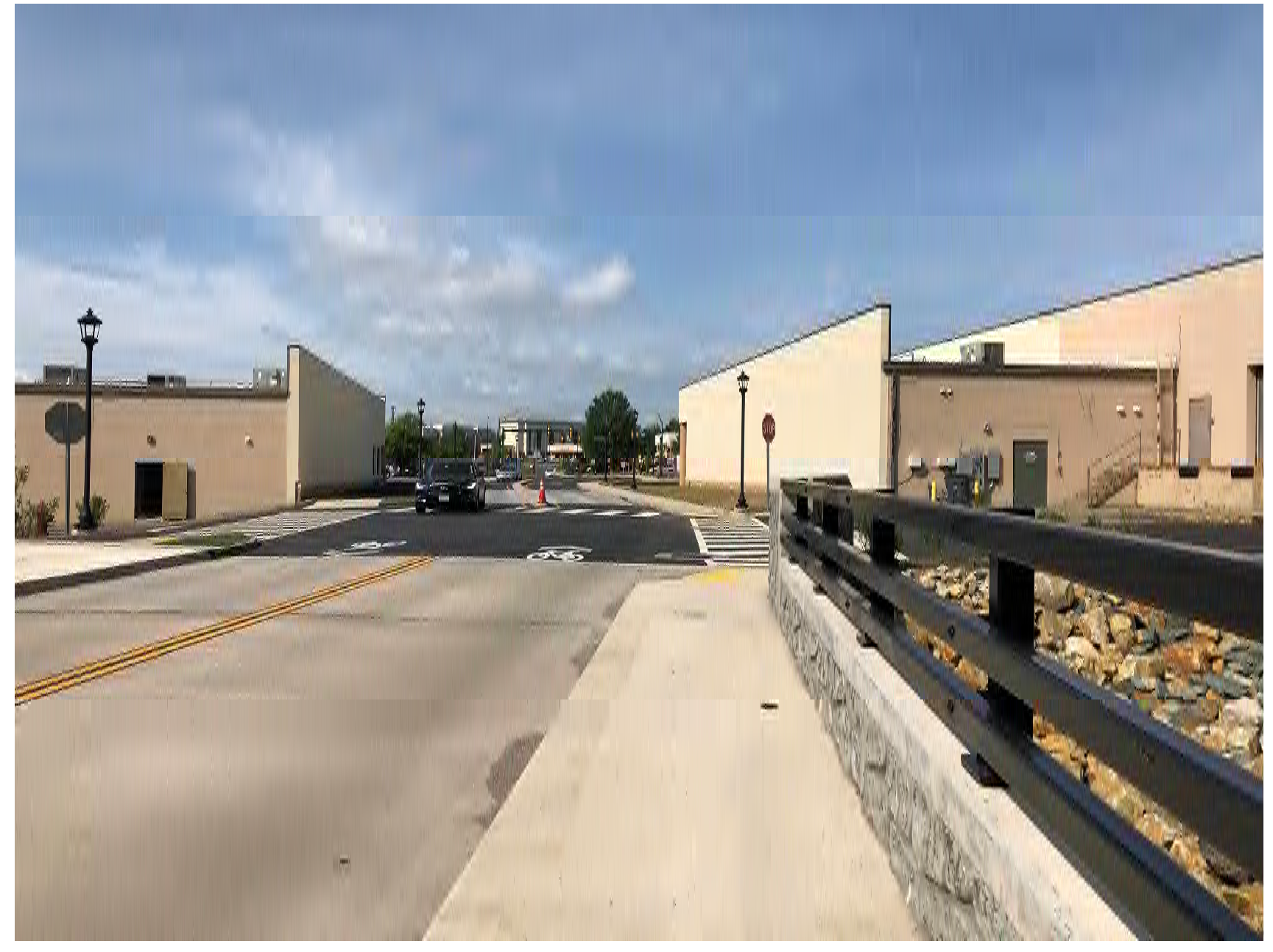
EXISTING CONDITIONS - NORTH WING REAR, HILLSDALE DRIVE
