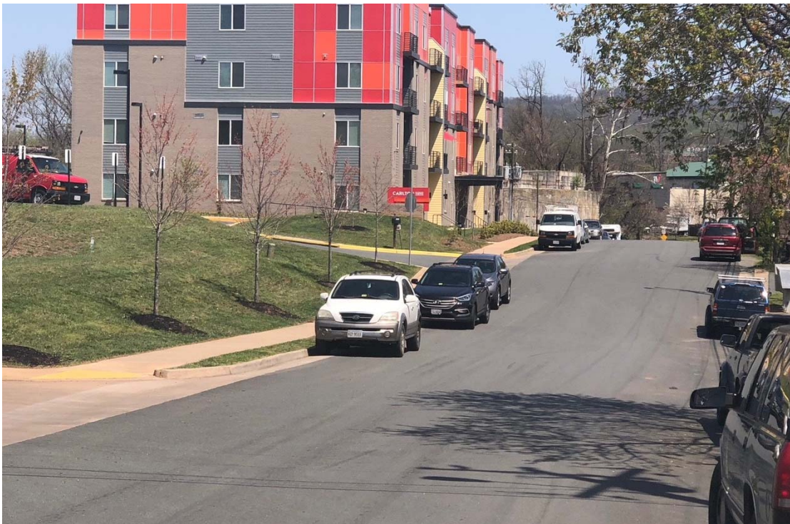
Picture of Carlton Avenue Improvements
