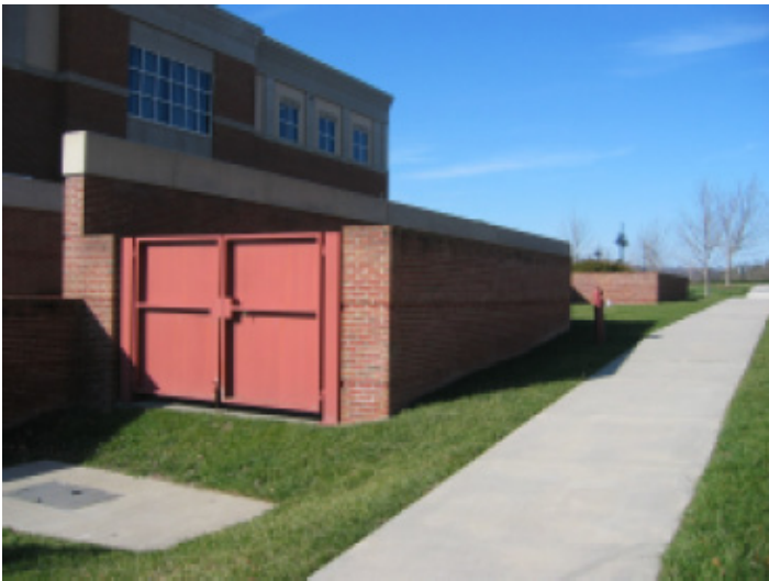
This enclosure coordinates well with surrounding buildings while screening mechanical equipment from view of passing pedestrian and vehicular traffic.
