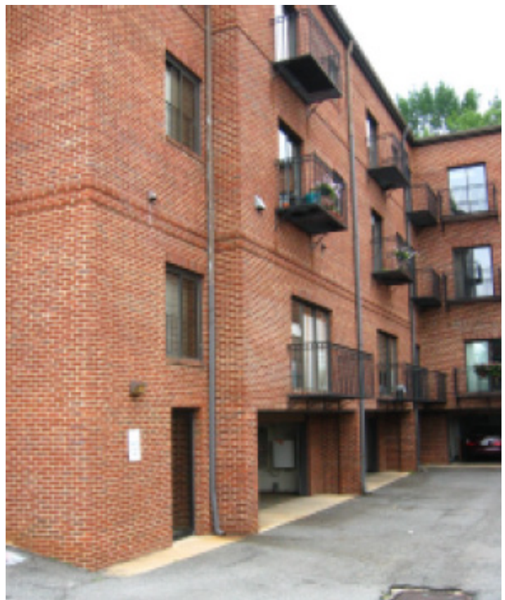
Ground level parking accessed from the rear of this mixed use building provides an ideal location for the placement of utility meters.
