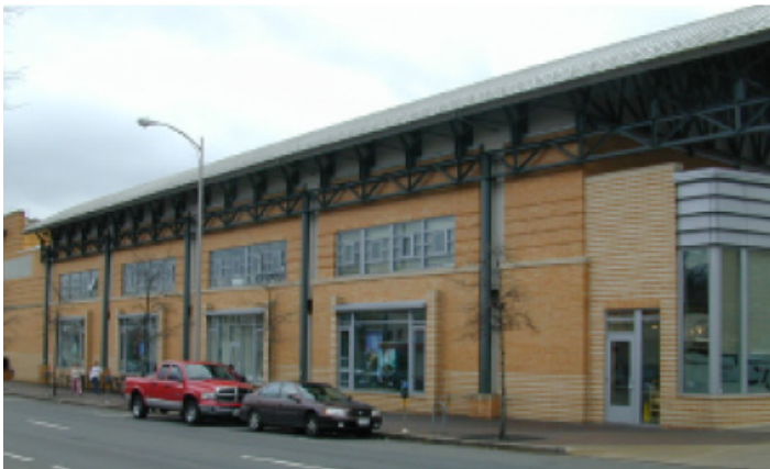
This grocery store uses large storefront display windows at street level, with smaller openings above, to break the facade into bays.
