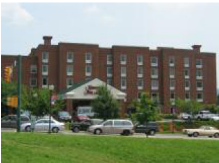
Cell towers are concealed within the chimneys of this hotel.
