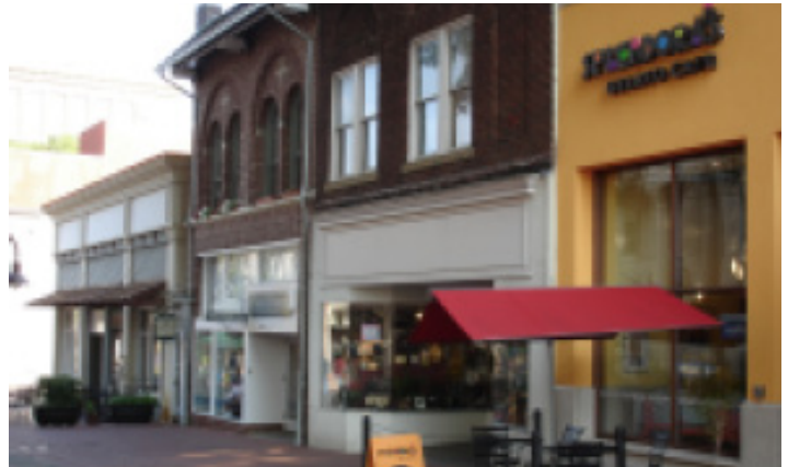
When renovating or designing a new storefront, consider using a traditional three-part facade of cornice, upper story windows and a storefront with an articulated base.
