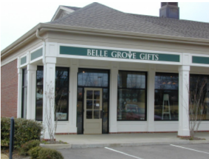
This storefront design is well detailed with transoms and an integrated sign band.
