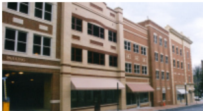
The design of this freestanding parking structure uses materials and forms to reflect the architectural character of the adjoining commercial area.
