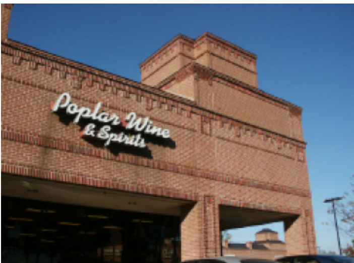
A stepped cornice tower, brick corbelling and string courses provide decorative details to this commercial structure.
