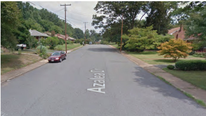
Azalea Drive south of Jefferson Park Avenue – 50’ with parking allowed on both sides and individual driveways; 4’-5’ sidewalks with obstructions both sides of the street.
