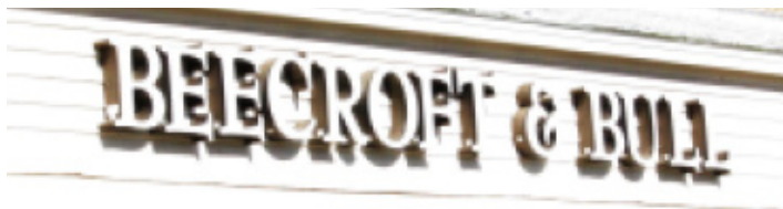
Channel set letters such as these at Barracks Road Shopping Center illuminate only the face of the letters and can be fabricated to match logos of individual stores as part of a unified sign plan.
