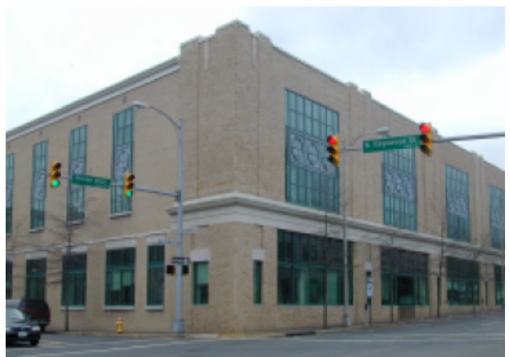
Vertical piers create bays and frame large expanses of glass divided into small panes accented with decorative insets. The storefront level is capped by a cast stone cornice.
