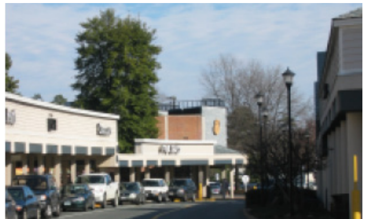
Parapet walls and railings shield rooftop equipment from view at Barracks Road Shopping Center.
