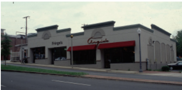
Remodeled facades on simple buildings have articulated cornices and colorful awnings on the storefronts.
