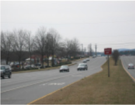
Sub-Area A: From the northern corporate limits to the 250 Bypass
