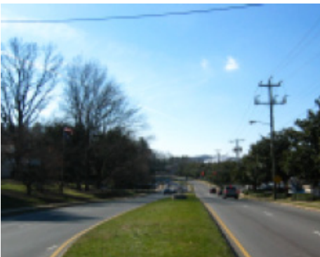
Sub-Area C: Barracks Road to Ivy Road
