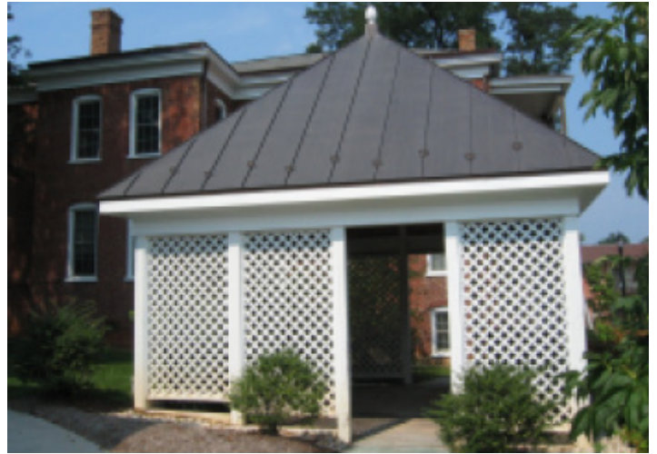
Plantings and lattice screen this service area for a multi-family residence from the adjacent structures and busy street.
