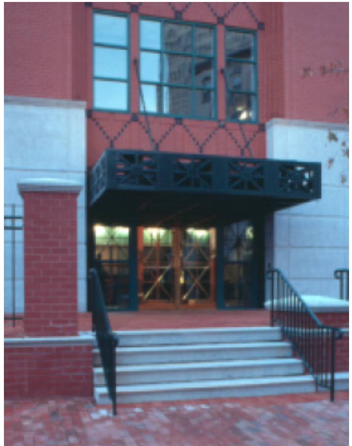
A decorative metal canopy and patterned brickwork help to emphasize the entry of this office building.
