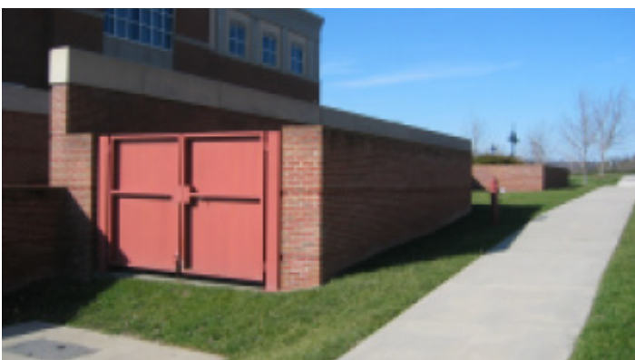
This brick wall, constructed of the same brick as the building, screens mechanical equipment from view.
