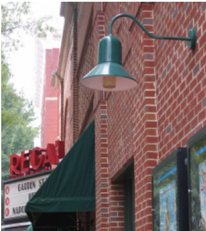
Attached to the building, this accent lighting is targeted downward and washes a portion of the facade as well as providing illumination to passing pedestrians. Additional accent lighting is located under the awnings.
