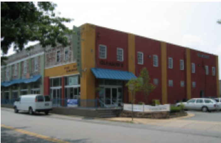
A strong palette of harmonious colors coupled with unpainted surfaces was used to differentiate between the feed store and former warehouse while tying the composition together with blue metal awnings.
